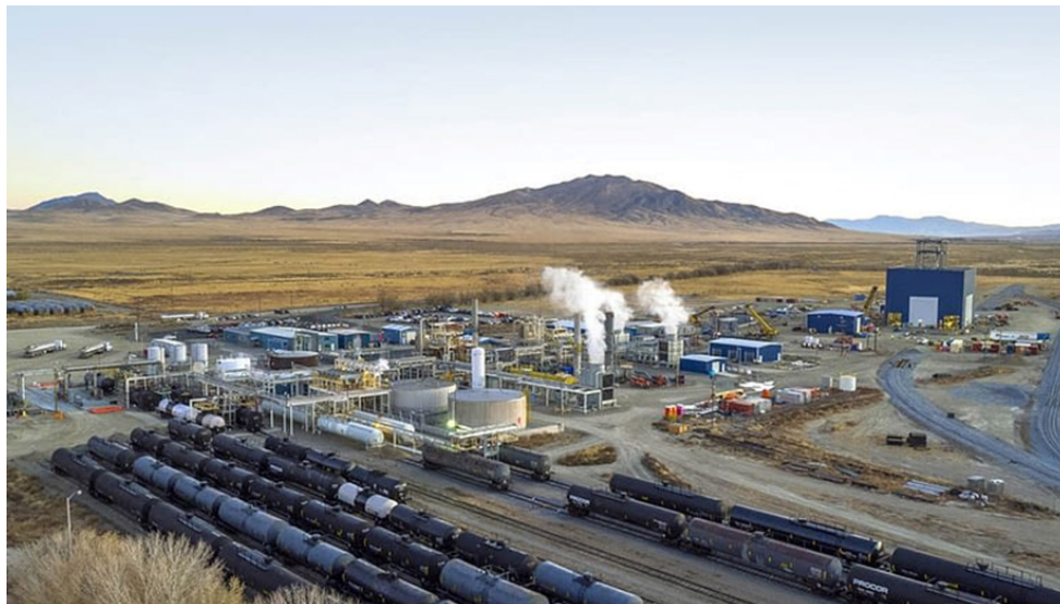
Figure 1. Cyanco Facility in Winnemucca, Nevada (Credit: Cyanco)
