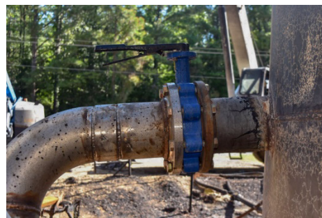
Figure 2. Open valve between new piping (left) and an old tank (right). (Credit: Red Hancock)
