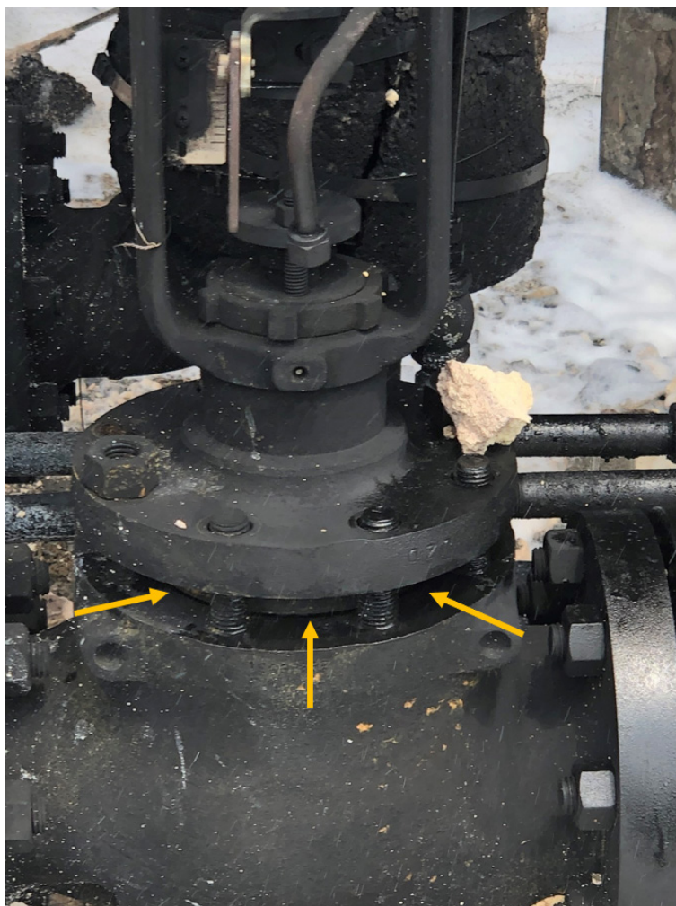
Figure 2. Naphtha release point (gold arrows). (Credit: CVR Energy with annotations by CSB)
