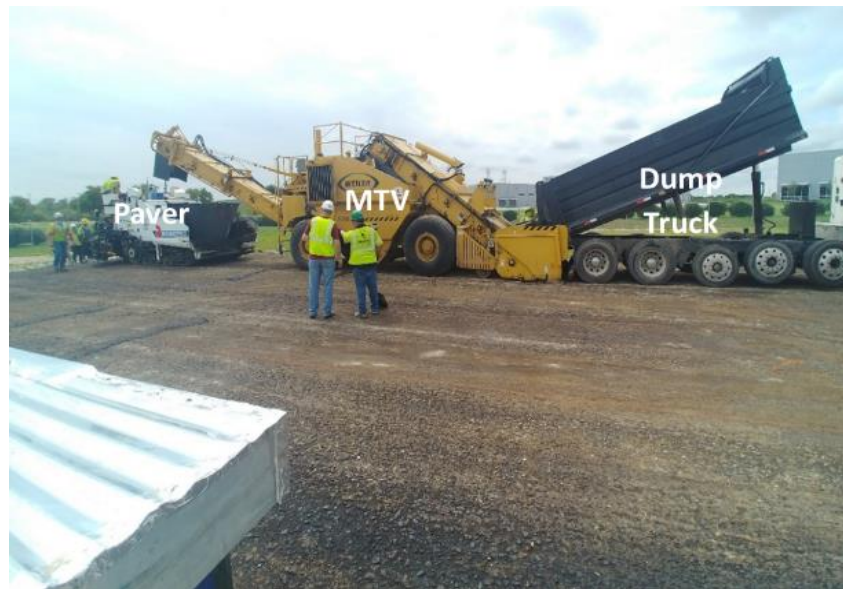
Figure 57. Paving Operation at Dallas Test Sections.
