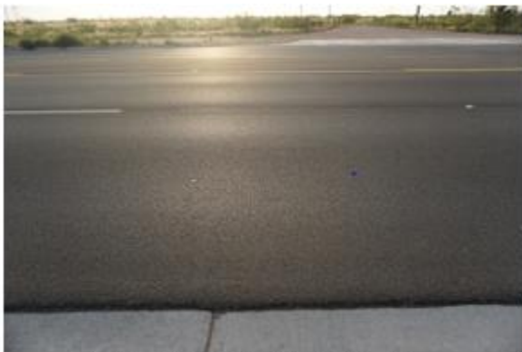
Rutting/Cracking/Pull-Up: None 03/07/2017
