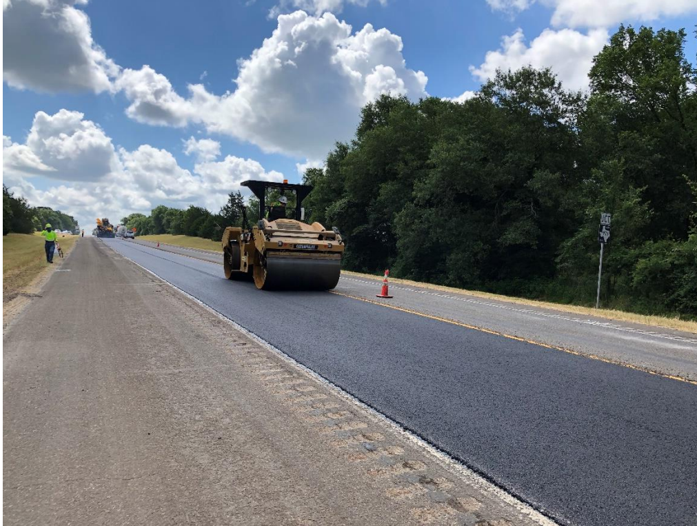
Figure 41. Compacting the Mat.
