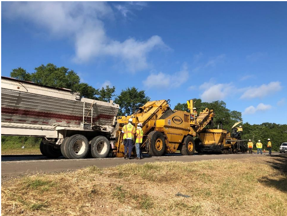
Figure 40. Paving Asphalt Mix.
