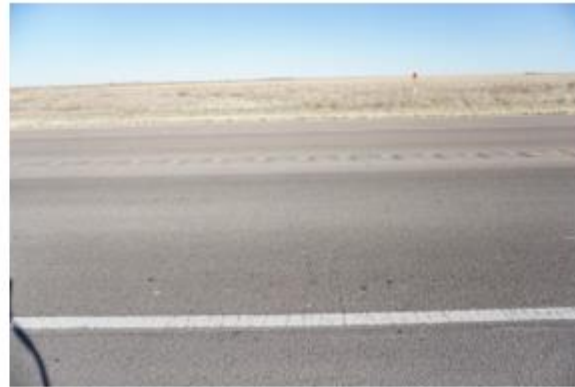
Transverse Cracking: 03/07/2017
