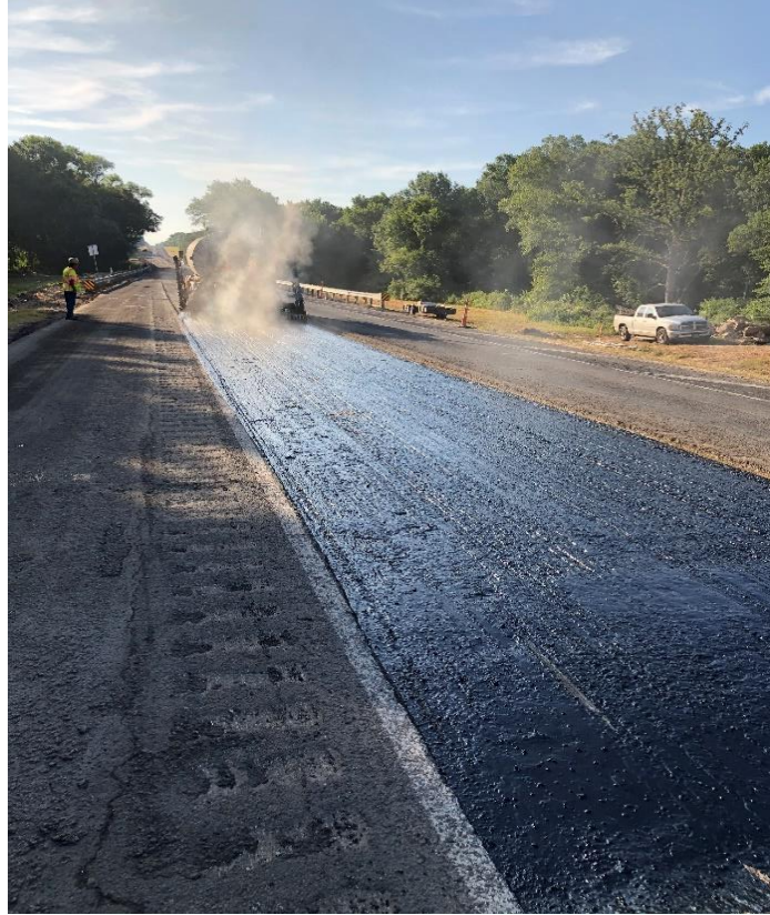
Figure 39. Applying Tact Coat.
