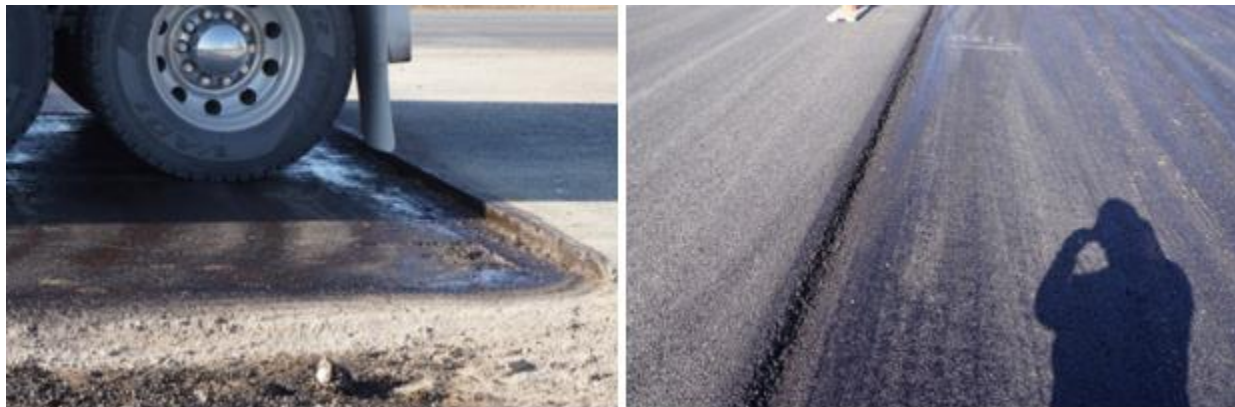
Figure 61. Applying Tack Coat on FM 2105.
