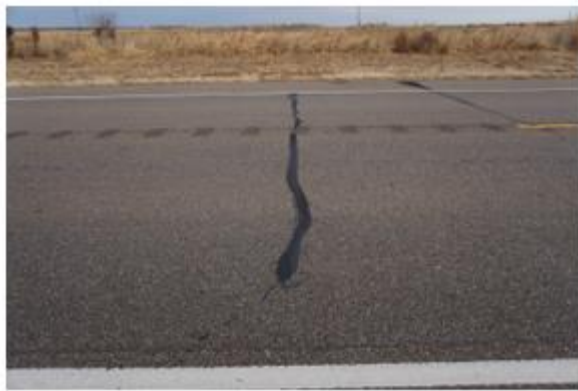
Transverse Cracking: 01/10/2018
