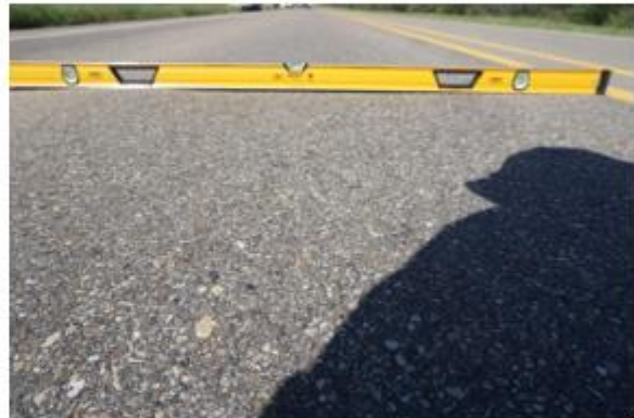
Rutting in Inner Wheel Path: 1/16–8/16 in. 10/09/2017
