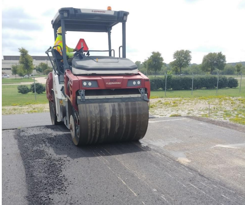
Figure 58. Compacting Test Sections at Dallas Test Sections.
