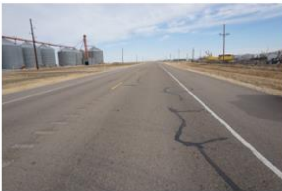
Overall Cracking: 01/10/2018
