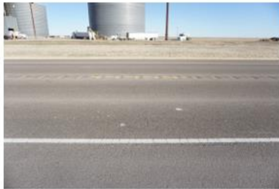
Transverse Cracking: 03/07/2017
