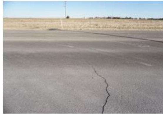
Transverse Cracking: 03/07/2017
