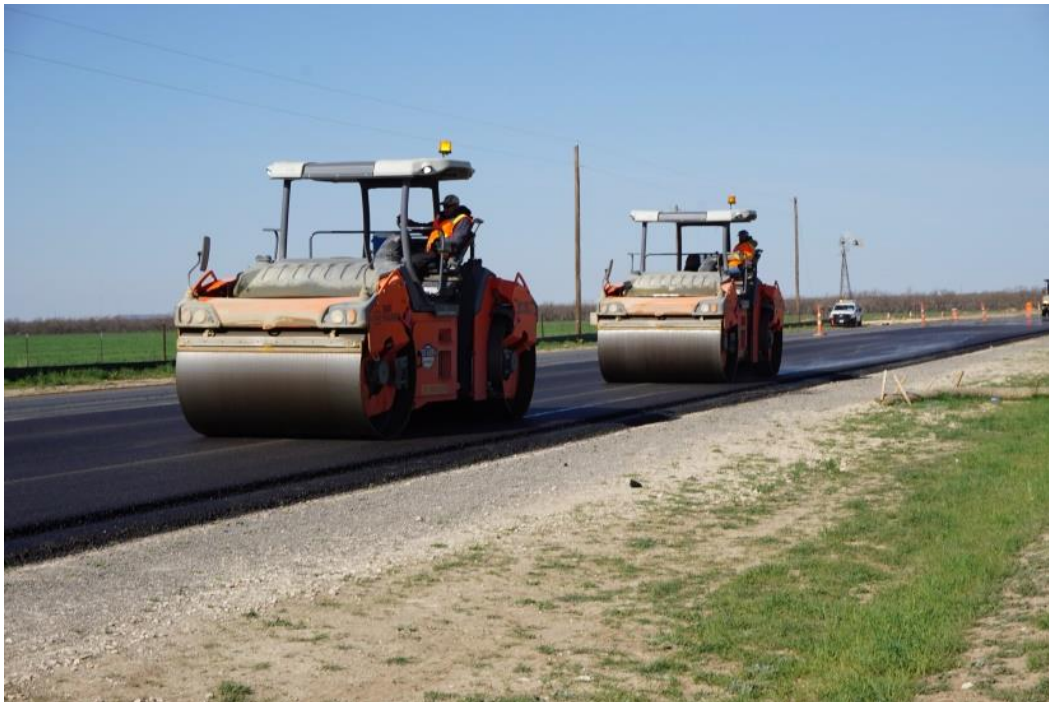
Figure 63. Compacting Test Sections on FM 2105.
