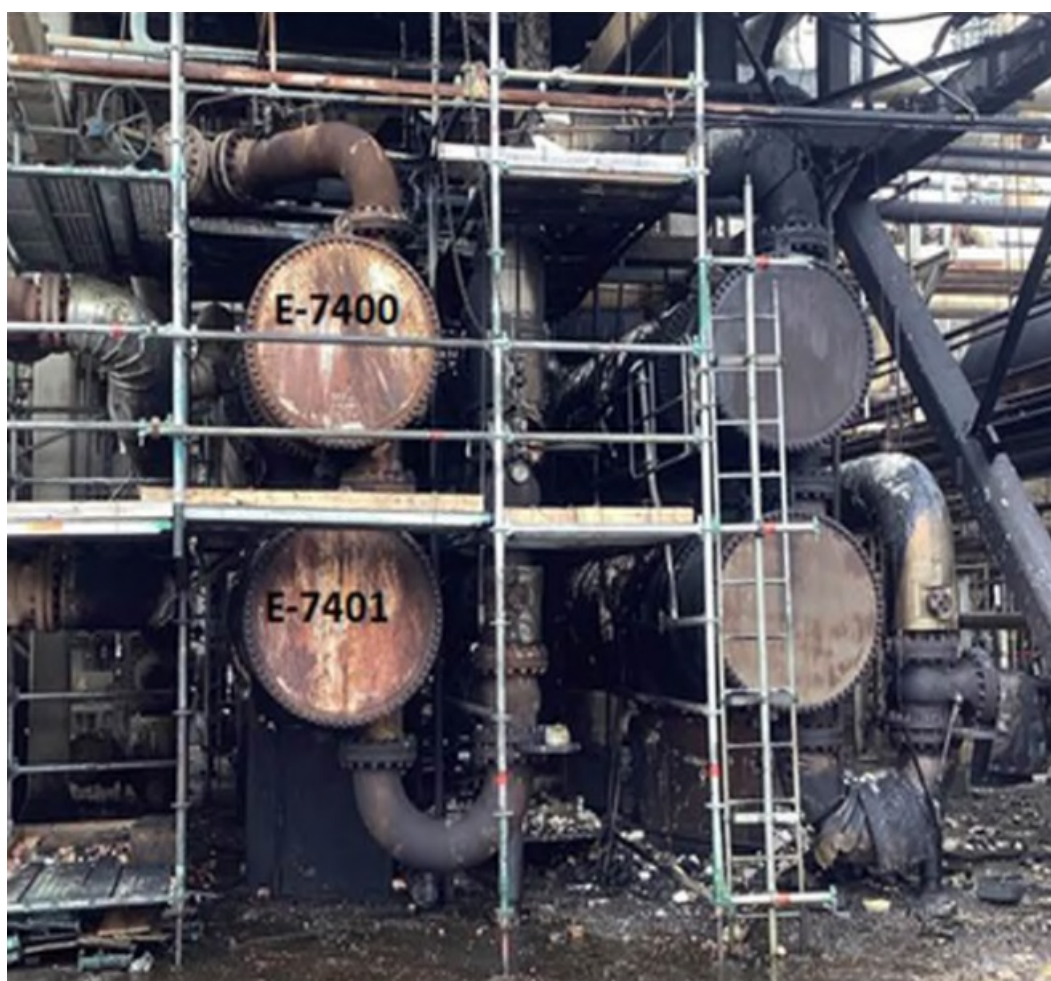
Figure 1. Heat exchangers after the incident. (Credit: Pemex)
