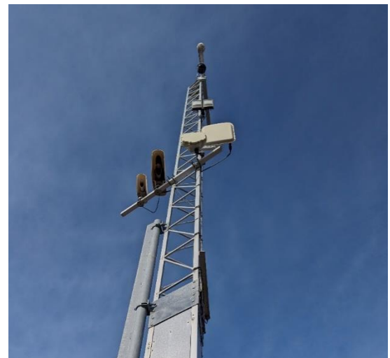
Figure 10: SDDOT Traffic Monitoring Equipment Installed on an ESS Tower
