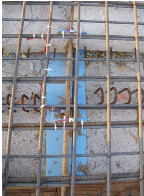
Figure 2.36. Construction of crack-forming wood detail, reprinted from Munsterman (2017).
