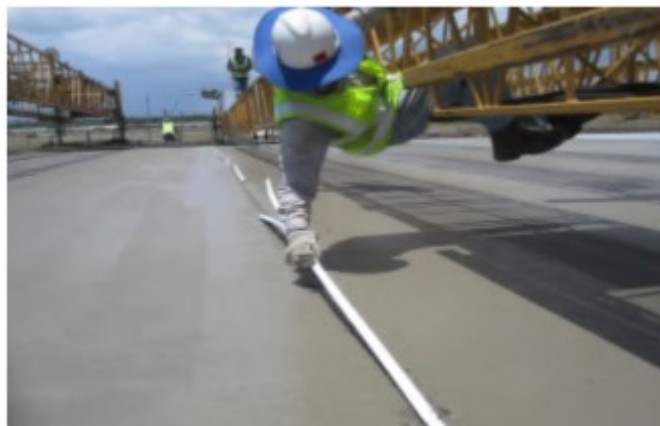
Figure 2.24. Installation of zip strip crack former, reprinted from Bayrak et al. (2013).
