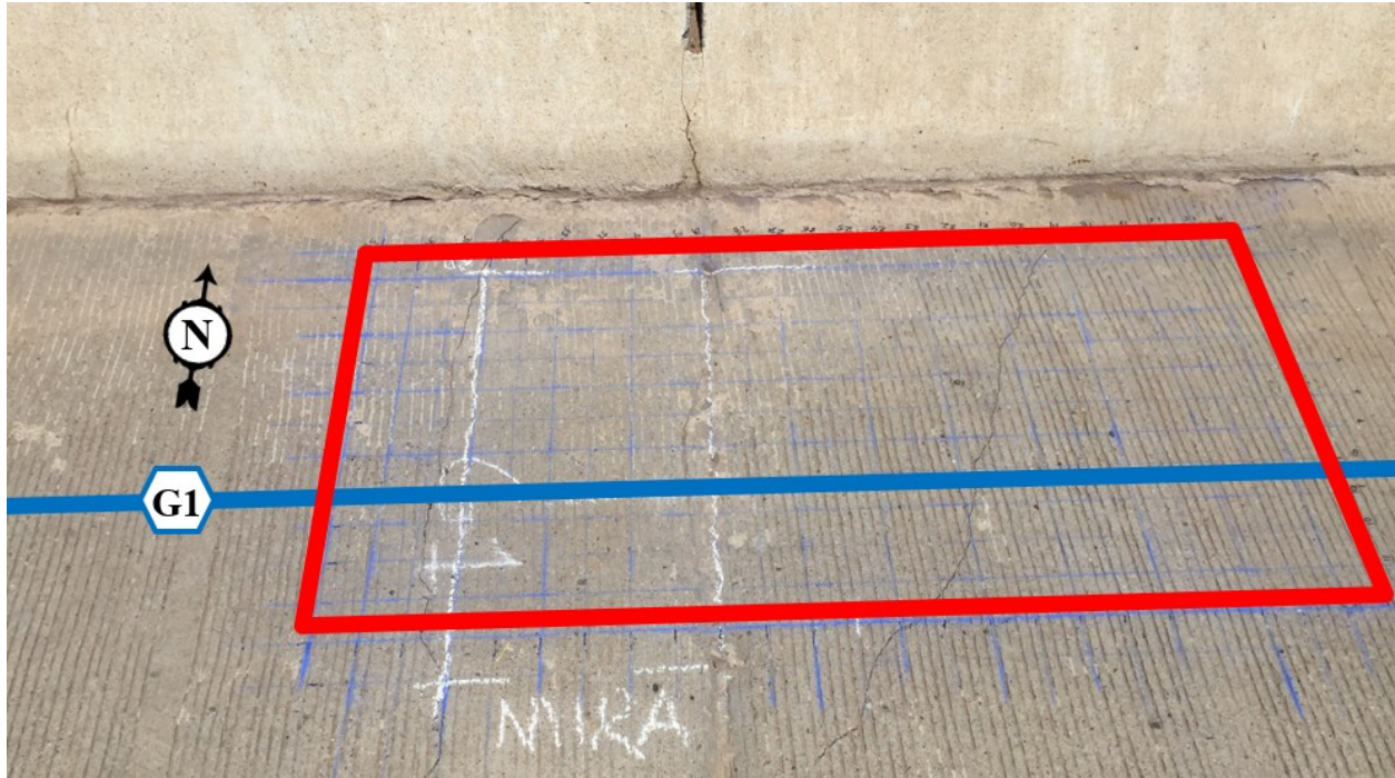
Figure 4.56. Secondary NDE region for GPR at Bent 3 in the overhang at Bridge LUB4 (WB Loop 289 over University Ave.).
