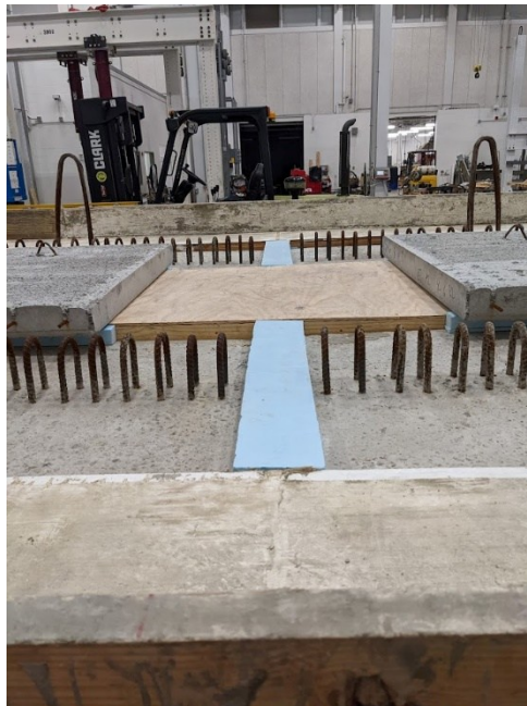
Figure 9.18. Formwork used between girder ends for offset panel tests (PBJ-OP1 shown); post-installed dowel bars not present.
