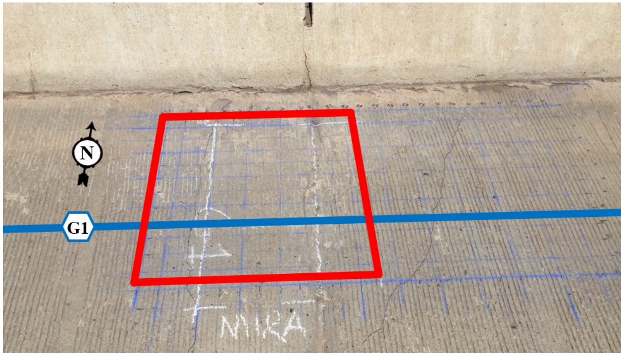
Figure 4.57. Secondary NDE region for UST at Bent 3 in the overhang at Bridge LUB4 (WB Loop 289 over University Ave.).
