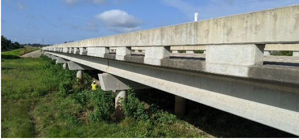
(a) Elevation view of bridge
