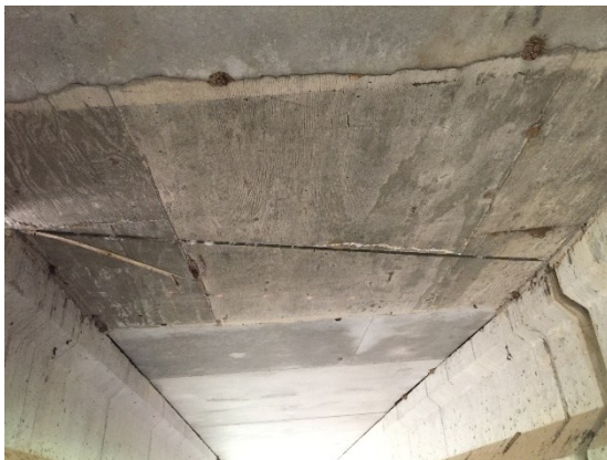
(a) CIP at continuous deck detail
