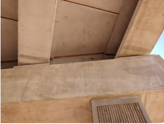
(a) Flush panels at continuous deck joint
