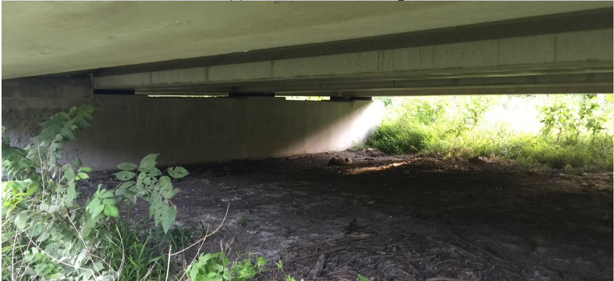
(b) View beneath bridge
