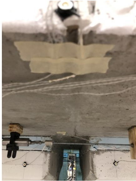
Figure 9.39. Surface strain measurements on bottom of deck using LVDTs.
