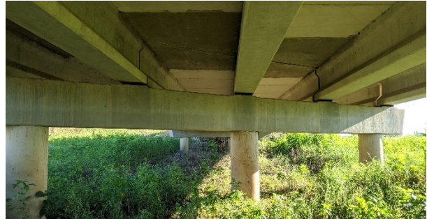
(b) View beneath bridge
