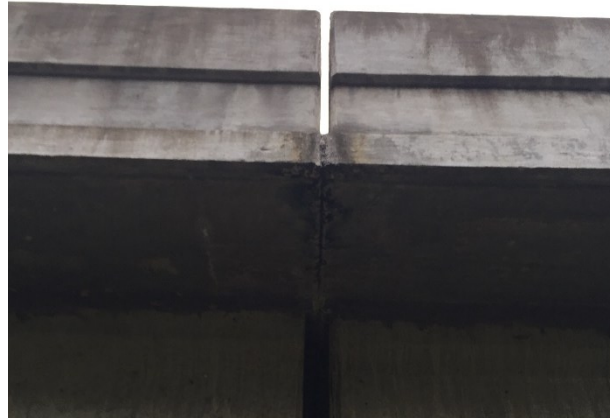
(b) Bottom of overhang at Bent 4
