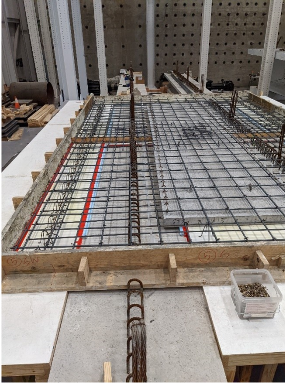
(a) Looking west
