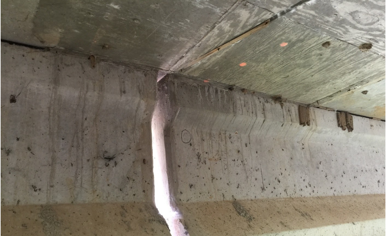
Figure 6.13. Atlanta District bridge without a foam insert or skewed girder end detail.
