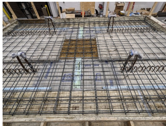
Figure 9.32. PBJ-OP2 formwork with all rebar (the north girder is at bottom and has supplemental top bars).
