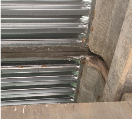
(a) PMDF at continuous deck
