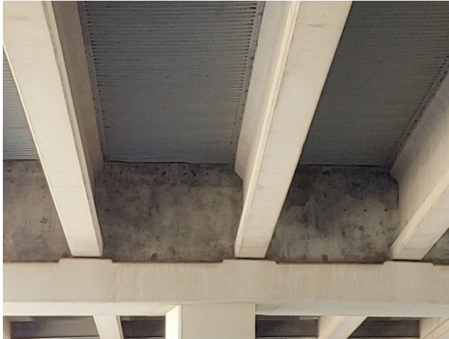
(a) Inverted-T bent cap and PMDF between girders
