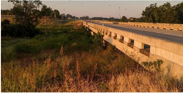
(a) Elevation view of bridge
