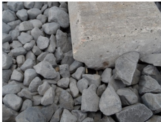
Figure 2 Concrete crosstie that experienced undercutting abrasion damage, including the exposure of some wires in a section of track in Washington State. (Picture courtesy of BNSF)
