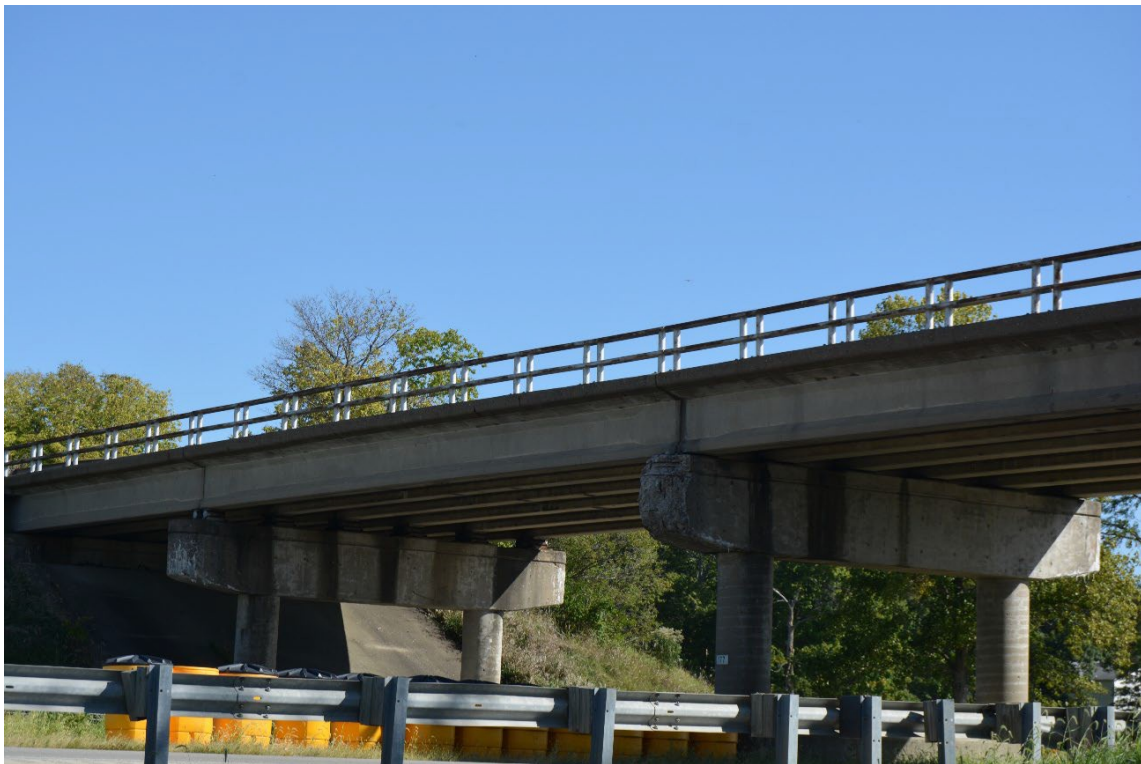
Figure 8. Bridge at 879 N Cottonwood Rd, Urbana
