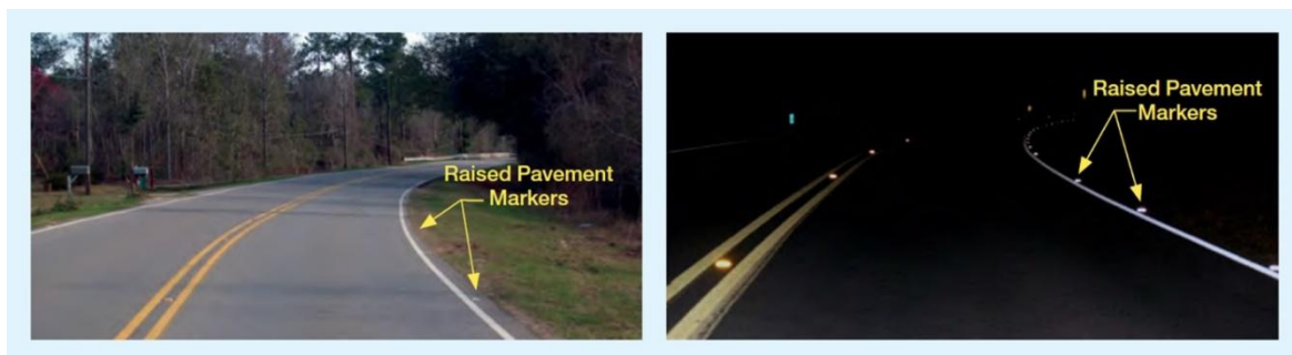
Figure 2.2: Example Images of Raised Pavement Marking (FHWA, 2013)
