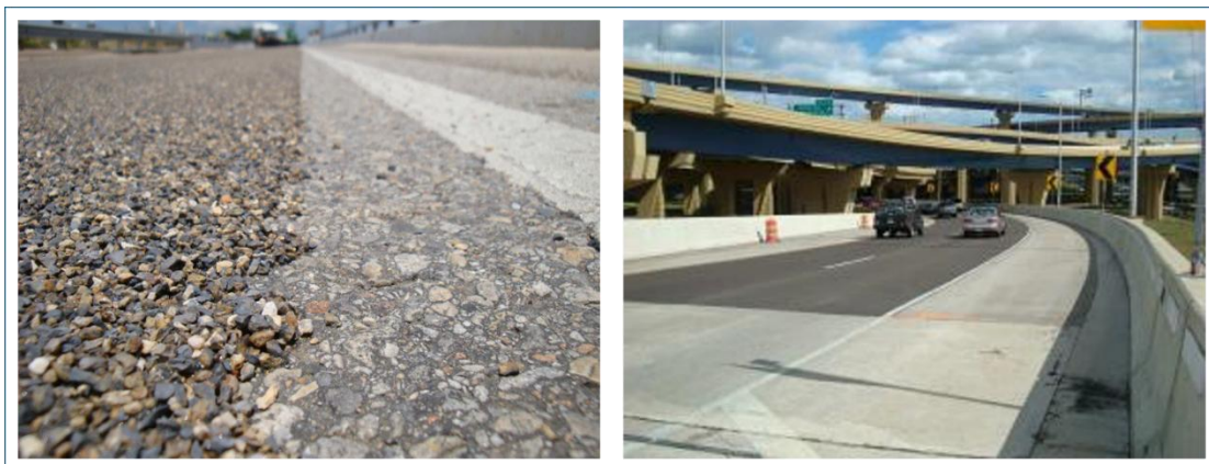
Figure 2.1: Example Images of High-Friction Surface Treatment (Merritt et al., 2020)
