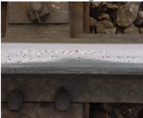
Flaking caused by centralized loading
