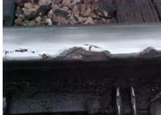
Side shells corrosion
