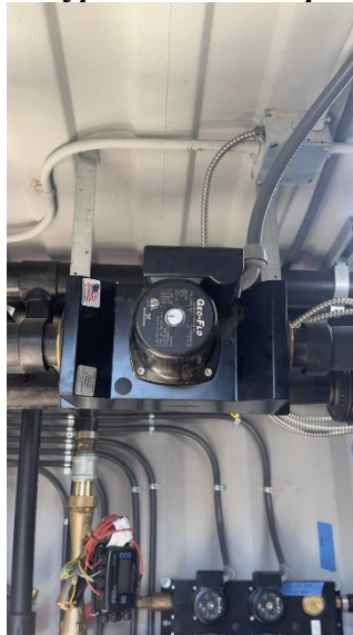
Bypass Flow Pump
