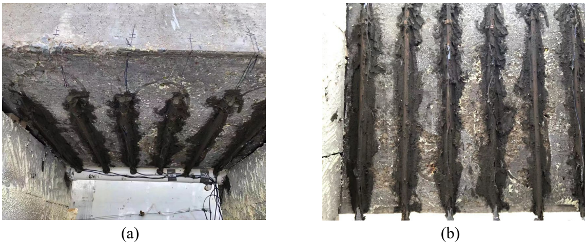
Figure 2.6 Attachment of the heat pipe on the bottom surface of the slab
