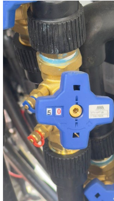
Manifold Balancing Valves
