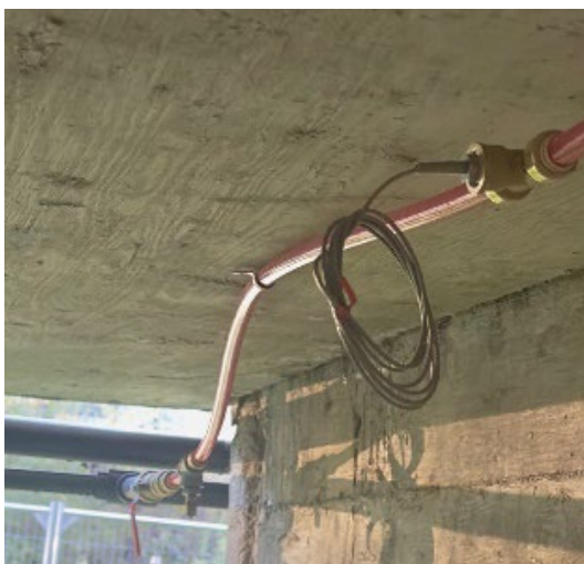
Figure 3.17 Installation of temperature sensors.
