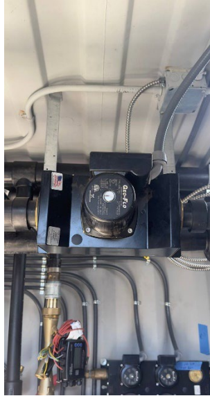
Bypass Flow Pump
