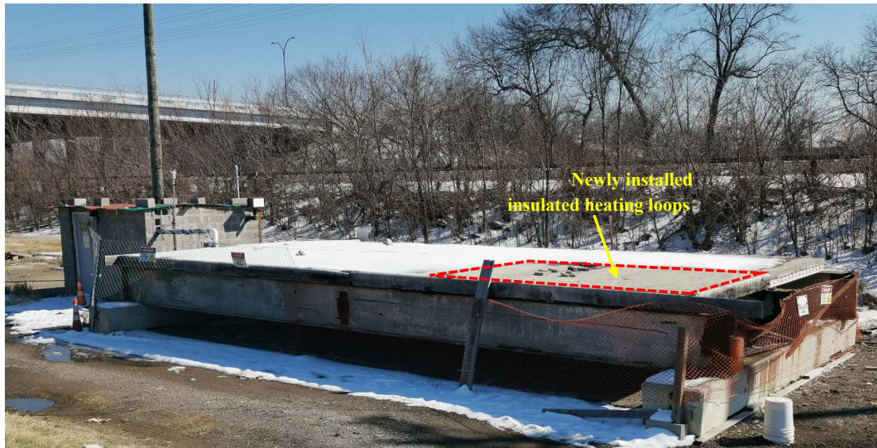
Figure 2.7 The geothermally heated mock-up bridge near Green Oaks BLVD and U.S. Highway 180 overpass bridge, Fort Worth, TX. The heating zone using the developed insulated PEX pipe channel is highlighted.
