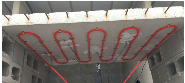
Figure 2.1 Concept design of externally heated bridge deck, i.e., attached hydronic loop (left), and a photo of PEX pipe attachment to a concrete slab (right) (Yu et al. 2020)
