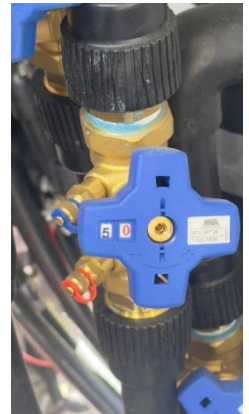
Manifold Flow setter
