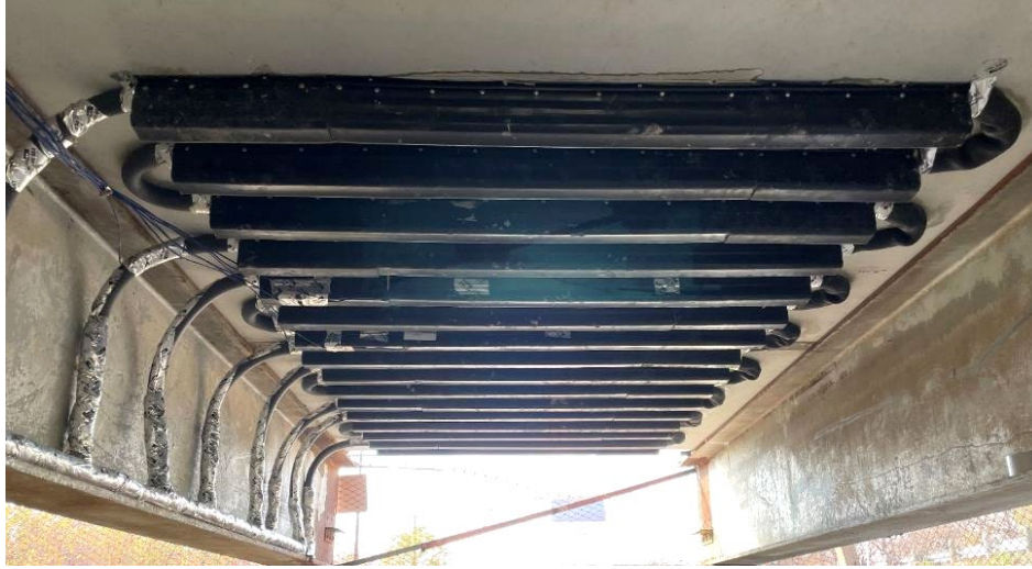
Figure 2.11 Installed insulated PEX pipe channel (bottom view of the bridge deck, the insulated loop section in Figure 2.9 (c))
