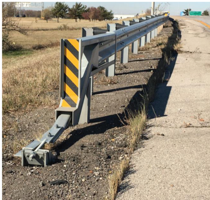
Figure 2.20 SoftStop System by Valtir.
