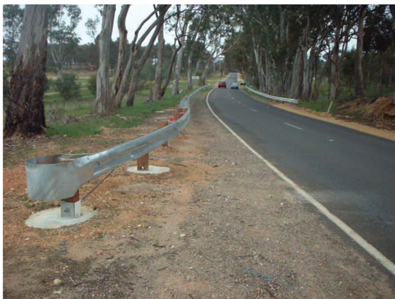
Figure 2.5 Breakaway cable terminal.
