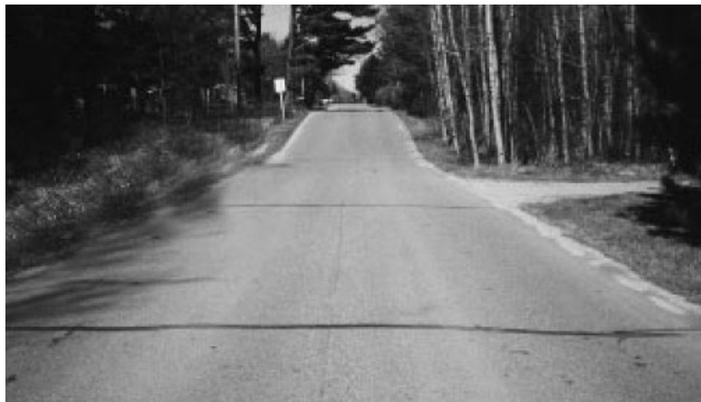
Figure 4-12: Tight and sealed transverse cracks (Source: Walker et al., 2002)
