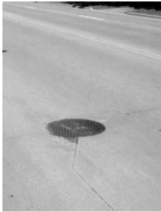
Figure 4-15: Isolated spall at manhole (Source: Walker et al., 2015)
