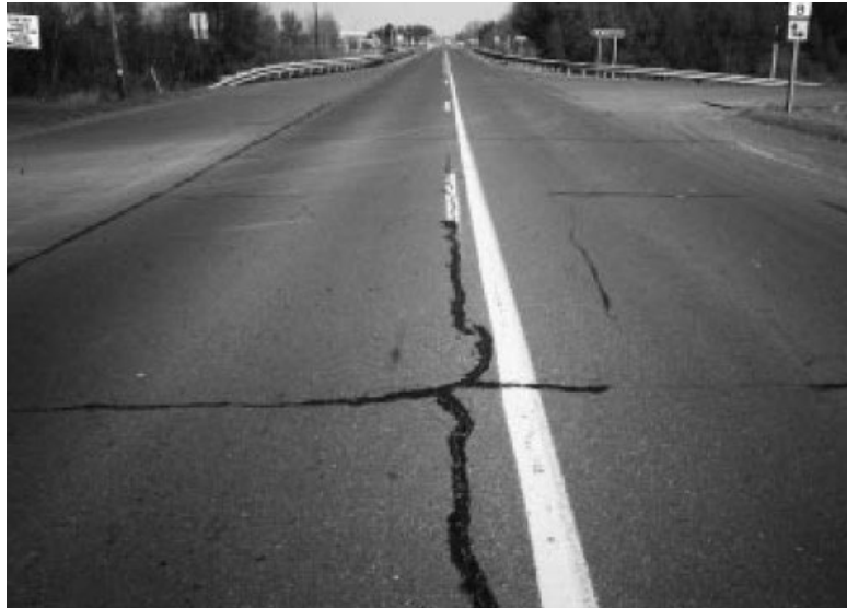
Figure 4-11: Tight and sealed transverse cracks (Source: Walker et al., 2002)
