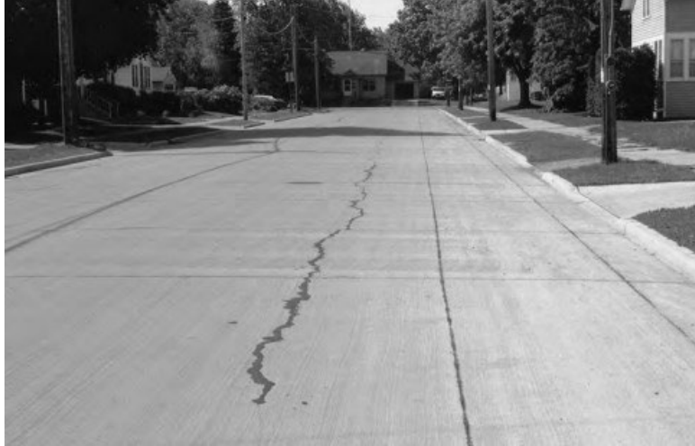
Figure 4-17: Tight and well-sealed isolated meander cracks (Source: Walker et al., 2015)
