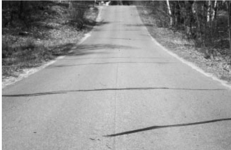
Figure 4-13: Transverse cracks about 10 feet or more apart (Source: Walker et al., 2002)
