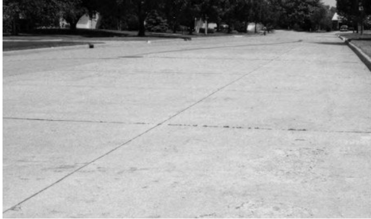
Figure 4-14: Slight scaling of concrete surface (Source: Walker et al., 2015)
