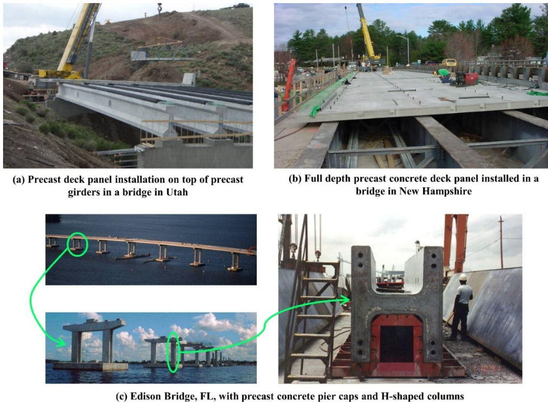
Figure 1. Precast bridge elements used in accelerated bridge construction
