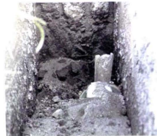
Photo V-4. Summit - Drainage Trench with Drain Pipe.
