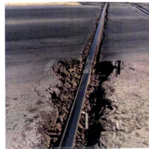
Photo VII-15. Pumping and Breakdown of Asphalt along Rail.
