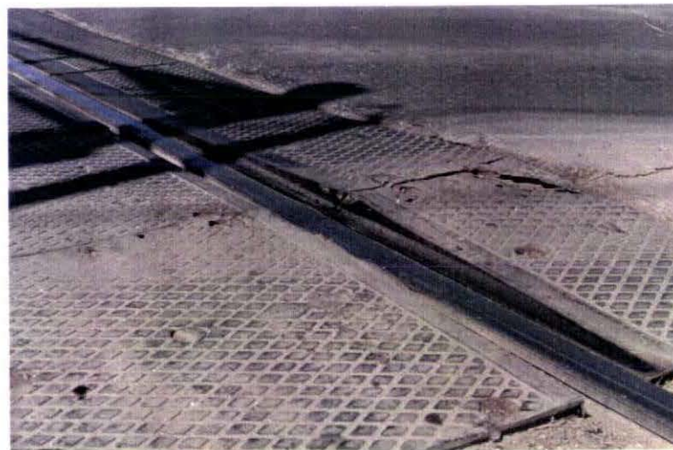
Photo VII-7. Loosening of Panels, Fastener Failure and Loss of Protective Caps.
