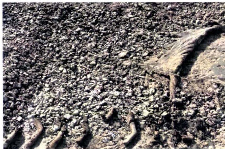
Photo V-32. Rapid City, Second Street - Ballast above Old Fabric and Subgrade Below Fabric.
