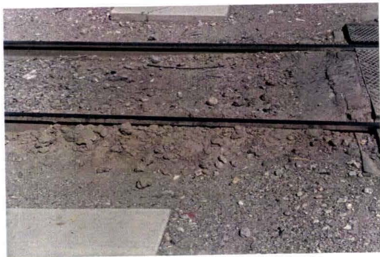
Photo VII-6. Pumping of Track Bed.
