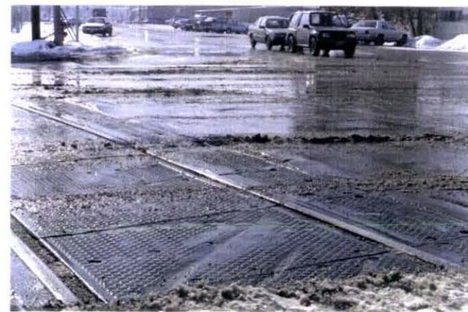
Photo VI-5. Effect of Freeze-Thaw - Frost Heave at Approach to Crossing.
