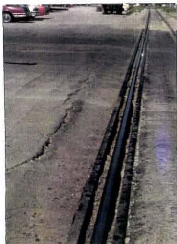
Photo VII-12 and 13. Differential Settlement Between Track and Approaches.
