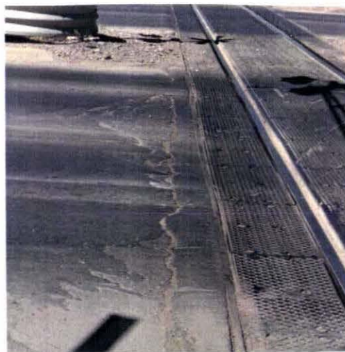
Photo VII-11. Rutting and Cracking of Approach Pavement and Frost Action.
