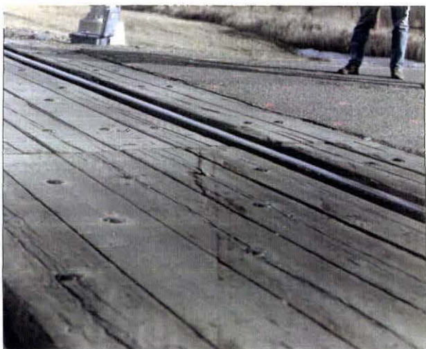
Photo VII-19. Relative Settlement between Crossing and Approach.
