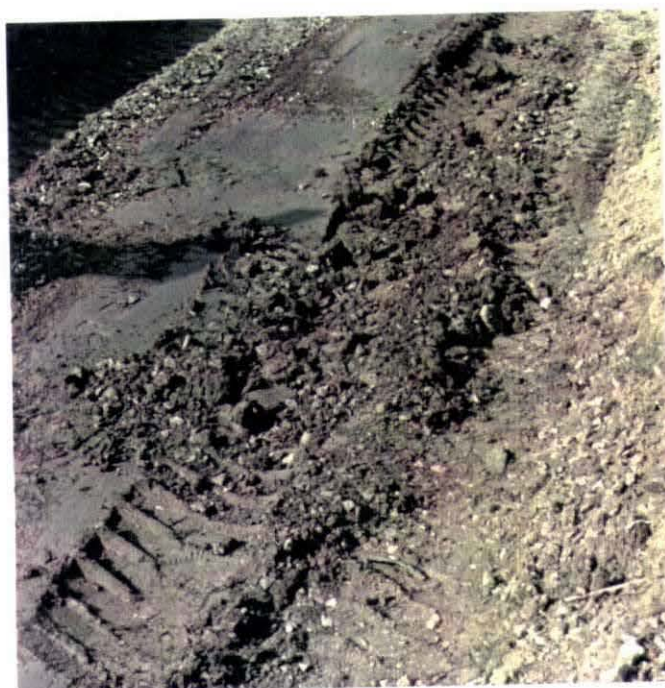
Photo V-37. Rapid City, Second Street - Finished Subgrade and Backfilled Rutting Marks.
