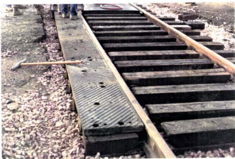
Photo V-17. Aberdeen, Fifth Street - Placement of Gen-Track Panels.
