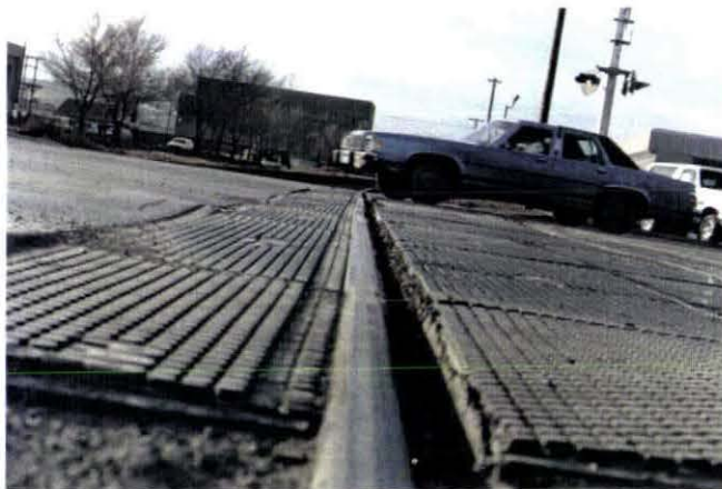
Photo VI-4. Effect of Freeze-Thaw - Mud Squeezing up between Rail and Panel and Outer Panels.
