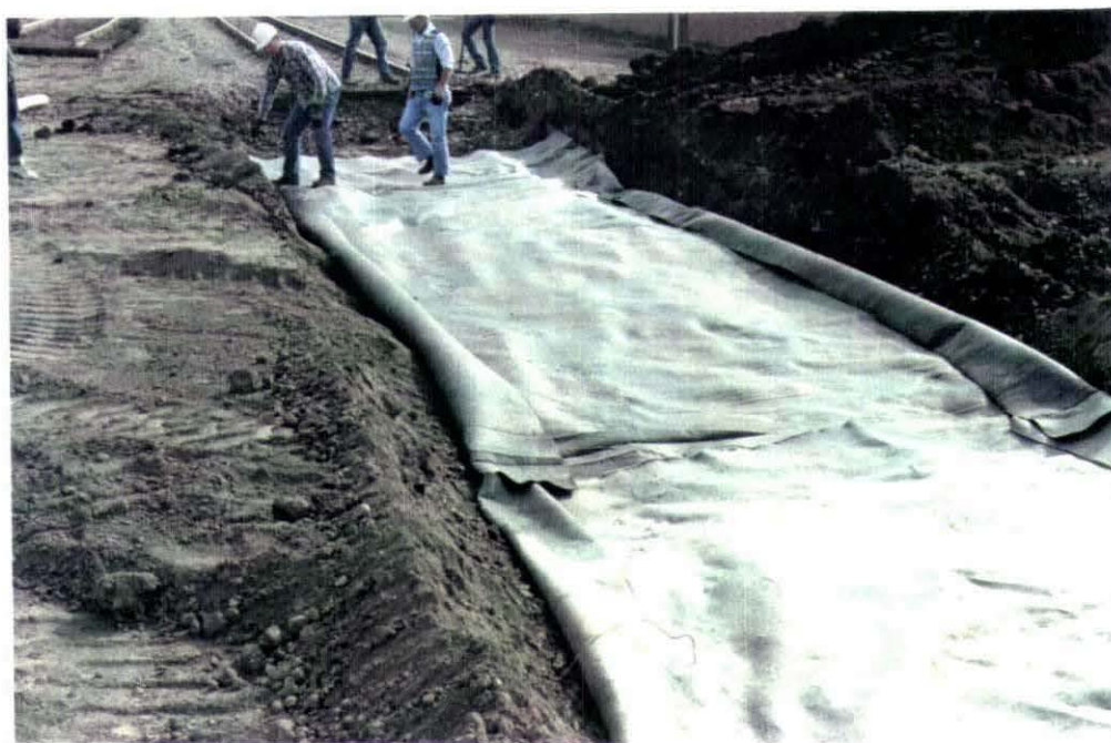
Photo V-38. Rapid City, Second Street - Placement of Fabric.
