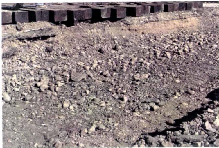
Photo V-13. Aberdeen, Fifth Street - Exposed Subgrade with Loose Cobbles.
