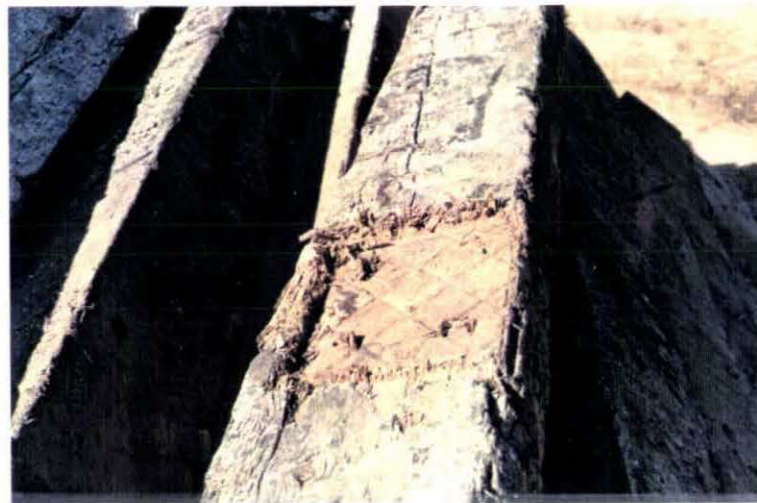
Photo V-26. Sturgis, Ball Park Road - Tie Damaged under Bearing Plate.
