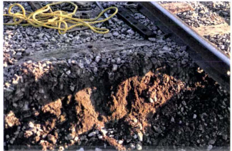
Photo V-34. Rapid City, Second Street - Deteriorated Ballast and Subgrade.
