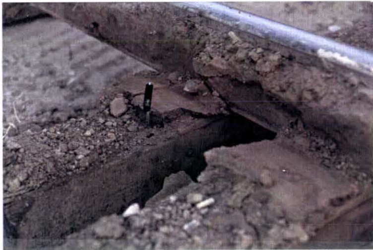
Photo V-33. Rapid City, Second Street - Mud Squeezed in between Bearing Plates and Mud Rail.
