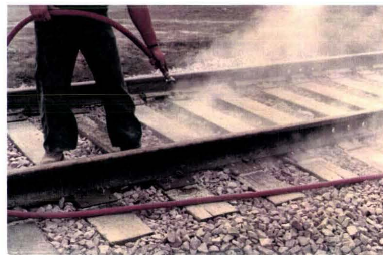
Photo V-16. Aberdeen, Fifth Street - Cleaning of Ties before Placement of Rubber Panels.
