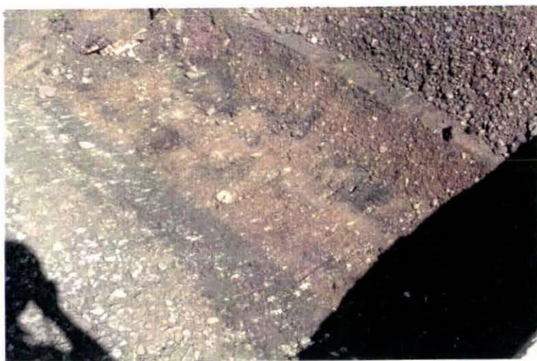
Photo V-7. Summit - Old Ballast, Base Material and Subgrade.
