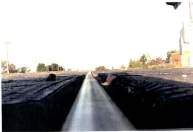
Photo V-3. Summit - Panels Raised Relative to Rail.
