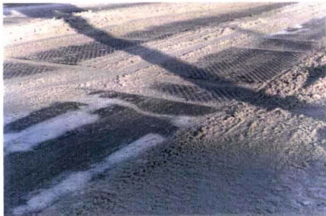
Photo VI-6. Effect of Freeze-Thaw - Frost Heave of Asphalt Approach.
