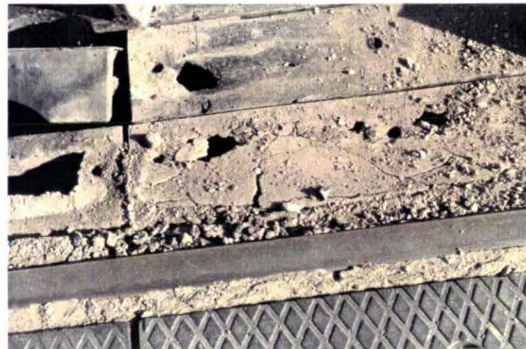
Photo V-6. Summit - Mud between Panels and Spacers.
