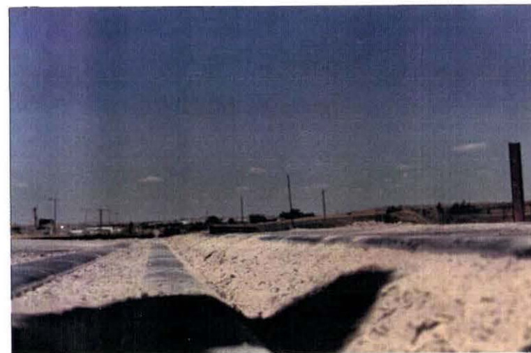
Photo VII-14. Differential Settlement between Main Rail and Mud Rail.
