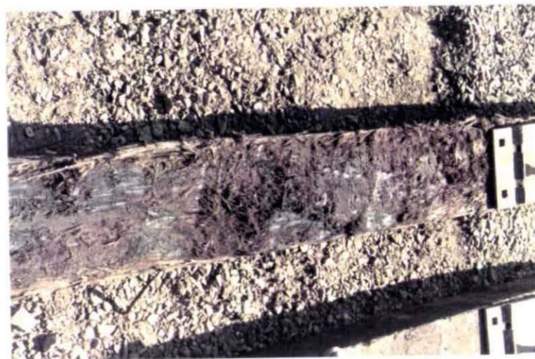
Photo V-10. Aberdeen, Fifth Street - Tie Damaged by Contact with Ballast.
