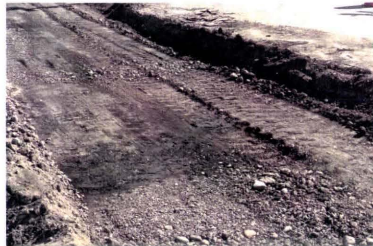
Photo V-14. Aberdeen, Fifth Street - Exposed Clay Subgrade.
