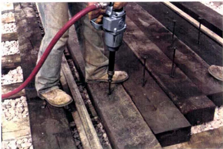
Photo V-21. Aberdeen, 12 Street - Fastening of Timbers with Camcar Screws.
