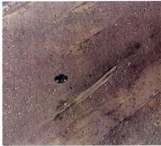
Photo VII-21 and 22. Snow Plow Damage.
