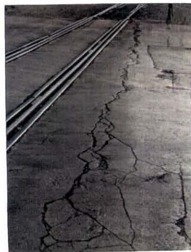
Photo VII-12 and 13. Differential Settlement Between Track and Approaches.
