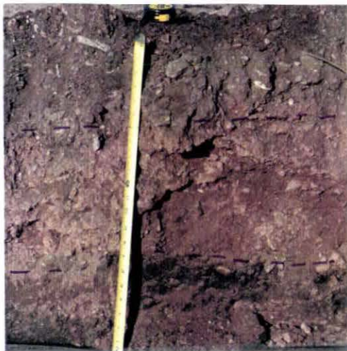
Photo V-25. Sturgis, Ball Park Road - Roadbase and Subgrade Exposed in Excavation.
