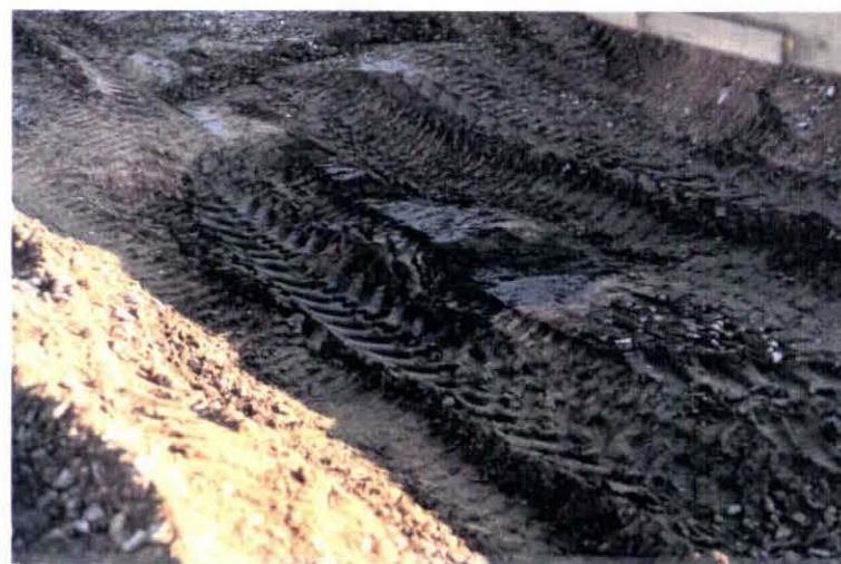
Photo V-28. Sturgis, Ball Park Road - Close-up of Rutting from Frontloader Tires.
