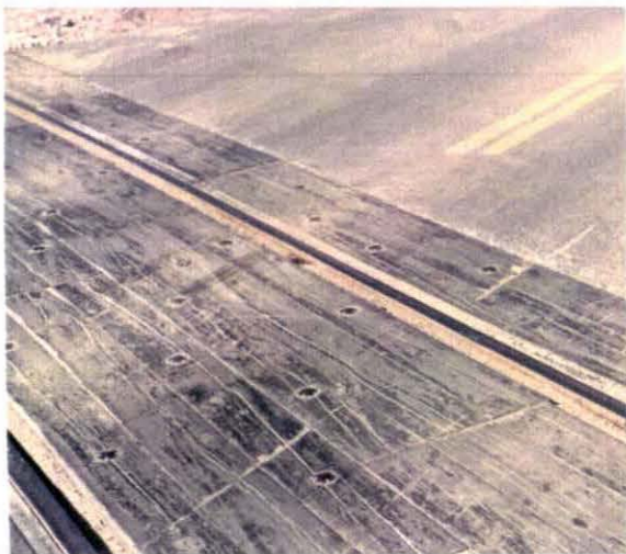
Photo VII-21 and 22. Snow Plow Damage.
