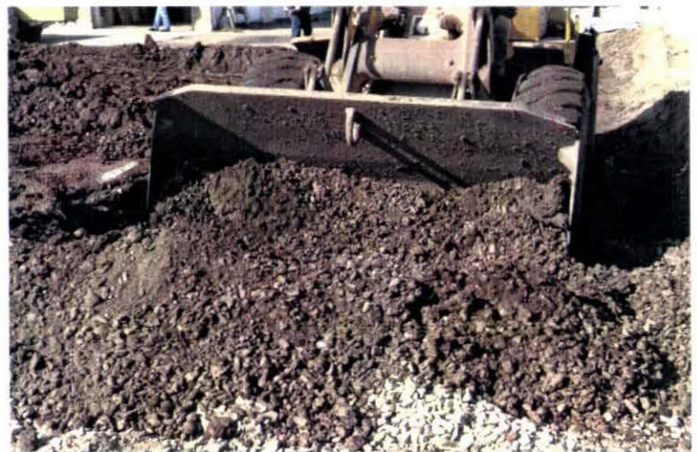
Photo V-36. Rapid City, Second Street - Removal of Old Ballast.
