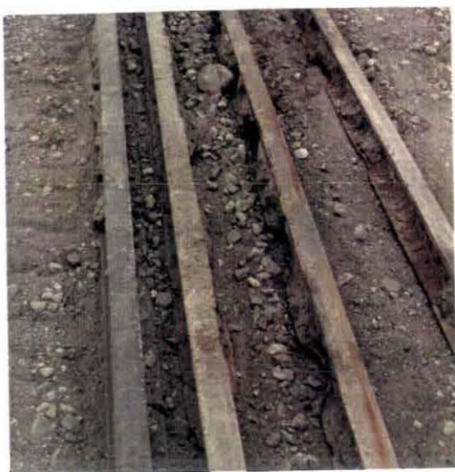
Photo V-19. Aberdeen, 12 Street - Corroded Rails.
