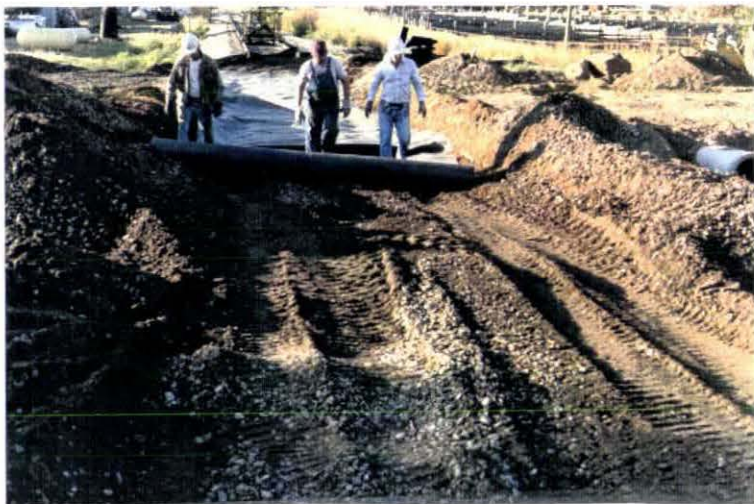
Photo V-29. Sturgis, Ball Park Road - Placement of Fabric.
