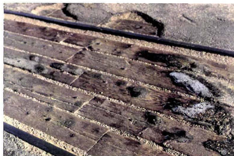
Photo VII-20. Wear by Traffic and Protruding Fasteners.
