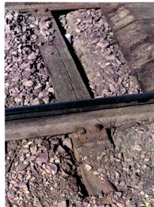
Photo VII-23. Pumping and Track Deflection.
