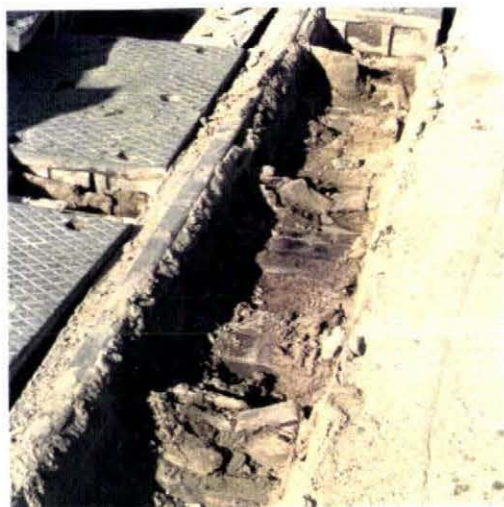
Photo VII-4. Debris Forced Under Panels.
