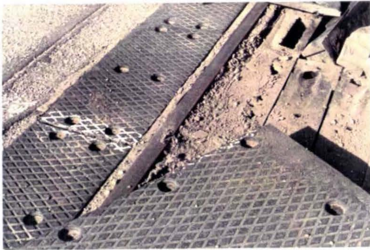
Photo V-1. Summit - Old True Temper Crossing. Panels Resting Rubber Spacers
