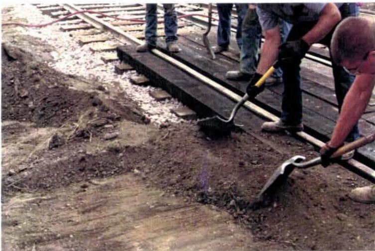
Photo V-23. Aberdeen, 12 Street - Placement of Soil Backfill.
