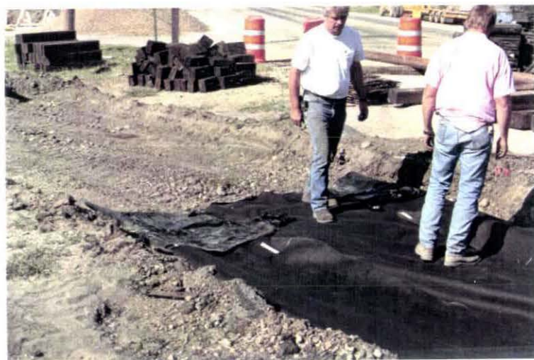
Photo V-15. Aberdeen, Fifth Street - Placement of Fabric.
