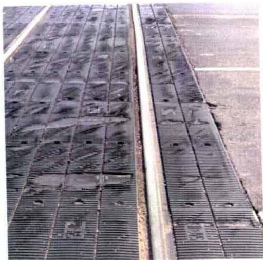
Photo VII-10. Panel Wear and Snowplow Damage.
