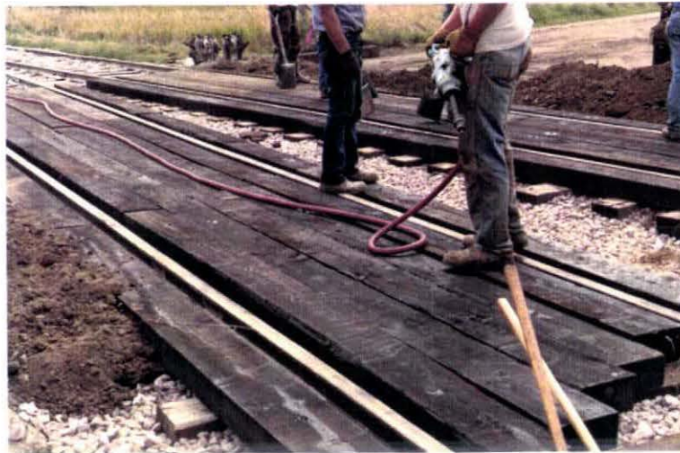
Photo V-22. Aberdeen, 12 Street - Completed Crossing Showing Uneven Timbers.
