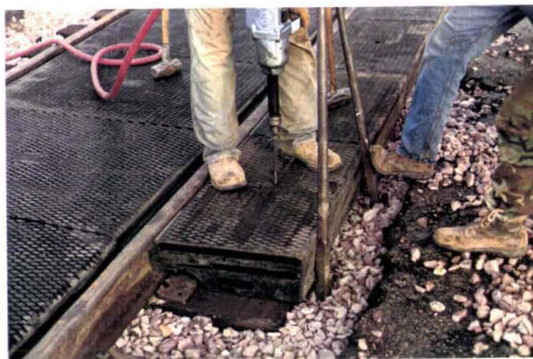
Photo V-18. Aberdeen, Fifth Street - Placement of HI-RAIL Panels.
