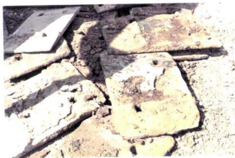
Photo V-12. Aberdeen, Fifth Street - Mud Squeezed in between the Rail and the Bearing Plates.
