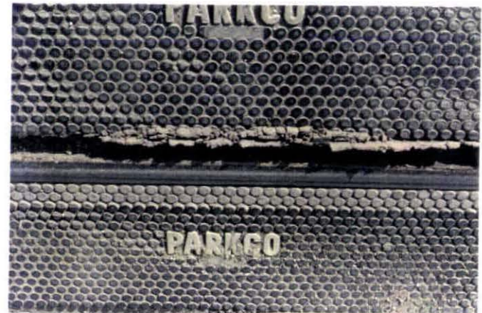
Photo VI-3. Effect of Freeze-Thaw - Mud Squeezing up between Rails and Panel.
