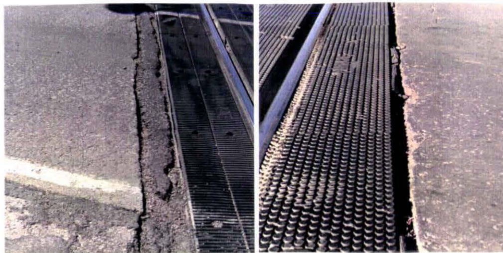
Photo VII-2 and 3. Failure of Asphalt and Wood Headers.
