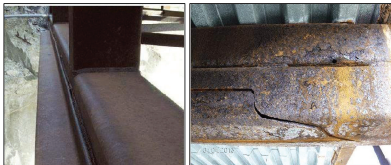
Figure 2.3 View of fractures in the floor beam and the longitudinal attachment to the bottom chords.
