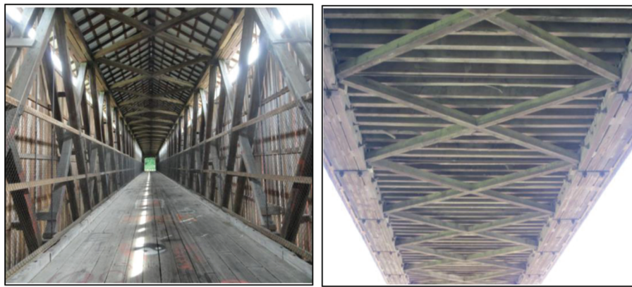
Figure 2.8 View of the top and the bottom deck of the timber bridge.
