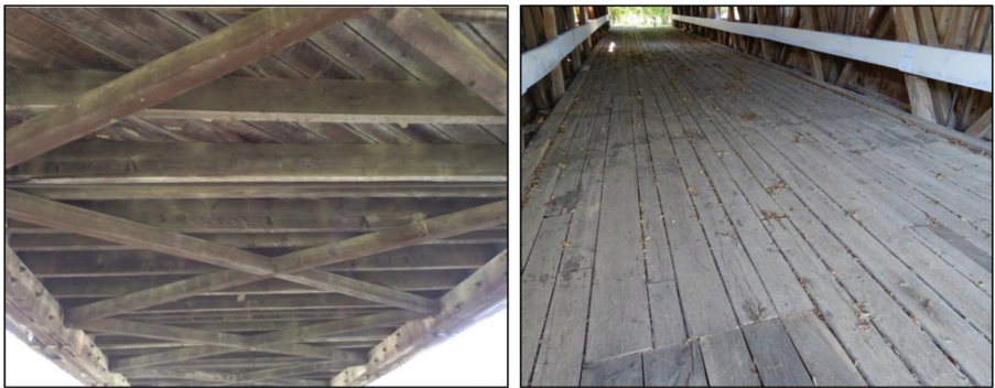
Figure 4.1 Example of timber deck with two layers planks, diagonal and longitudinal planks.
