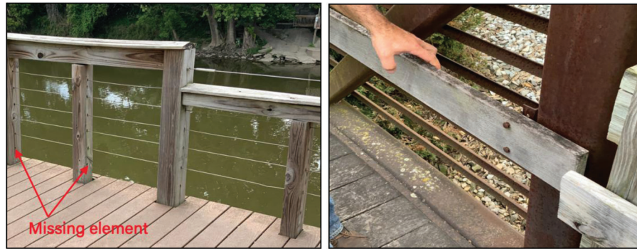
Figure 2.5 View of missing element and inadequate anchorage of bridge railing.
