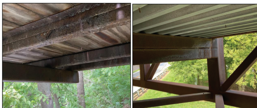
Figure 2.4 View of the stringers and floor beam in timber and a stay-in-place concrete deck.
