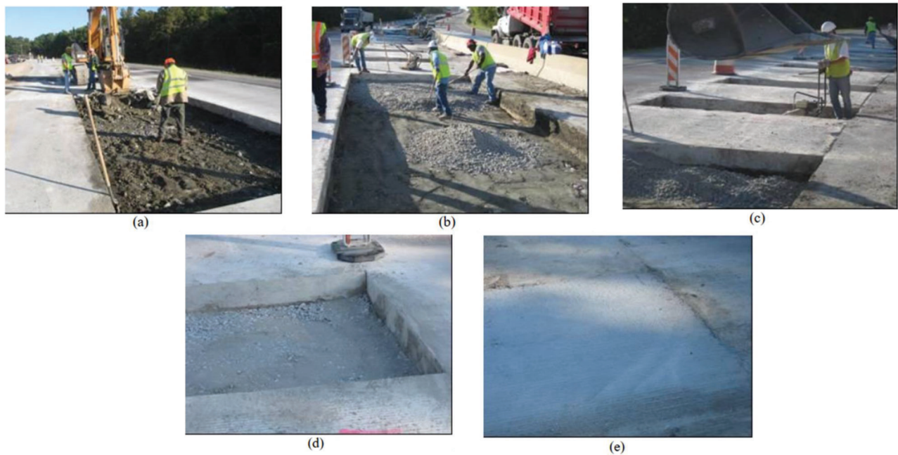
Figure 2.7 Full-depth patching: (a) removing the existing slab, (b) placing the subbase materials, (c–d) compacting the subbase, and (e) the new slab surface.
