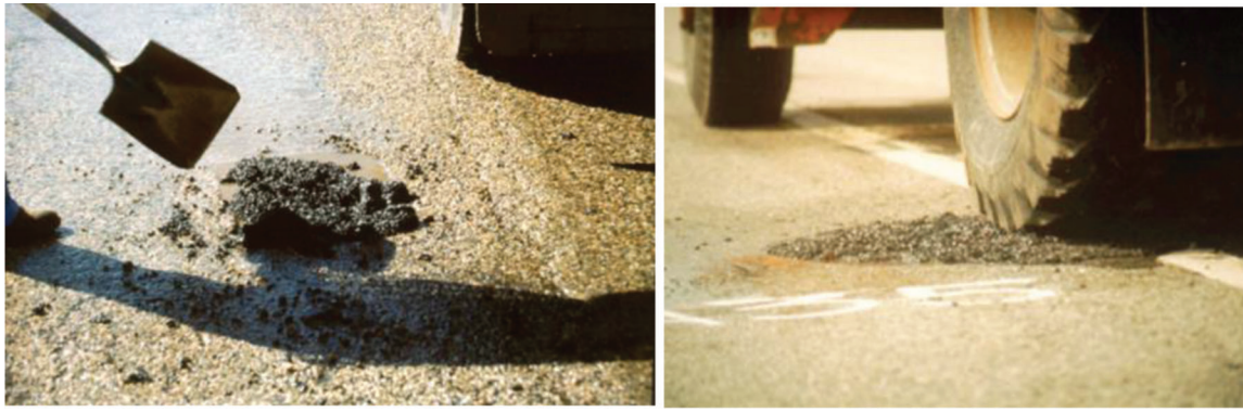
Figure 2.2 Throw-and-roll procedure.
