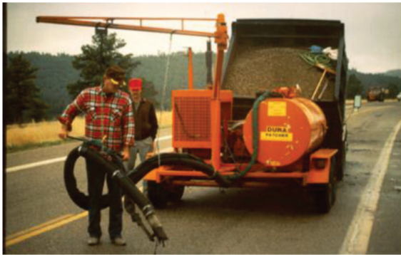
Figure 2.4 Spray injection method.
