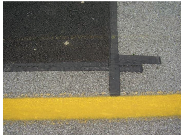
Figure 2.5 Edge sealing method.
