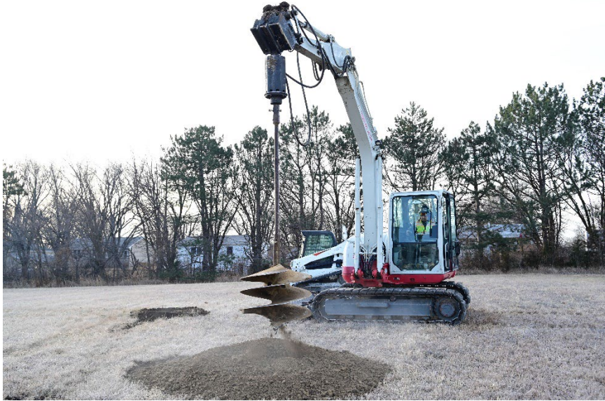
Figure 3.7 Auger Drive Digger used to excavate the holes
