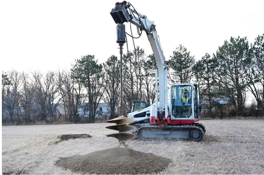
Figure F.1 Drilling operations
