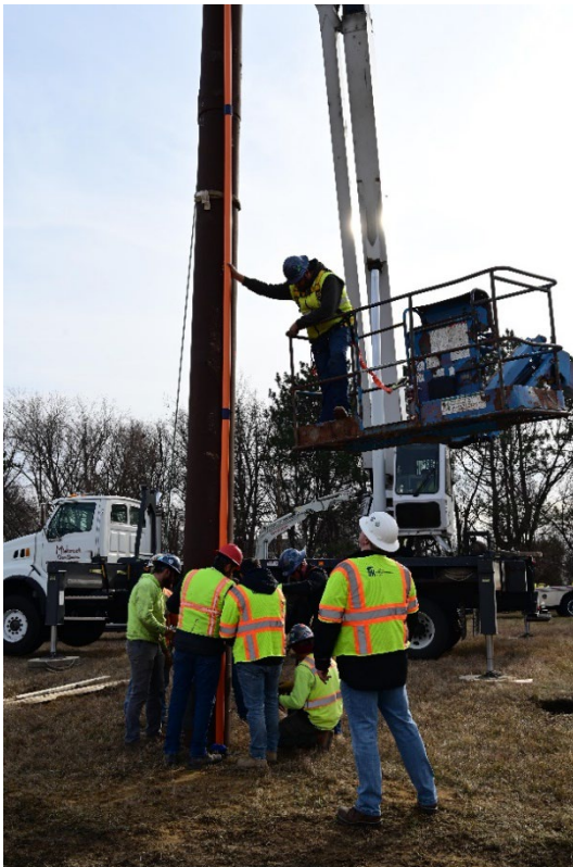
Figure 3.10 Process of attaching the inclinometer casing to the pole
