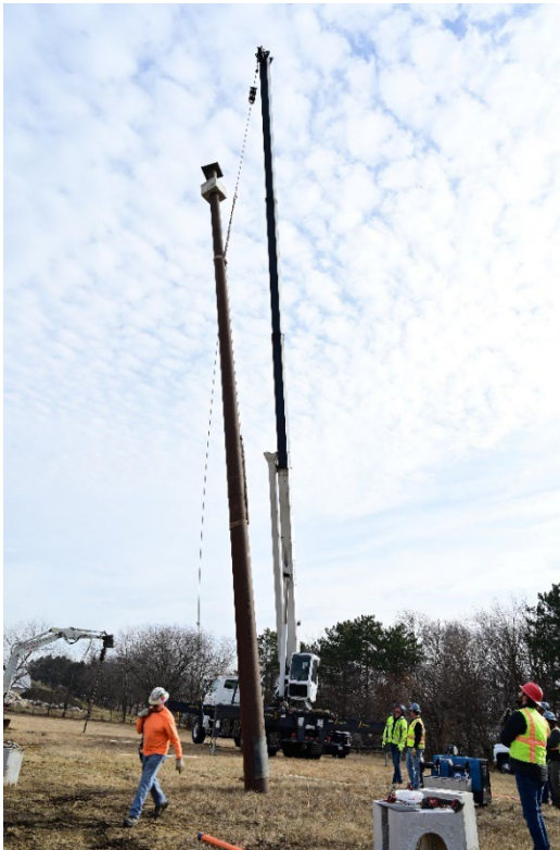
Figure 3.9 Lifting the pole using a crane and placing it inside the hole
