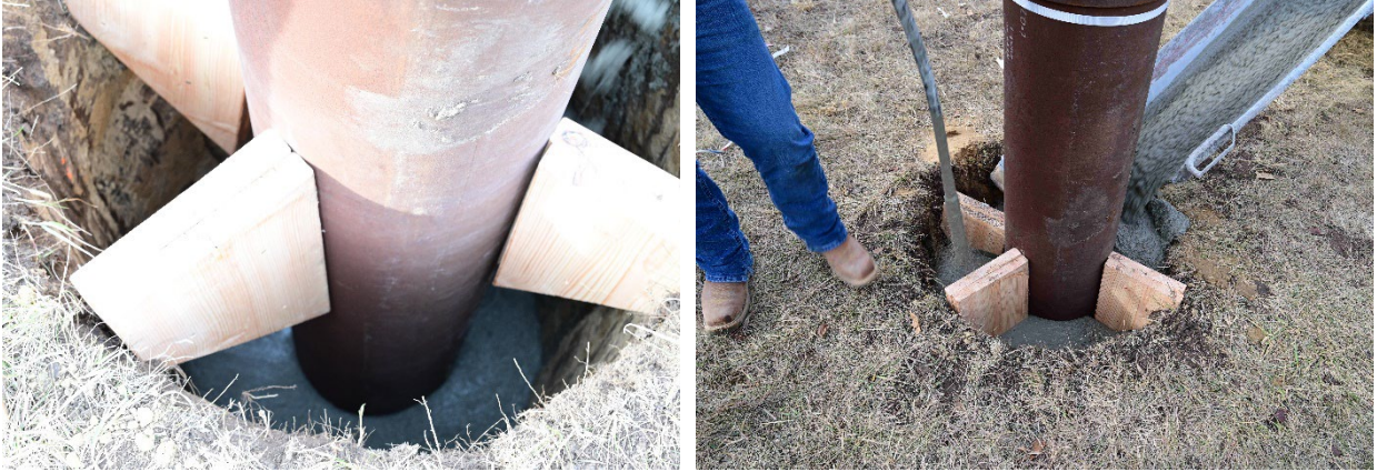
Figure F.3 Placing the concrete backfill and using an electric vibrator to ensure proper compaction
