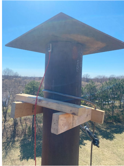
Figure 4.7 Steel cable connected to the top of the pole for static and pluck tests
