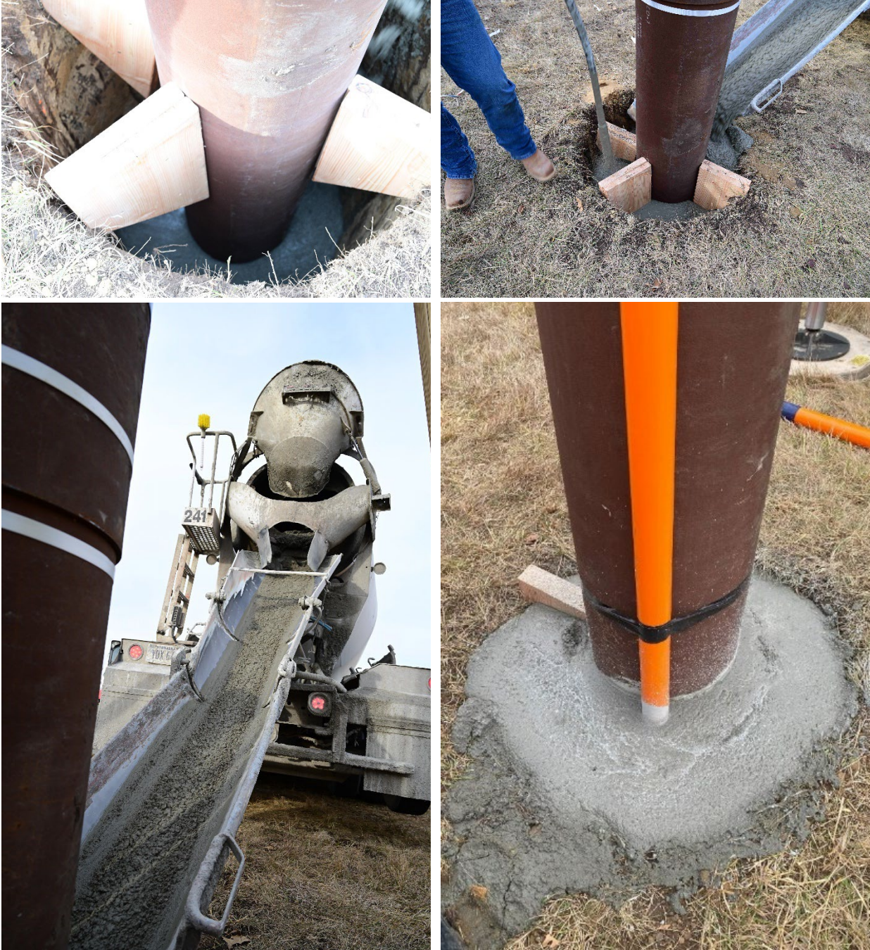
Figure 3.12 Placing the concrete backfill and using an electric vibrator to ensure proper compaction
