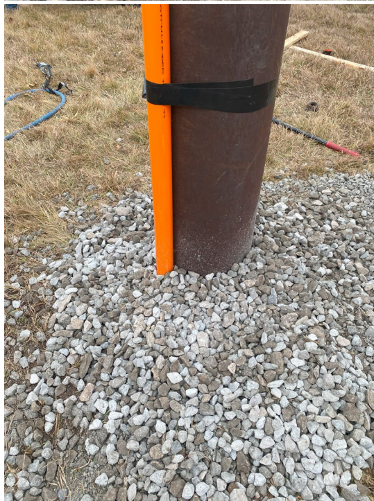
Figure 3.13 Placing the gravel backfill and using an electric tamper to ensure uniformly compacted around the annulus
