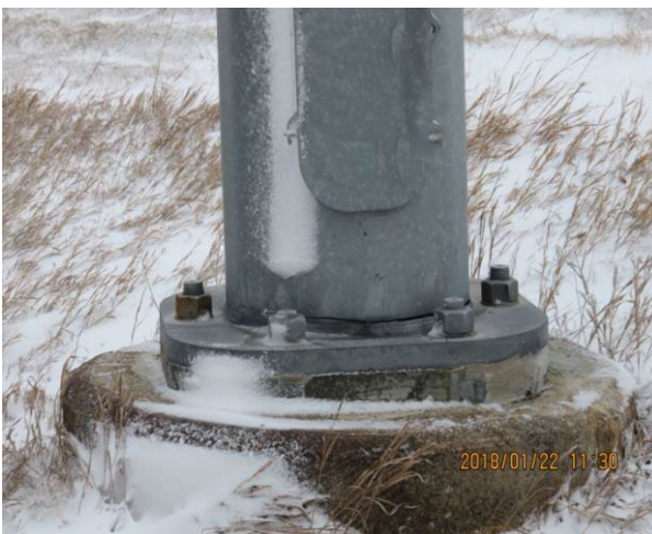
(a) High-mast Tower Base Plate, Anchor, Non-shrink Grout, and Cast-in-Place Foundation
