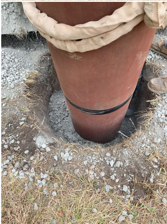
Figure 3.13 Placing the gravel backfill and using an electric tamper to ensure uniformly compacted around the annulus
