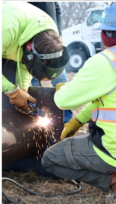
Figure 3.8 Installing the concrete donuts and welding the steel plates to the top of the poles
