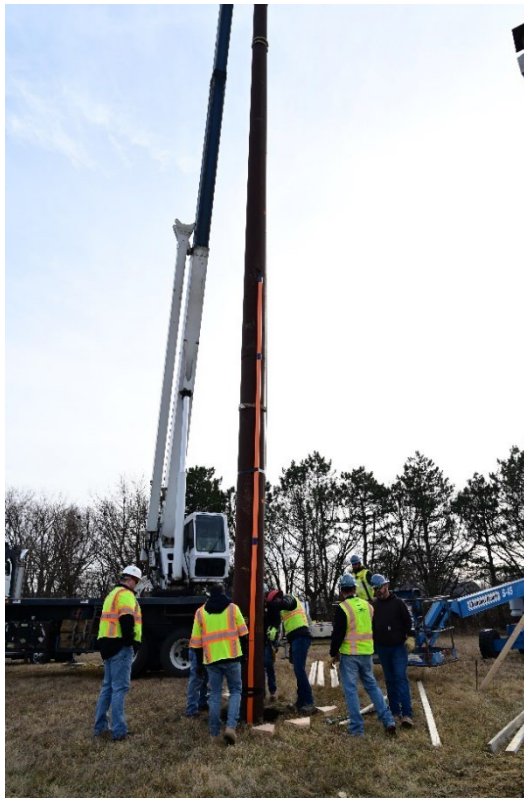
Figure 3.10 Process of attaching the inclinometer casing to the pole
