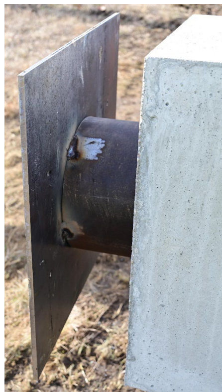
Figure 3.8 Installing the concrete donuts and welding the steel plates to the top of the poles
