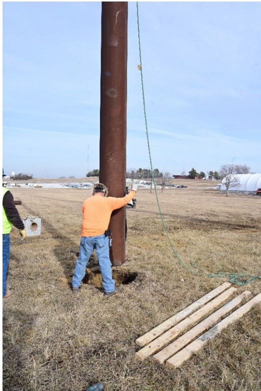
Figure 3.9 Lifting the pole using a crane and placing it inside the hole
