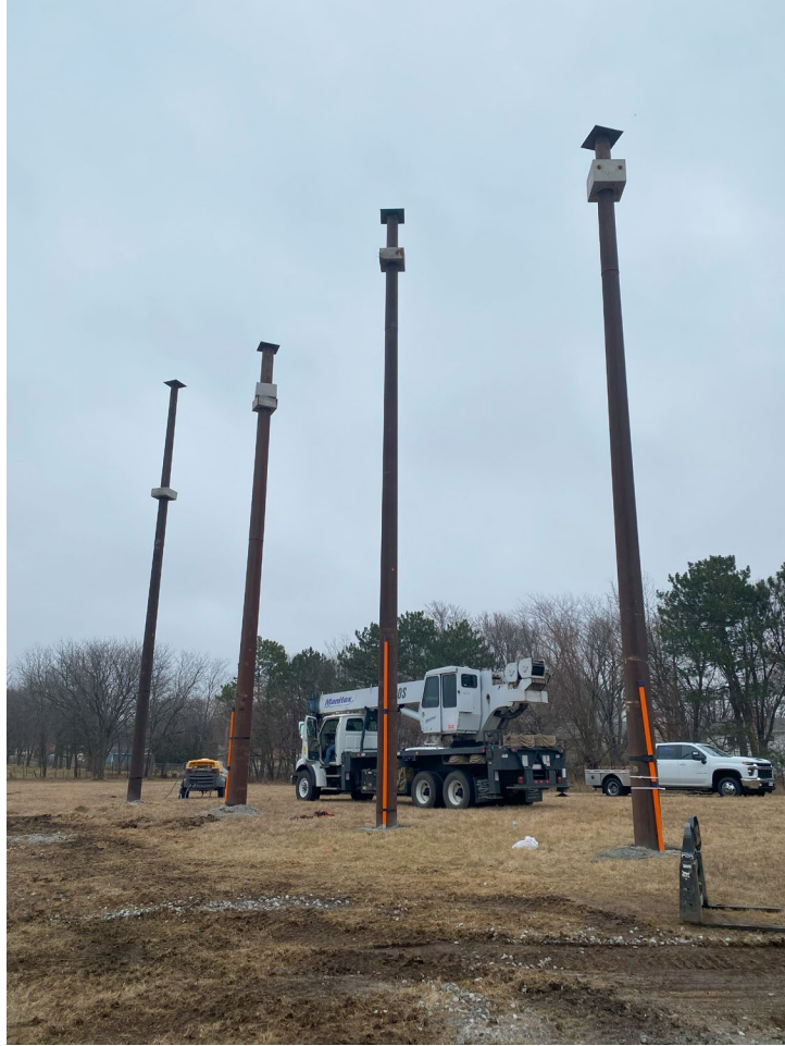
Figure 3.14 Poles in the field at the end of the installation process
