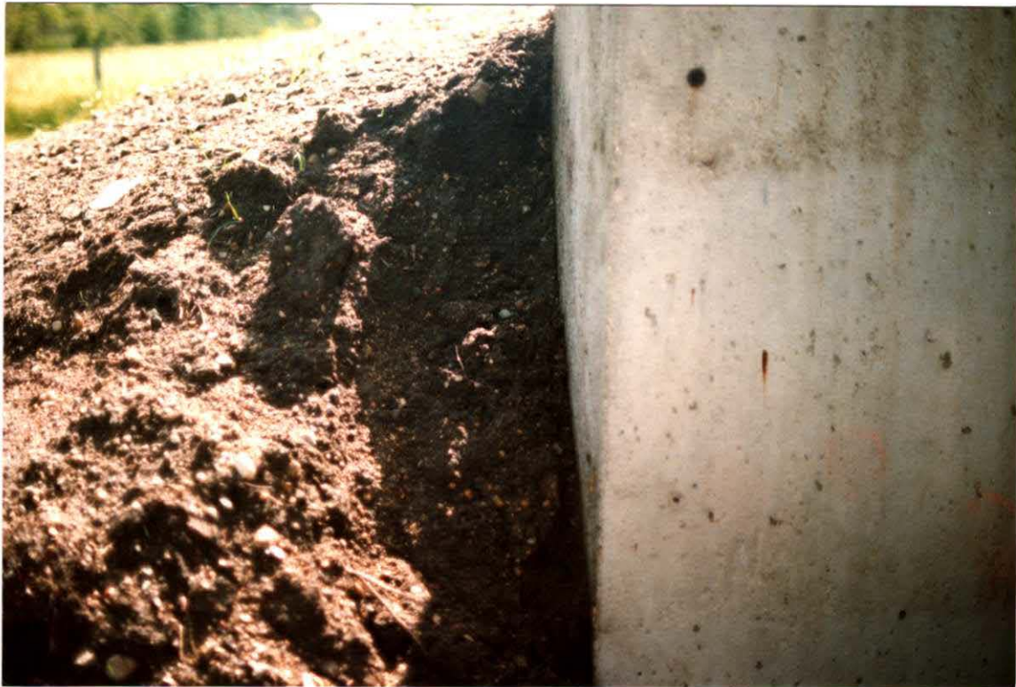
Figure 5-17. Erosion around wing wall following March rainstorm.
