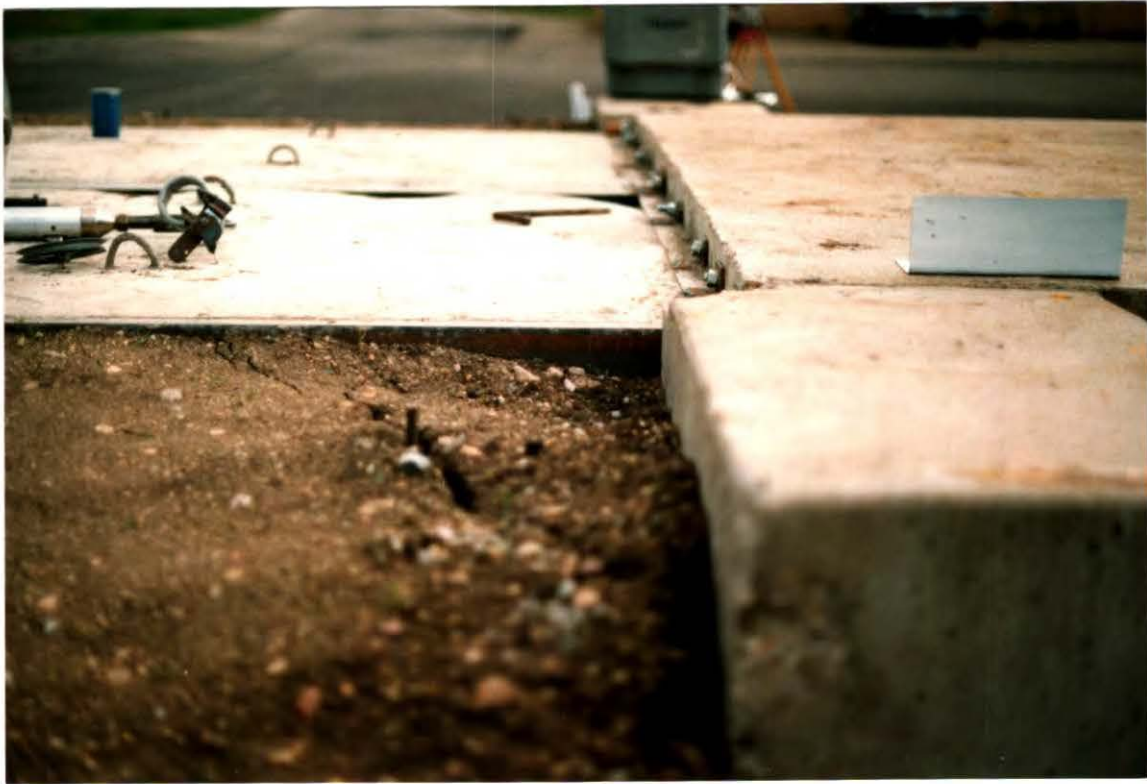
Figure 5-14. Settlement of north embankment next to approach slab and wing wall. February cycle.
