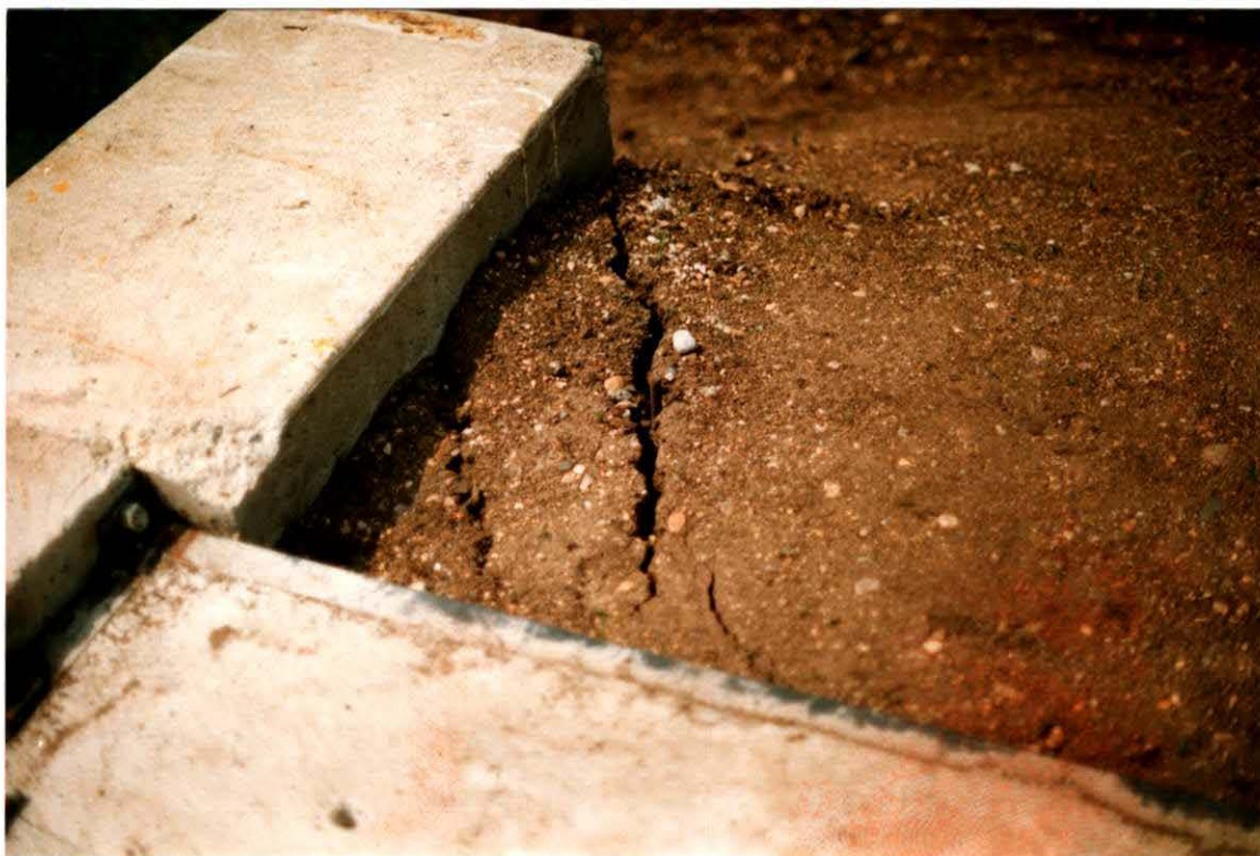
Figure 5-13. Crack development in front of north wing wall during winter month cycles.
