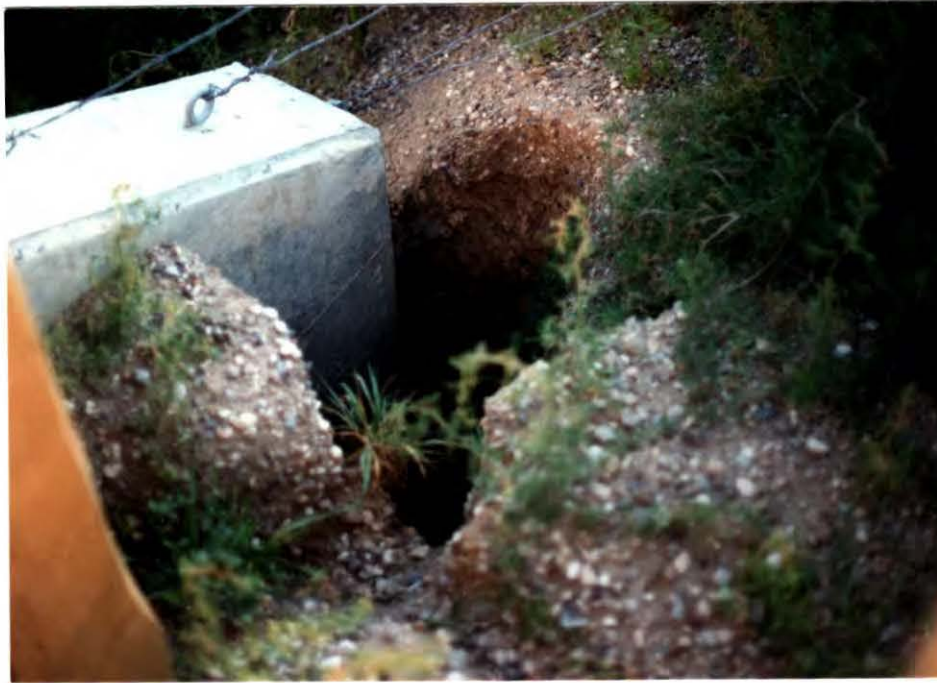
a. Erosion around wing wall. Structure No. 48-440-253 on SD 53 in Mellette Co.
