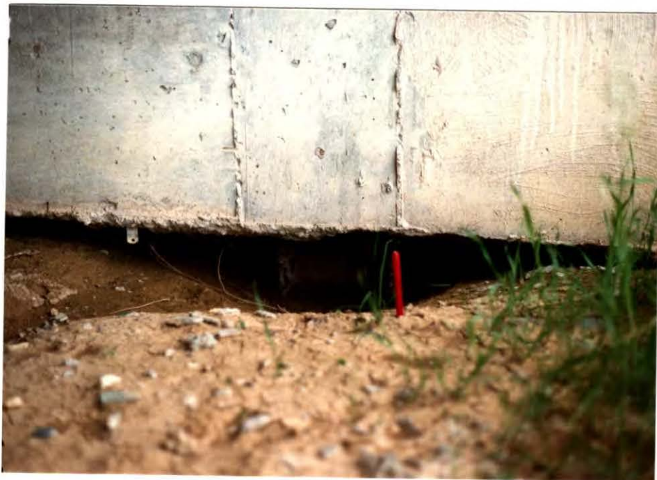
Figure 3-3. Photograph of void development under abutment, note exposure of H-pile. Structure No. 36-071-077, on I-90 eastbound at mile marker 125.53 in Jackson Co.
