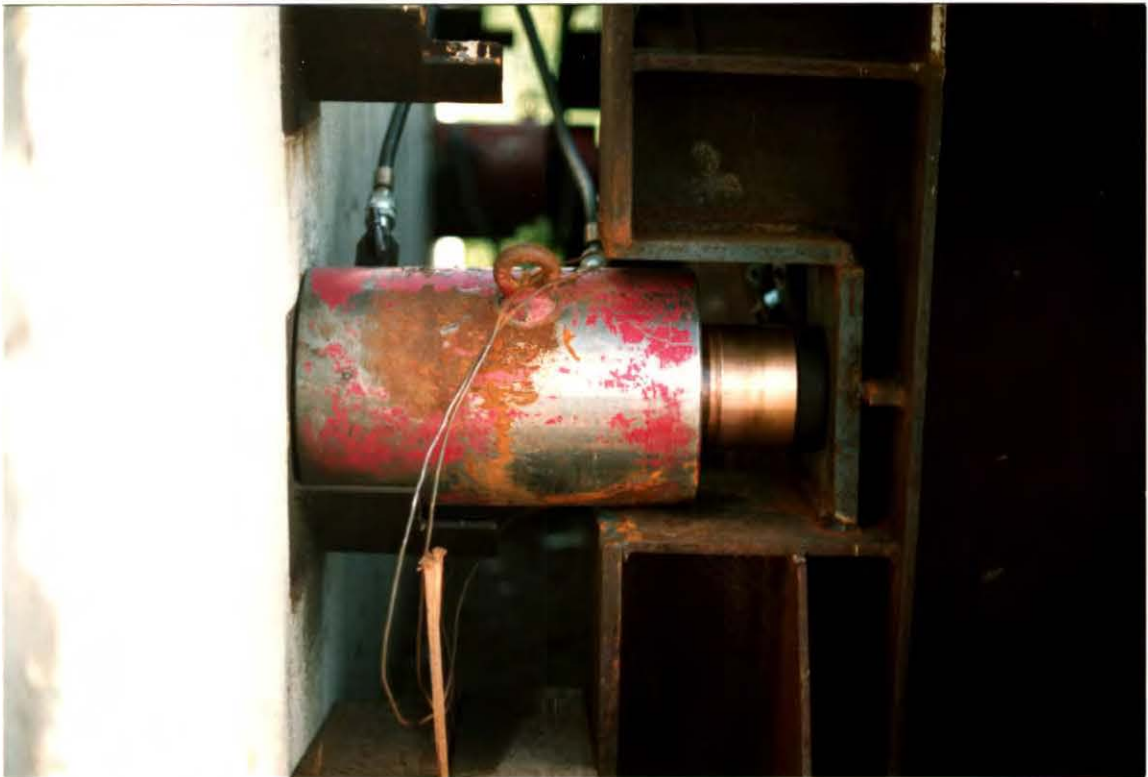
b. Hydraulic jack placement on main bridge beams. Jacks used to push abutment into approach backfill.
