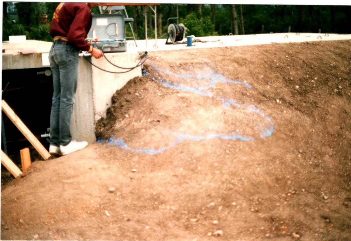
Figure 5-12. Outline of a wedge of failed embankment. Failure occurred during September expansion step.
