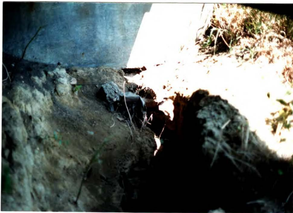
b. Erosion of berm in front of abutment. Structure No. 14-100-200 on SD 50 in Clay Co.
