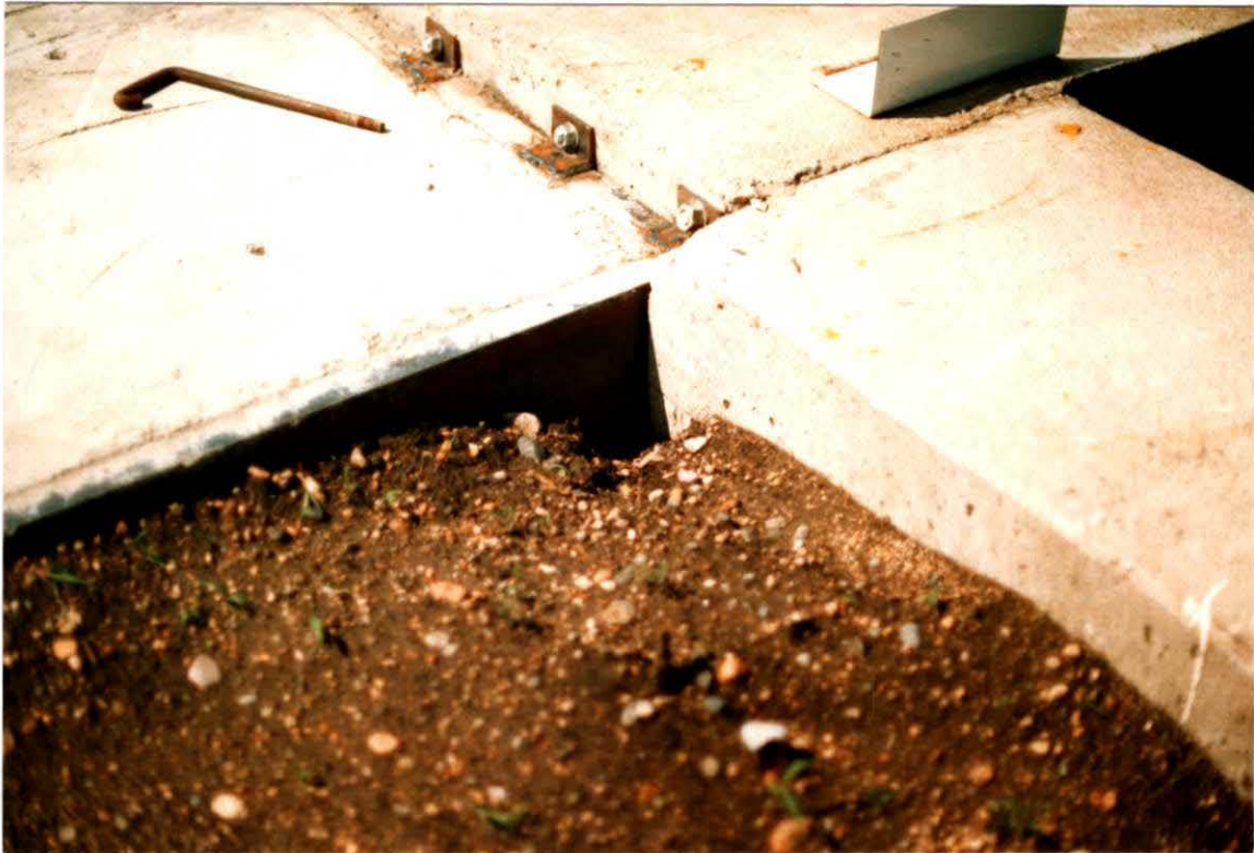
Figure 5-16. Void development exposed on north embankment after a March rainstorm.
