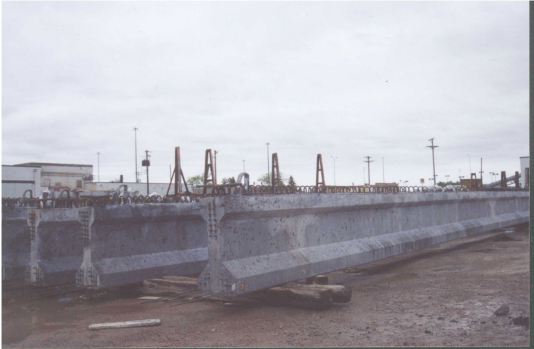
Figure 7. Magnetoelastic sensors installed in a fabricated beam
