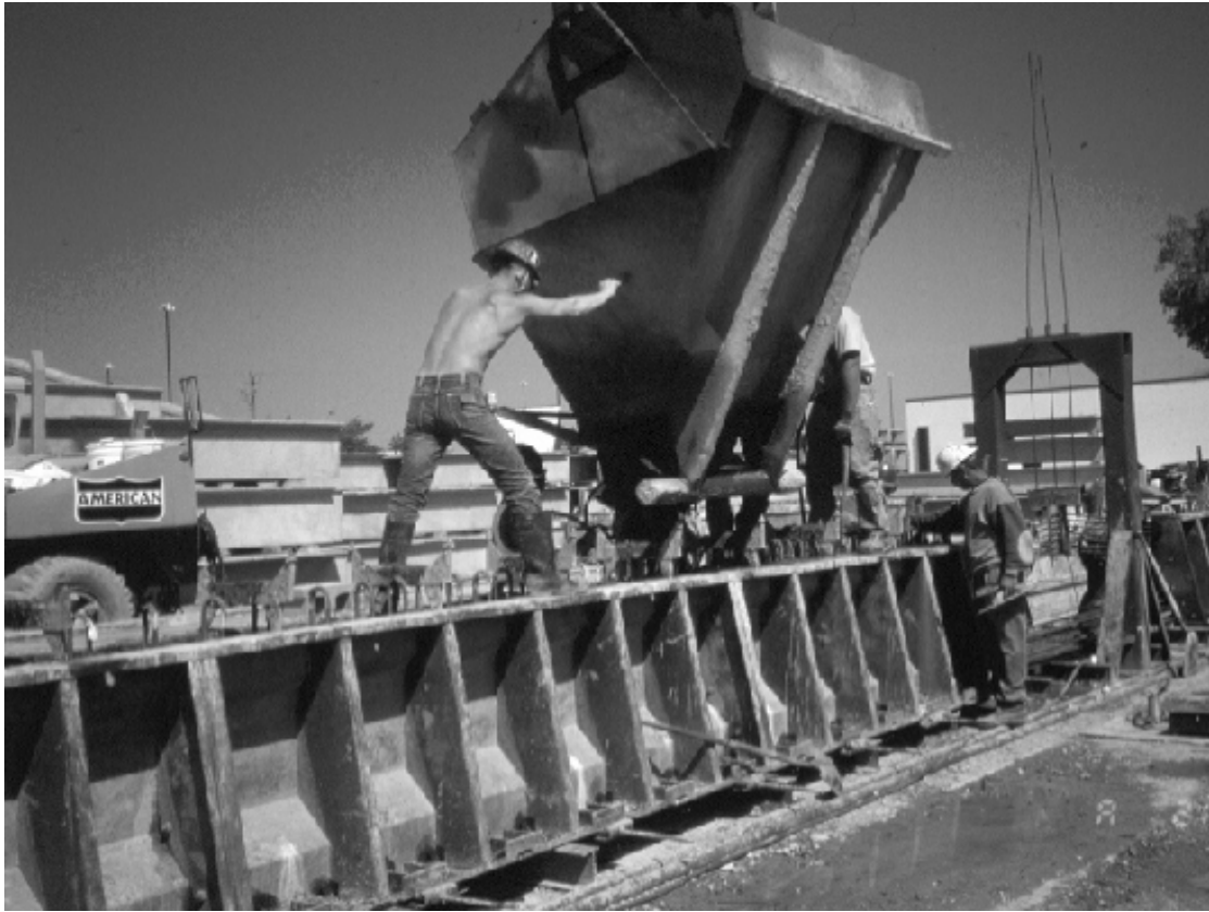
Figure 3.46 Casting one of the girders for bridge 1.
