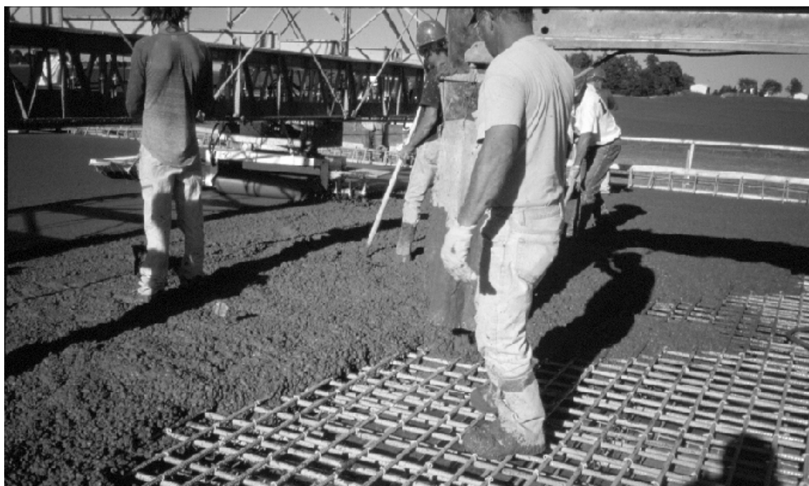
Figure 3.47 Deck placement on bridge 1.
