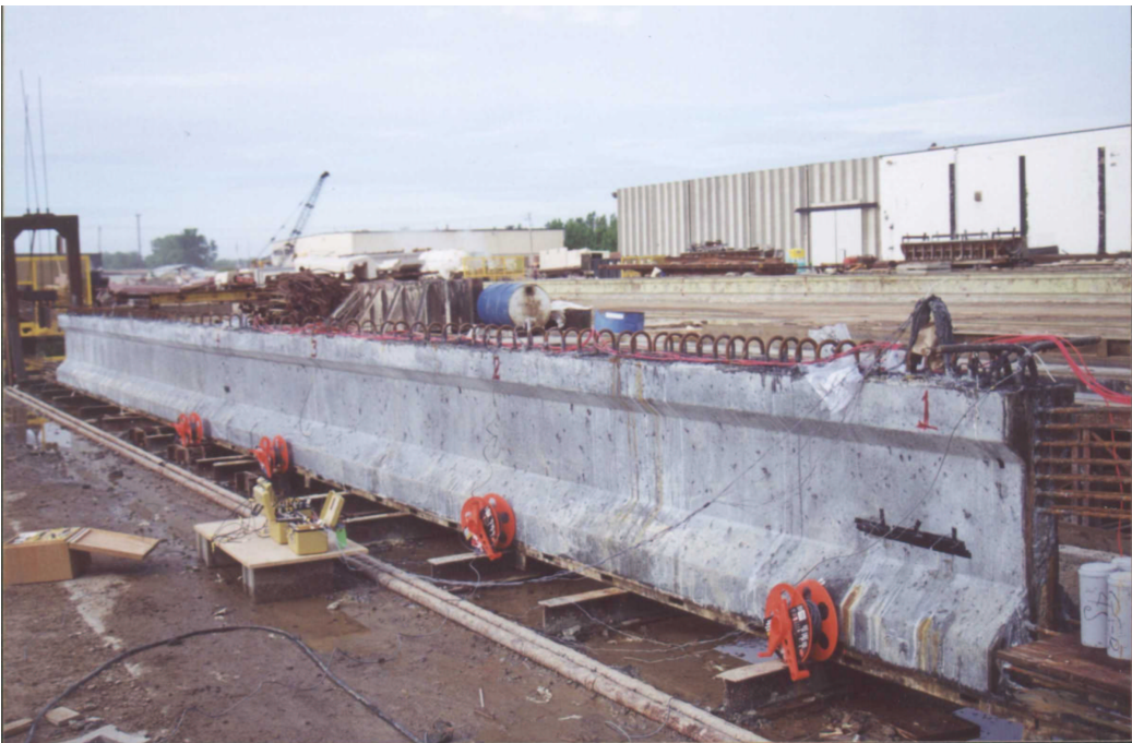
Figure 8. Fabricated pre-tensioned I-beams
