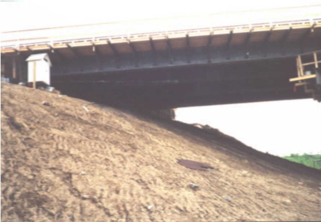
Figure 9. Final position of the beam at the site.
