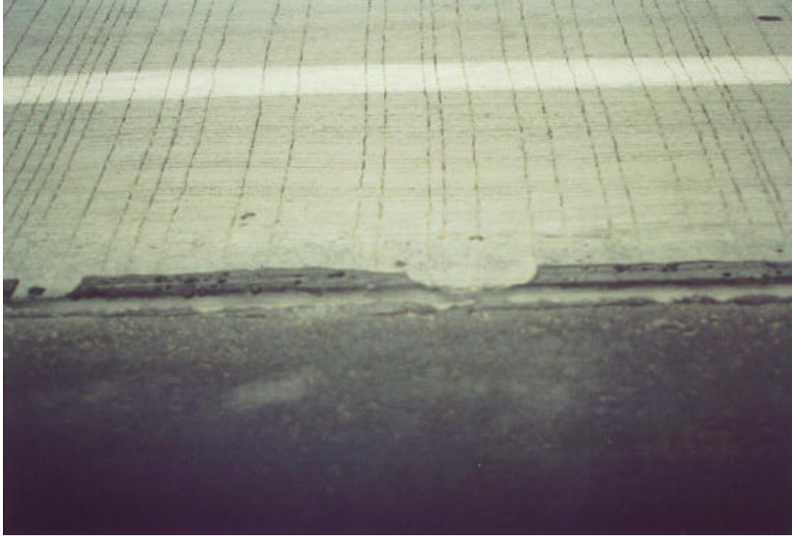
Figure 23. Snowplow damage to band-aid seal in daylighted ATPB test section (strategy 9).
