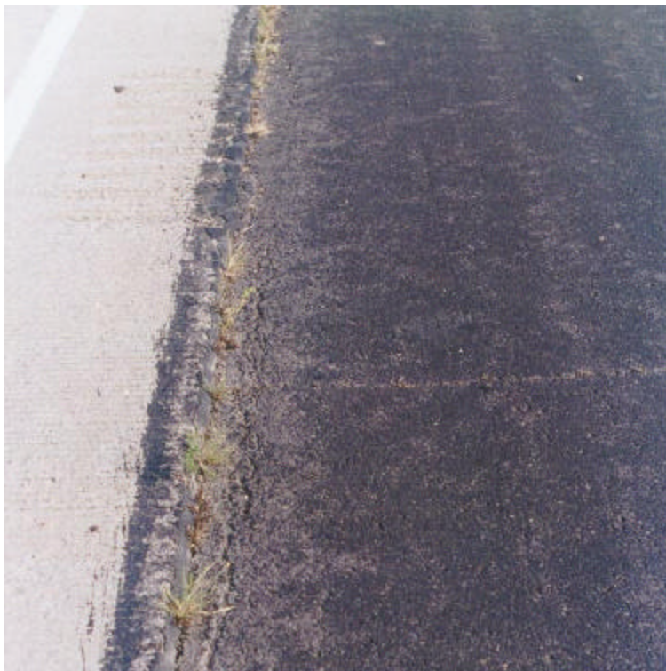
Figure 7. Joint seal failure and inside edge fatigue cracking on project 1 (US 81, Arlington).
