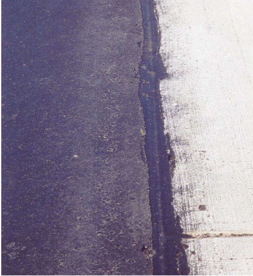
Figure 20. Longitudinal joint seal in recessed band-aid configuration.
