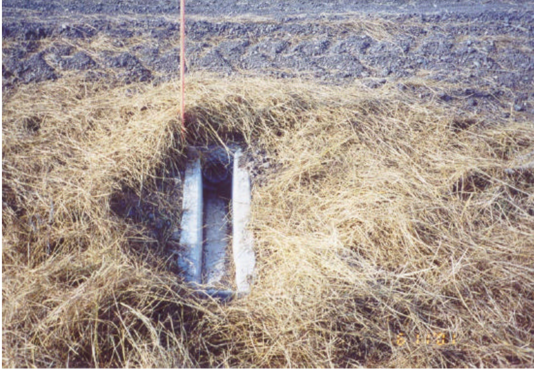
Figure 17. Longitudinal edgedrain outlet and headwall for shoulder strategy 4.
