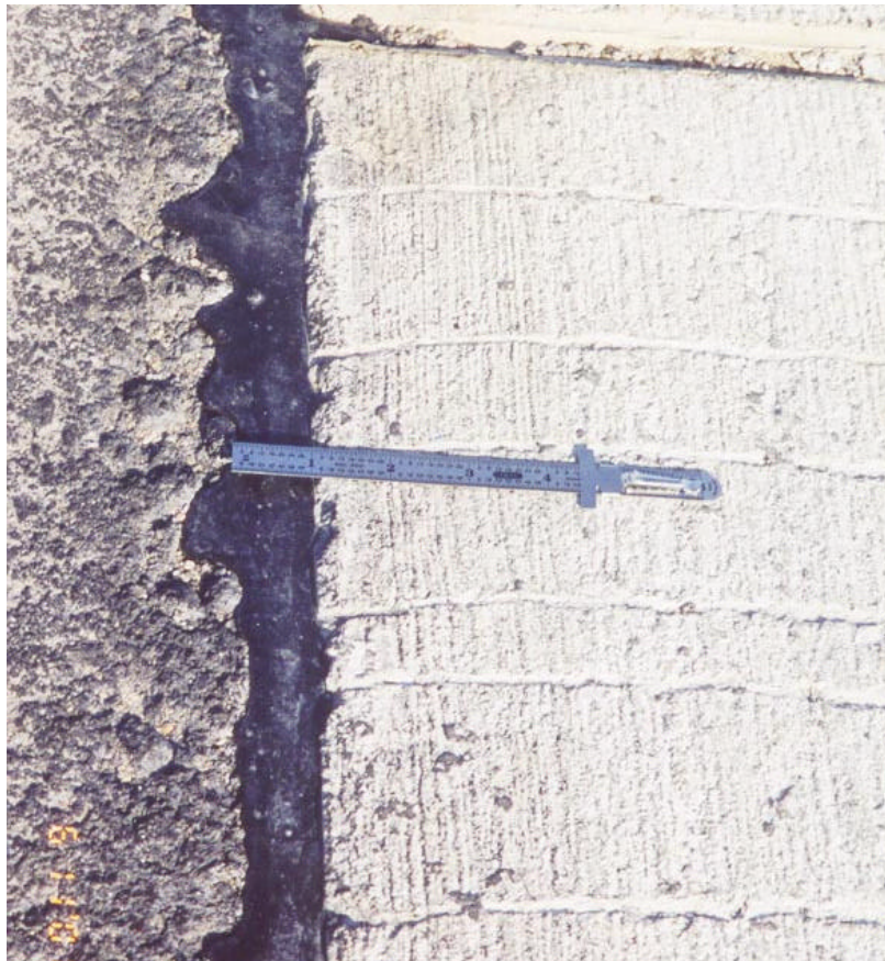
Figure 19. Longitudinal joint seal in standard reservoir-and-flush configuration.
