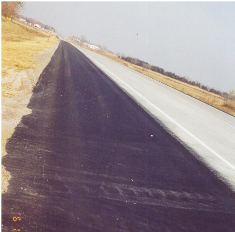
Figure 18. Completed AC-surfaced shoulder section.
