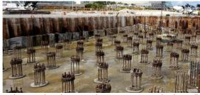
To be completed in 2027, the I-395 signature bridge will be 1,025ft long and span over NE Second Avenue and Biscayne Boulevard. The center pier construction will include 128 piles (3 ft in diameter with 27-in cages and extend approximately 120 ft below existing grade) as captured here in this image.
