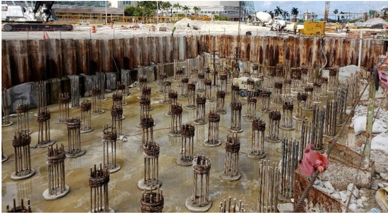
Figure 2.17 I-395 signature bridge center pier construction
