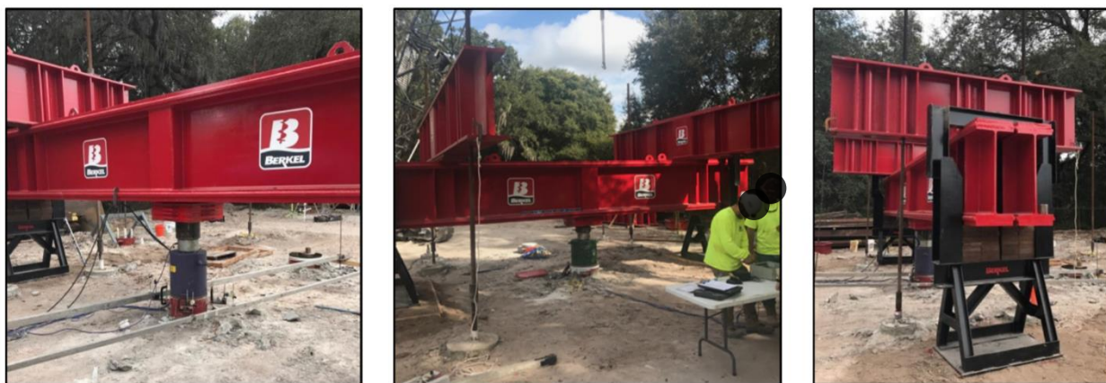
Figure 2.11 DFI pilot study compressive load test setup (Marinucci & NeSmith., 2017)
