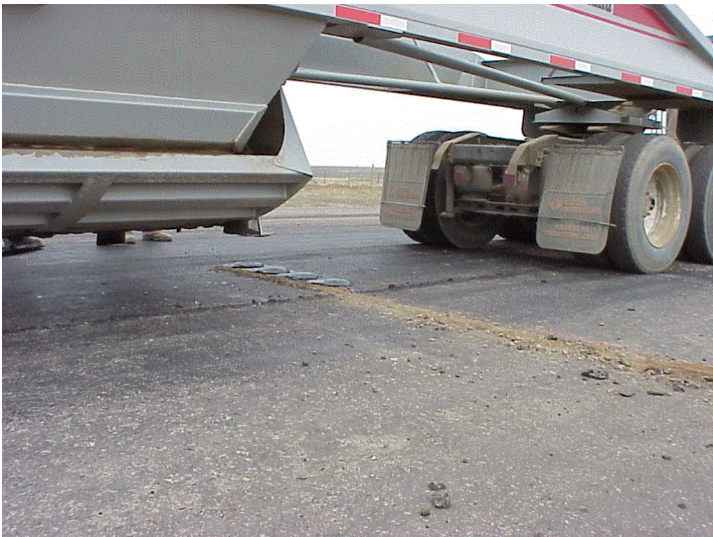
Figure 16: Strain Gauges Covered with HMA Mix and Being Overlaid
