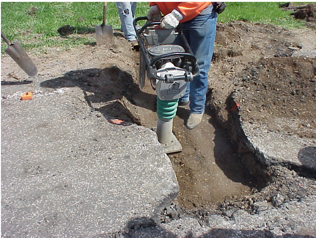
Figure 18: Base Materials Being Compacted on Top of the Pressure Cell
