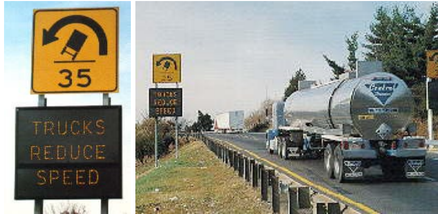
Figure 1. A speeding truck activates the sign
