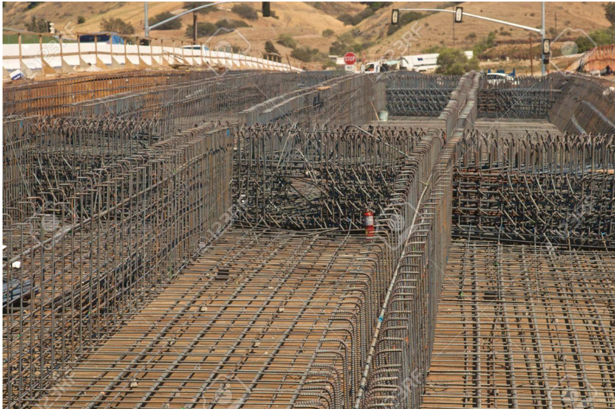
Figure 42 Example of a rebar array
