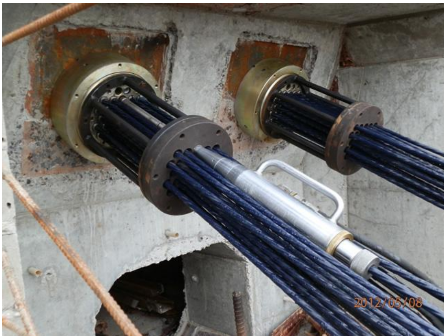
Figure 45 Example of an anchor
