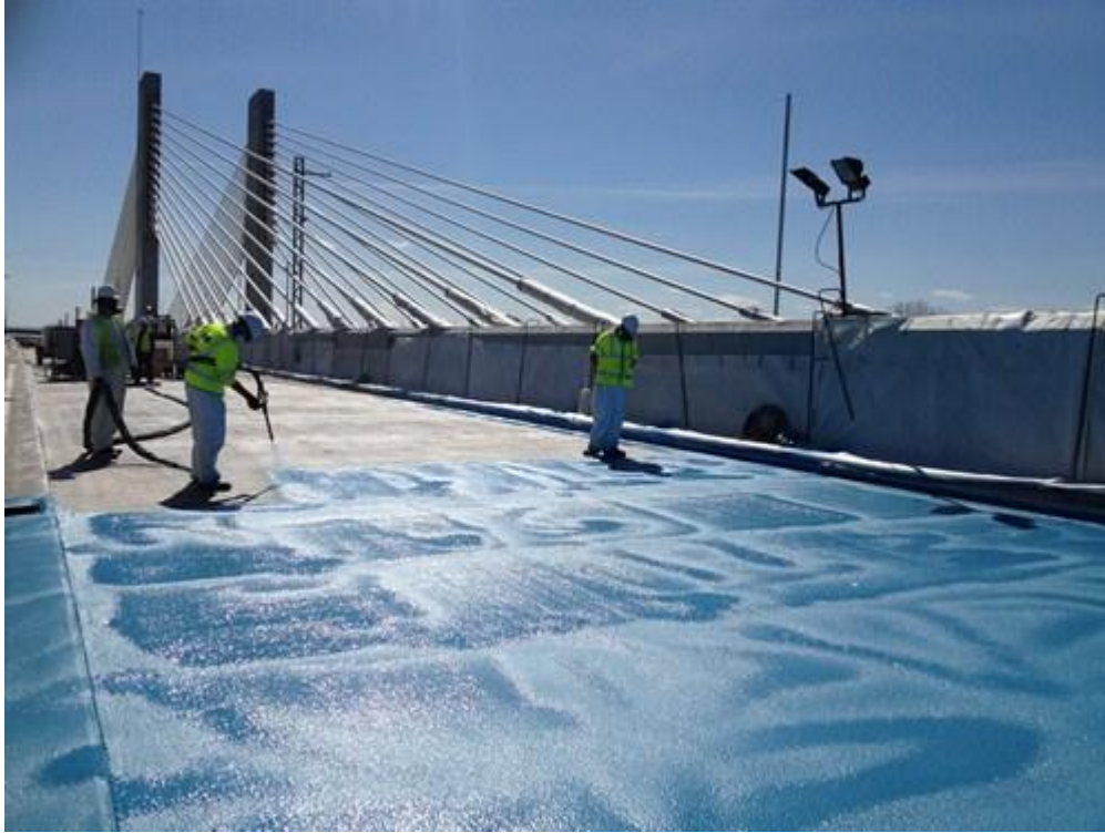
Figure 32 Example of a waterproofing membrane
