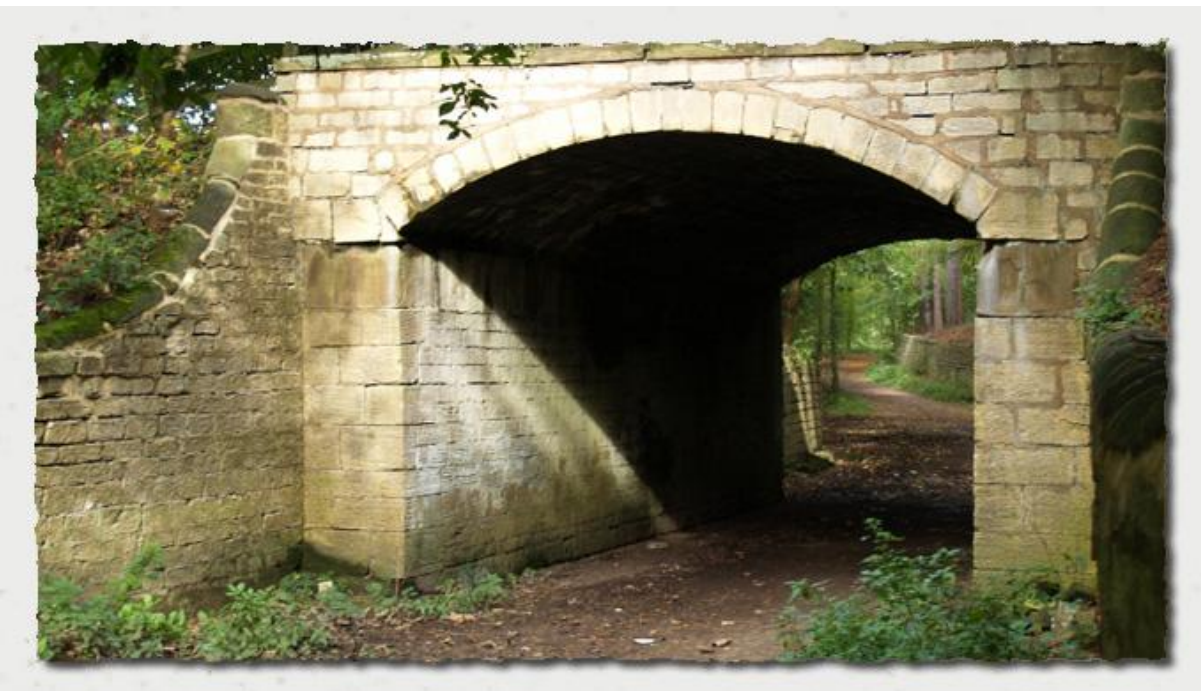
Figure 13 Example of a springer
