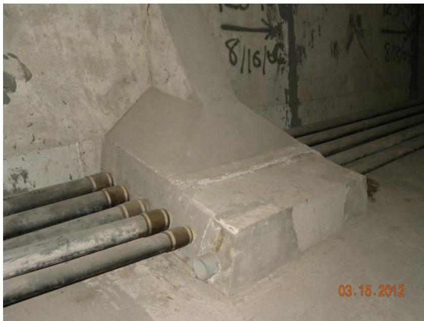
Figure 49 Example of a deviator
