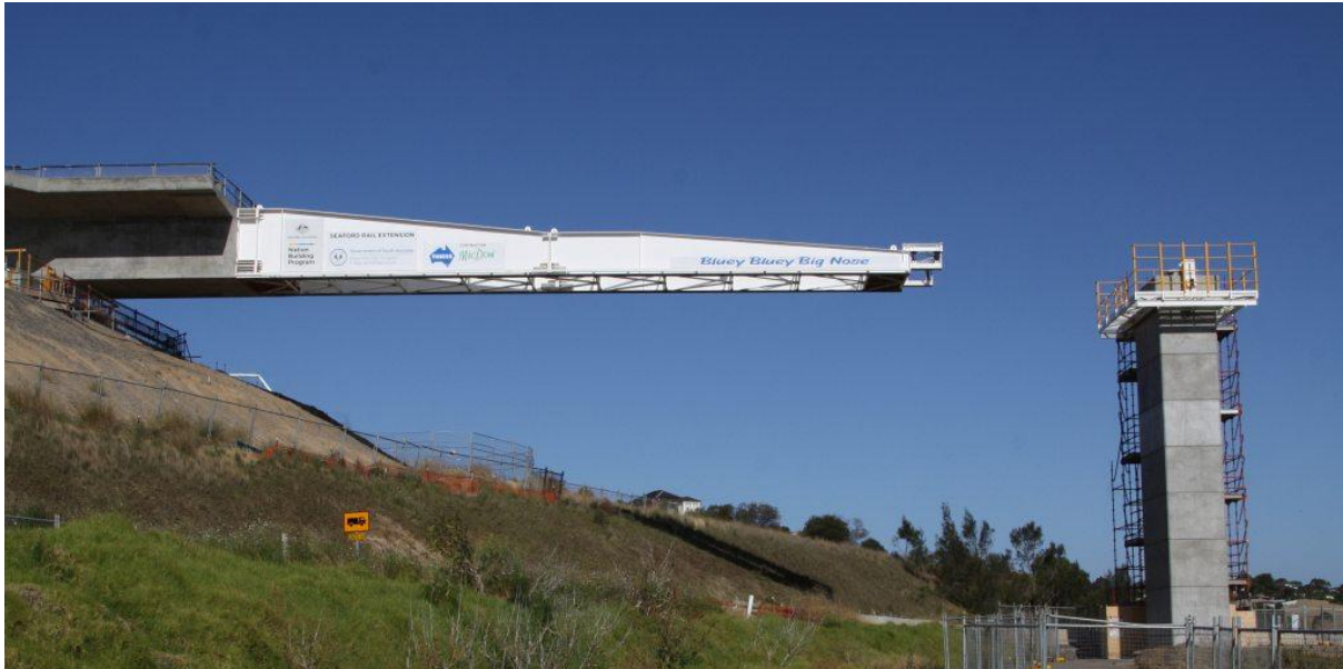
Figure 58 Example of a Launching nose
