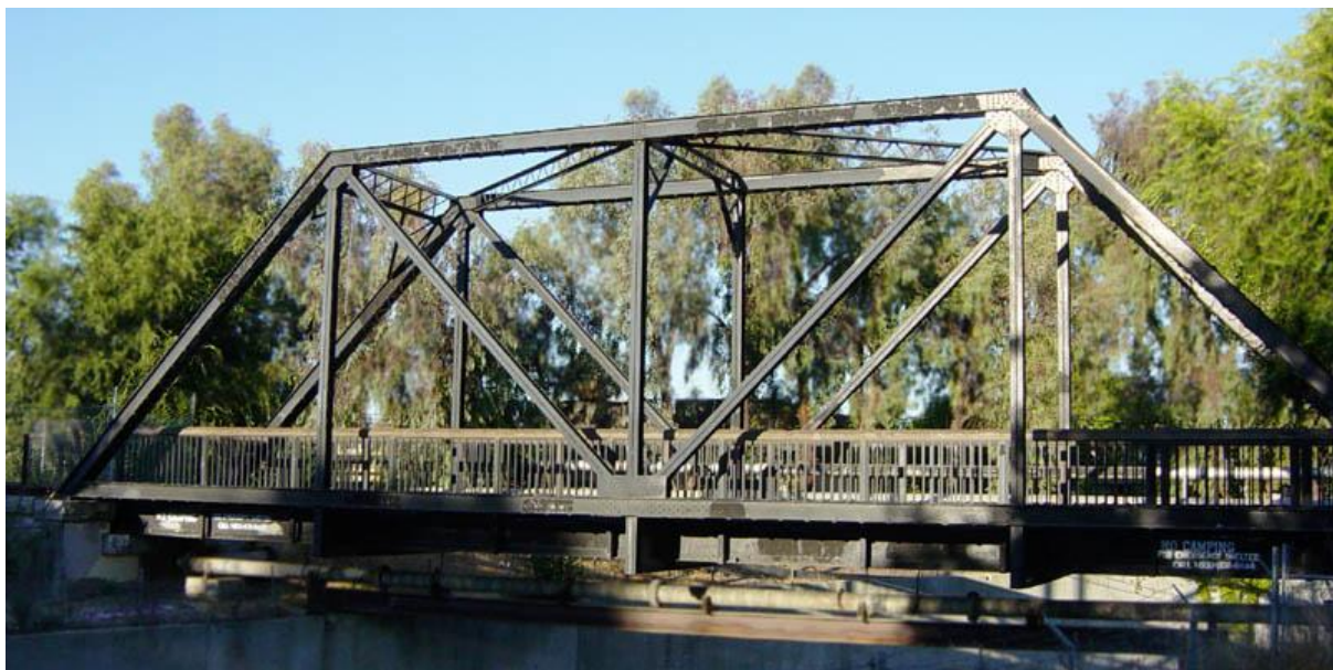
Figure 24 Example of a truss
