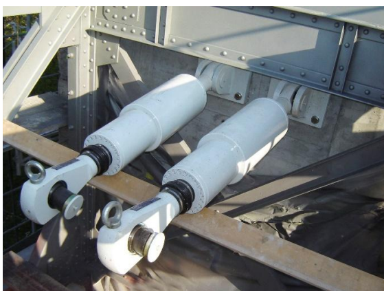
Figure 40 Example of a shock absorber
