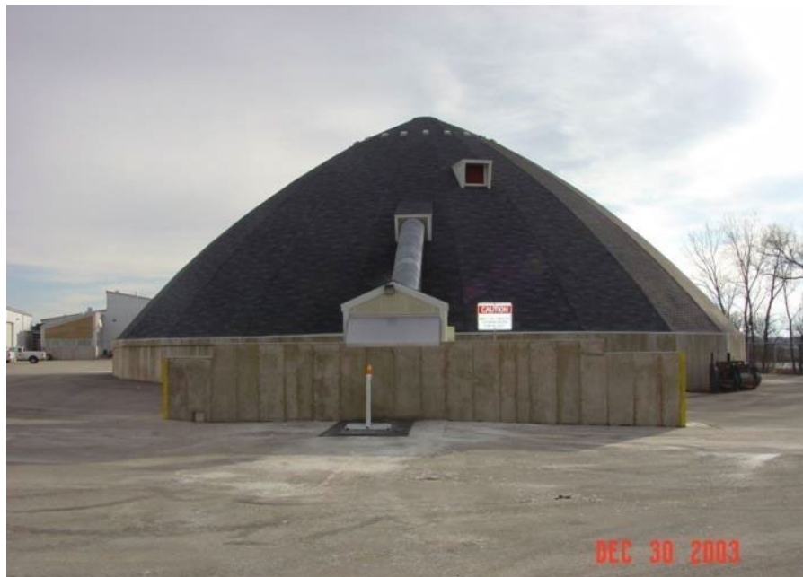
Figure 1 A Pit Type of Conveyor System for Loading Salt into Storage
