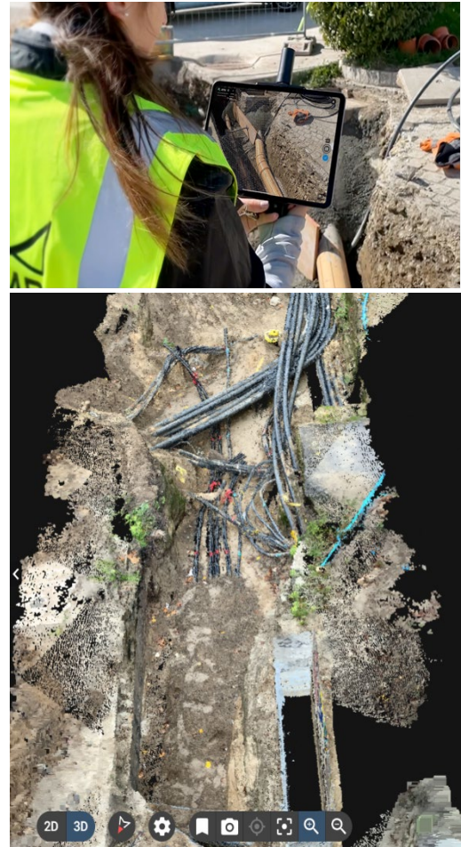
Figure 7. Pix4D is easy to deploy and readily provides spatially accurate, high resolution digital as-built positional and geometric data of open trench and surface utility installations.
