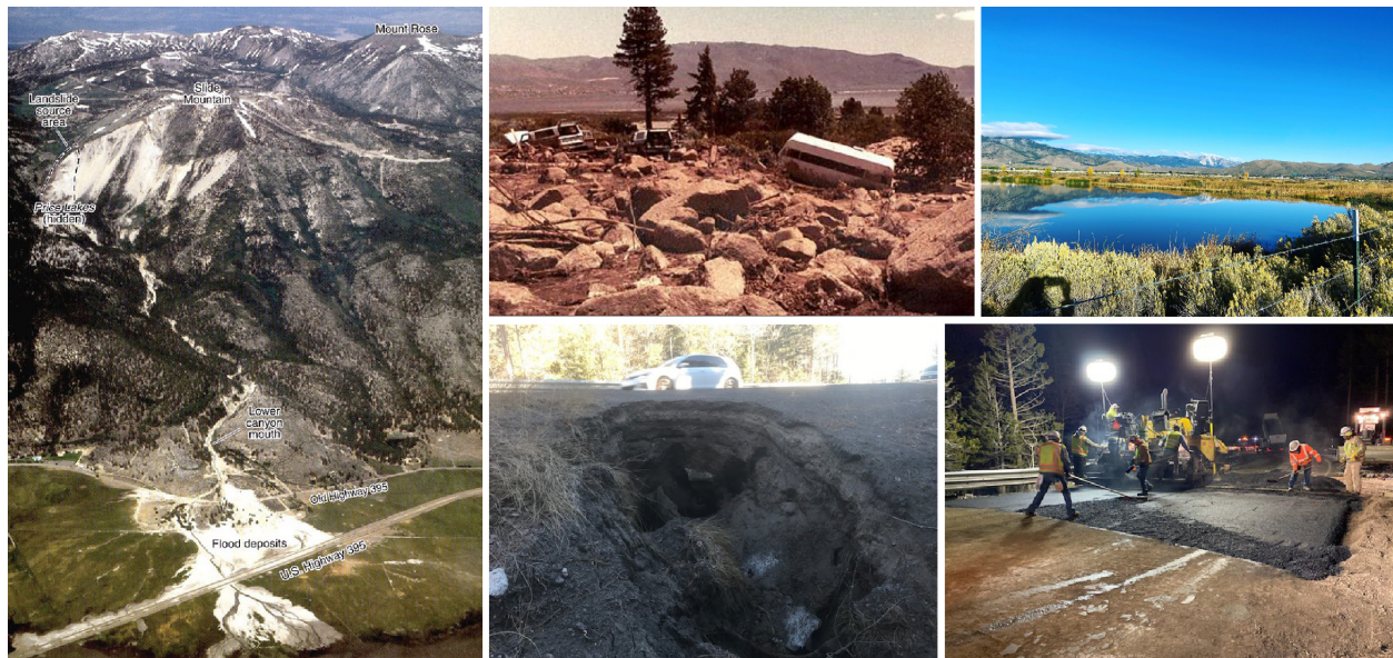
Figure 1: Examples of cool season flood impacts on Nevada roads. Clockwise from left: Snowmelt or extreme rainfall on Slide Mountain can produce debris flows that impact NV-580; Flood deposits on NV-580 following the May 1983 flood; The Carson City Wash mitigates flood impacts; NDOT workers repair a damaged culvert on NV-431; Erosion from extreme runoff damaged NV-431.
