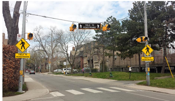
Figure 70. Enhanced amber beacon system in Toronto, Ontario, Canada – photo altered to show US MUTCD style signage including overhead blank-out sign. The unretouched image is shown in Figure 93. (Photo: City of Toronto)
