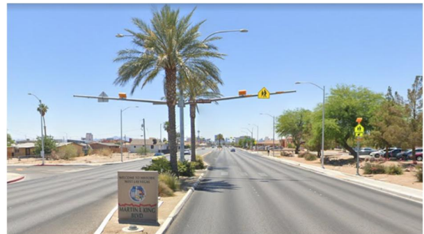
Figure 58. Rectangular rapid-flashing beacons (RRFBs) mounted on a mast arm, Martin Luther King Boulevard, West Las Vegas, NV (Image: Google Earth)
