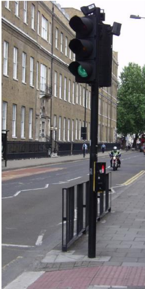
Figure 19 – Typical Puffin Crossing and Near-side Pedestrian Signal Module with Pushbutton
