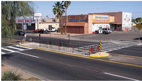
Figure 69. Fenced offset median refuge. Typically, the direction of the offset is arranged so that pedestrians will look toward traffic as they make the zigzag. (Photo: Arizona DOT)
