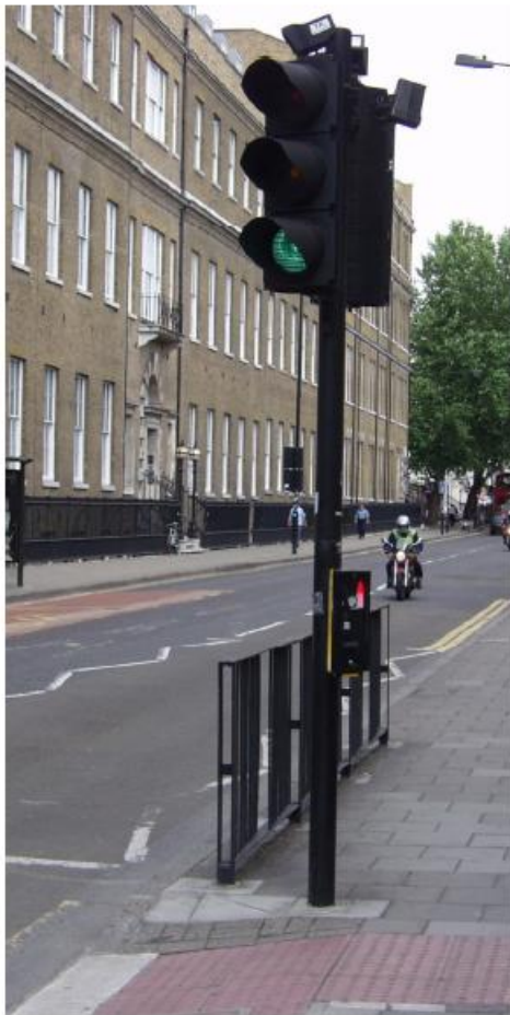
Figure 83. Typical puffin crossing and near-side pedestrian signal module with pushbutton
