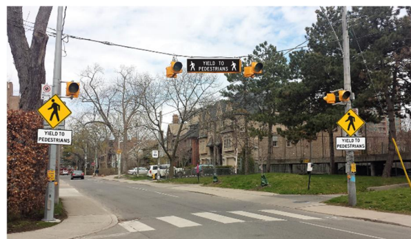
Figure 60. Enhanced amber beacon in Toronto, Ontario (digitally altered to show US MUTCD style signage). Base image: City of Toronto
