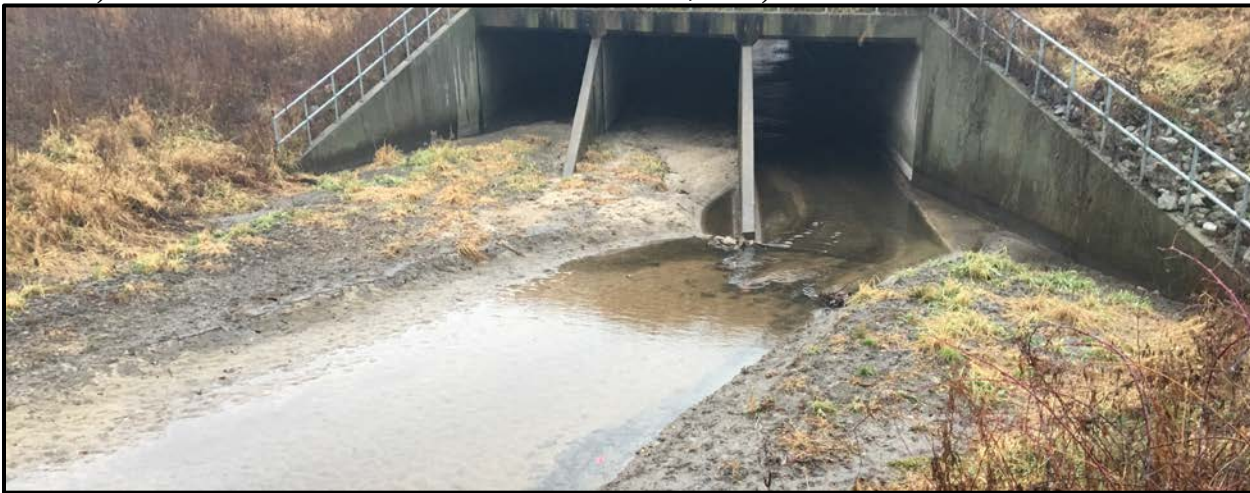
Figure 25. Development of the underwater sediment deposits in the upstream area of FHWA #364790 culvert site over the period of study. Note: the draining pipe shown in Figures 23 was used to empty the pooled area. The culvert downstream area is not shown as it remained submersed after pipe opening.
