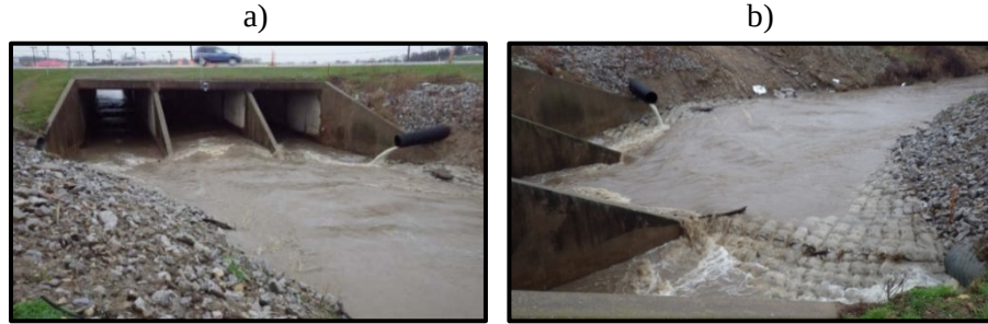
Figure 20. Documentation of the culvert performance during a storm event at FHWA #031711: a) and b) views of the flow through culvert during a storm; c) precipitation and stage hydrograph at the culvert location for the same storm.
