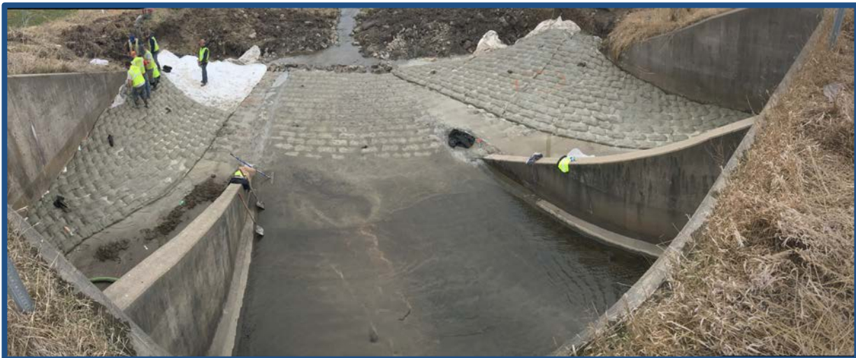
Figure 9. Aspects of the preparation and installation of the articulated block mat at FHWA #031711 site
