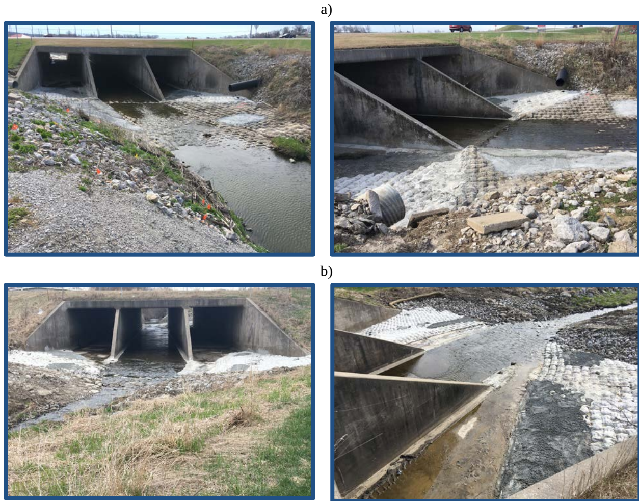
Figure 10. Views of the completed retrofitting at the FHWA #031711 culvert site: a) culvert inlet, b) culvert outlet
