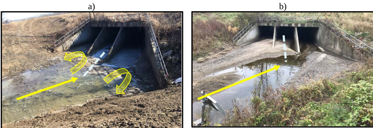
Figure 24. Preferential sedimentation of the sediment transport in the upstream area of the FHWA #364790 culvert during the first 12 months of culvert operation from the total cleanup: a) culvert after cleanup in February, 2018; b) sediment deposits in October, 2018. Yellow arrow: streamflow dominant direction; dotted white line: culvert orientation.
