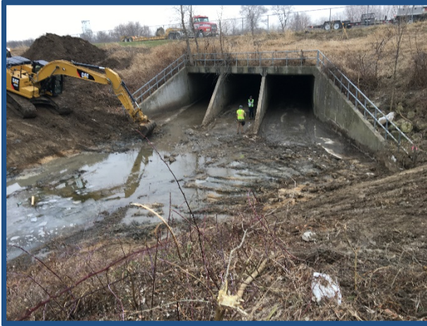
Culvert inlet at the end of cleanup
