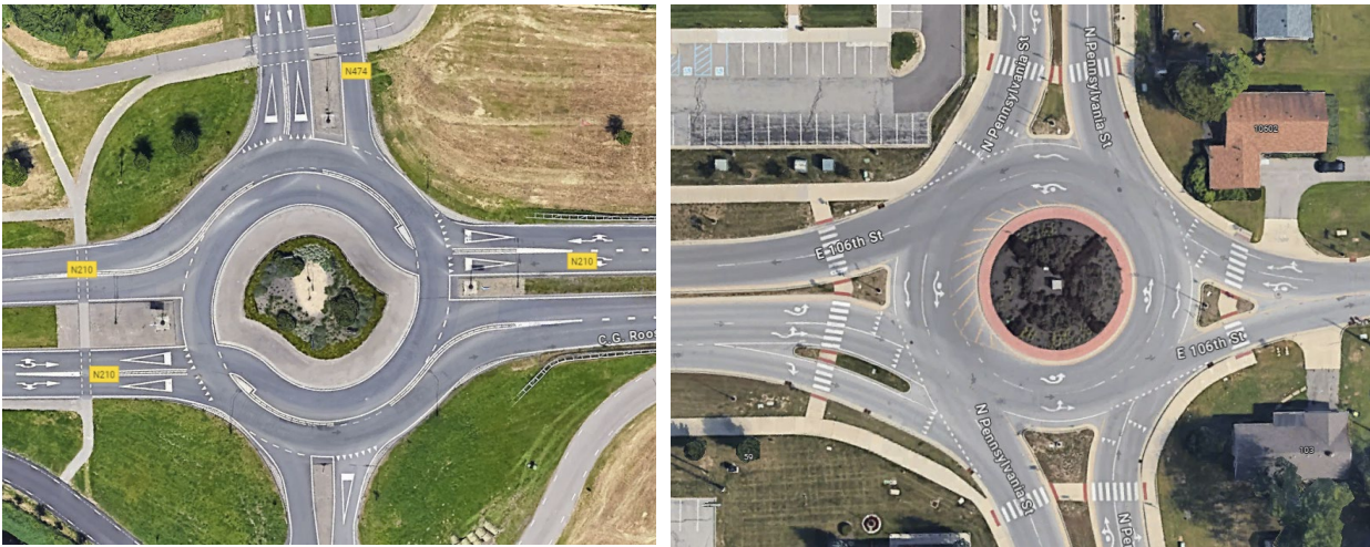
(a) Turbo roundabout, Netherland
