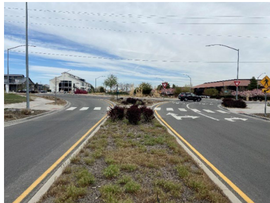
(b) North bound Approach-Kietzke Lane
