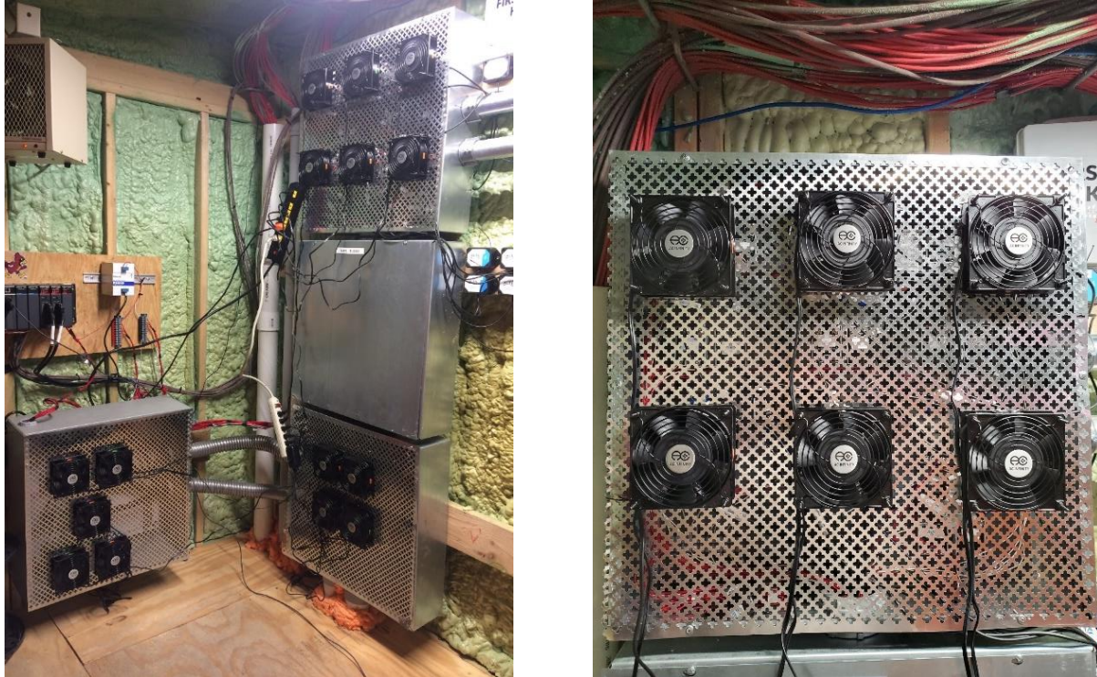
Figure 33. Cooling fans installed on the relays
