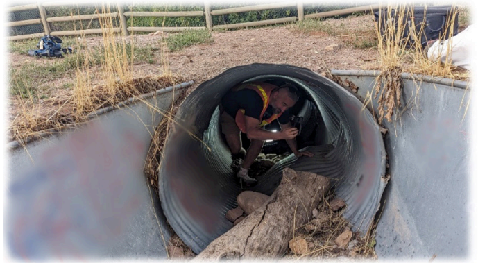
Figure 9. Photo. Example of PL data-collection process in the culvert.
