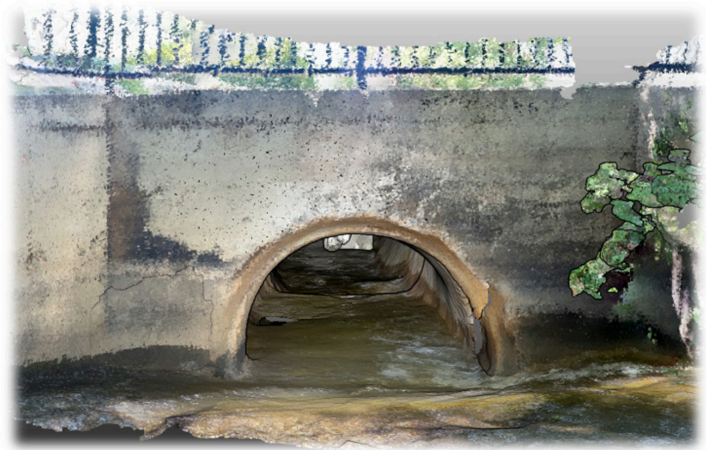
Figure 17. Screenshot. Example scan of the entrance of the Parley's Creek pavilion culvert.
