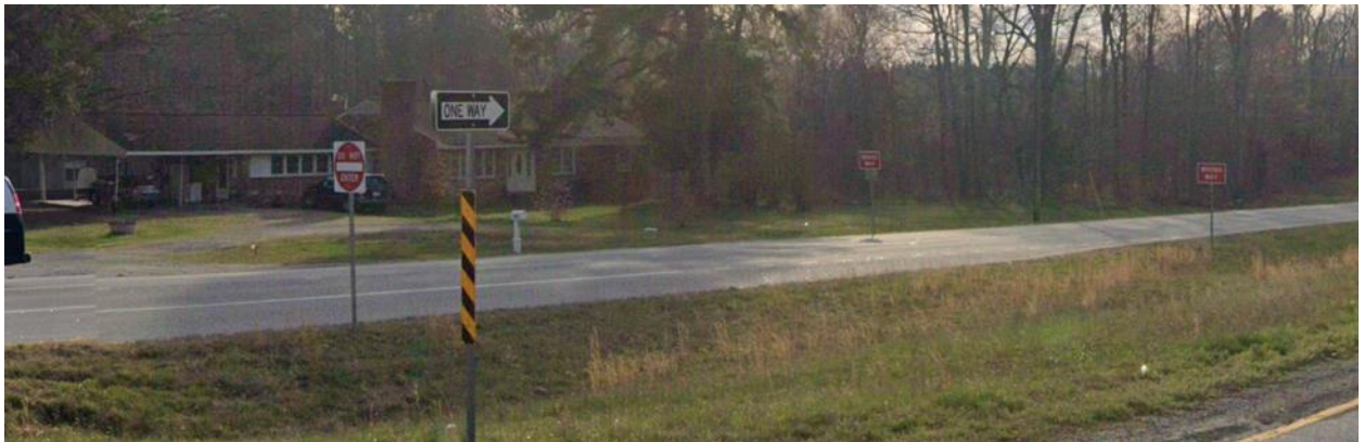
Figure 29. Route 58 Eastbound at the Reedy Creek Road Intersection Showing DO NOT ENTER and Dual Mounted WRONG WAY Signs (Google Street View, March 2023)
