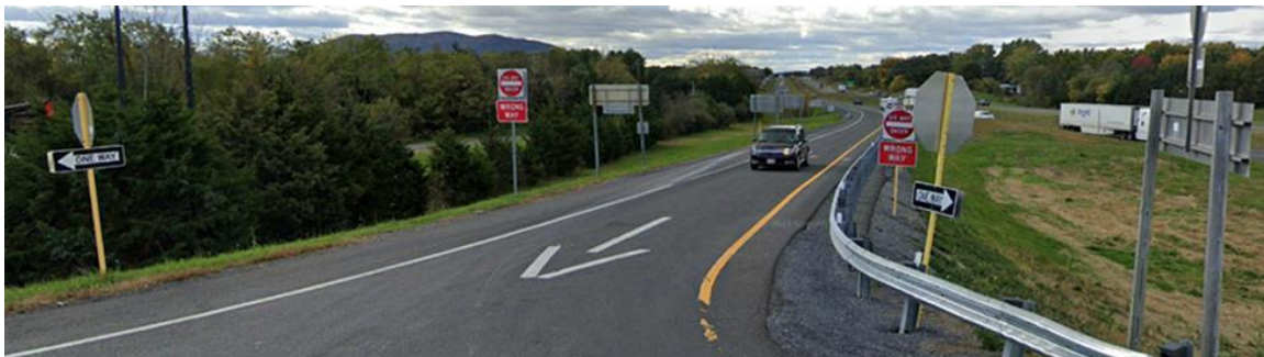
Figure 32. DO NOT ENTER and WRONG WAY Signs, Dual Mounted ONE WAY Signs, and Wrong Way Arrow (Google Street View)
