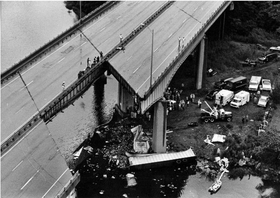
Figure 2.3: Collapse of the hanger span of the Mianus River bridge in Connecticut. Source: Hartford-Courant.
