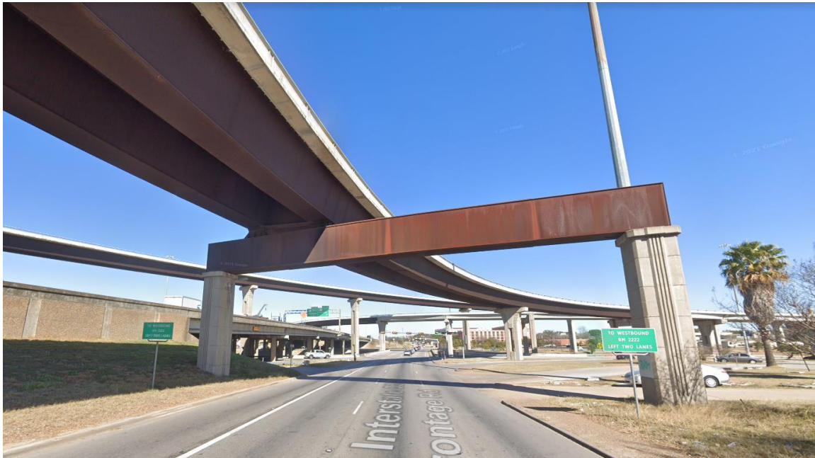
Figure 1.1: Steel box straddle cap supporting twin tub girders. Source: Google Maps.
