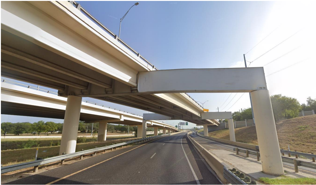
Figure 3.2: Non-integral steel box straddle caps supporting longitudinal prestressed concrete girders on South MoPac Expressway and West Cesar Chavez Street, Austin, TX. Source: Google Maps.
