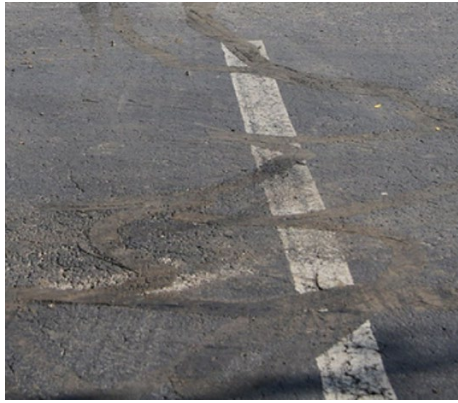
Figure 33. Photo. Crack Sealing on Pavement Marking.
