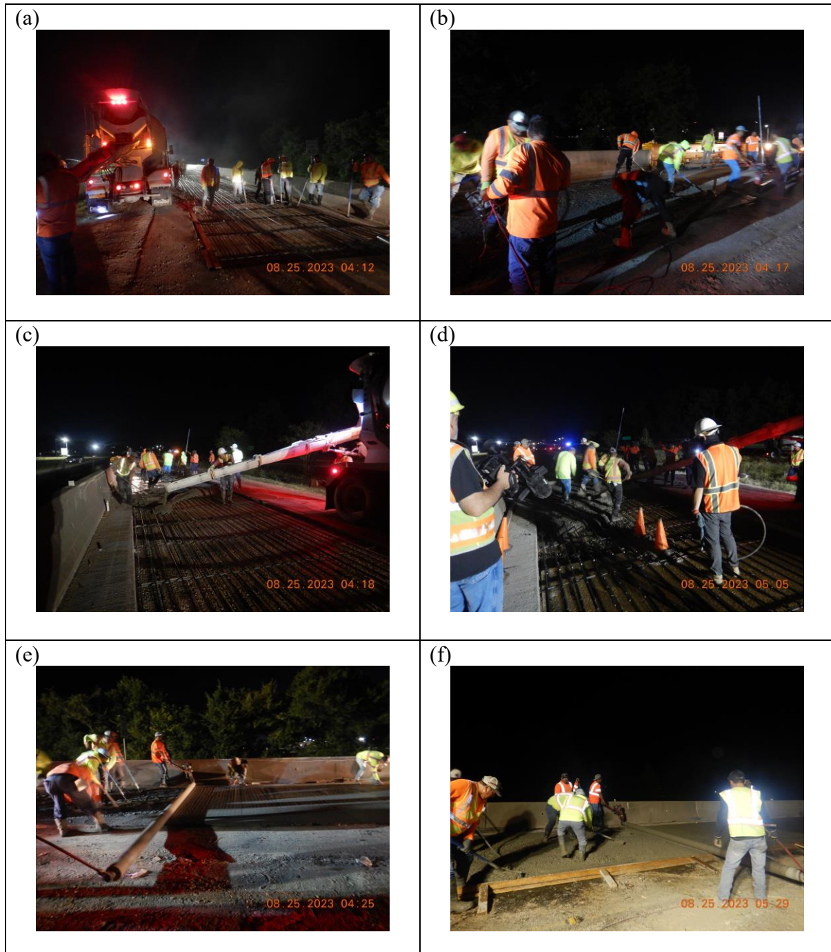
Figure 48 Concrete placement and consolidation on inside lane
