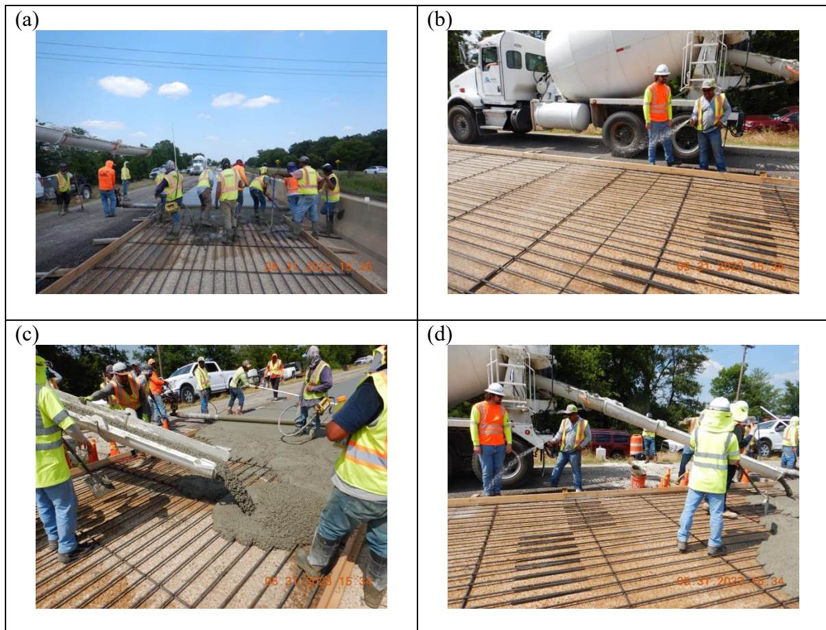
Figure 47 Surface condition during concrete placement
