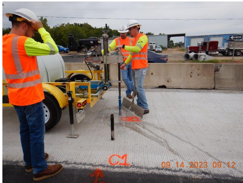
Figure 79 Trailer mounted coring machine used for Inside lane
