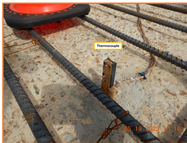
Figure 35 Field gauge installation at section 2
