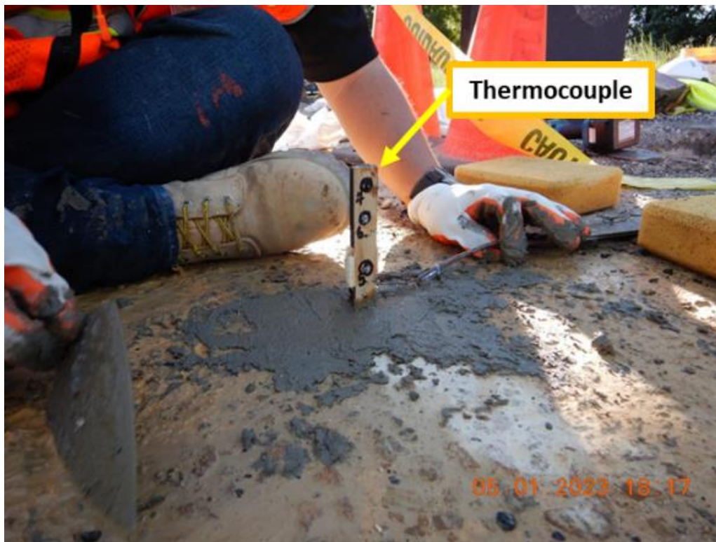
Figure 30 Typical Installation of Thermocouple
