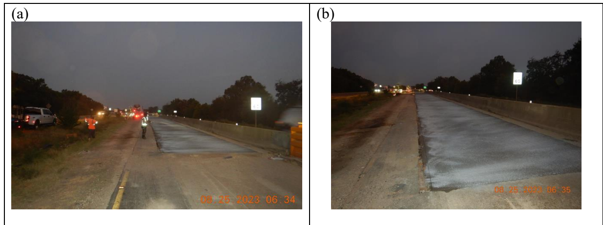
Figure 50 Curing compound application after concrete placement
