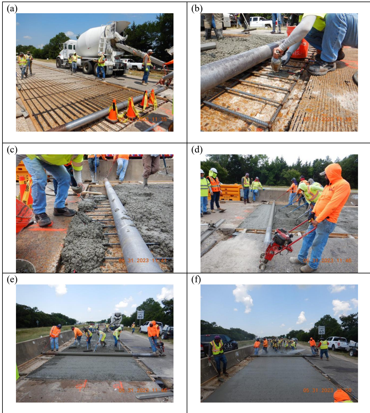
Figure 43 Concrete placement and consolidation on outside lane.
