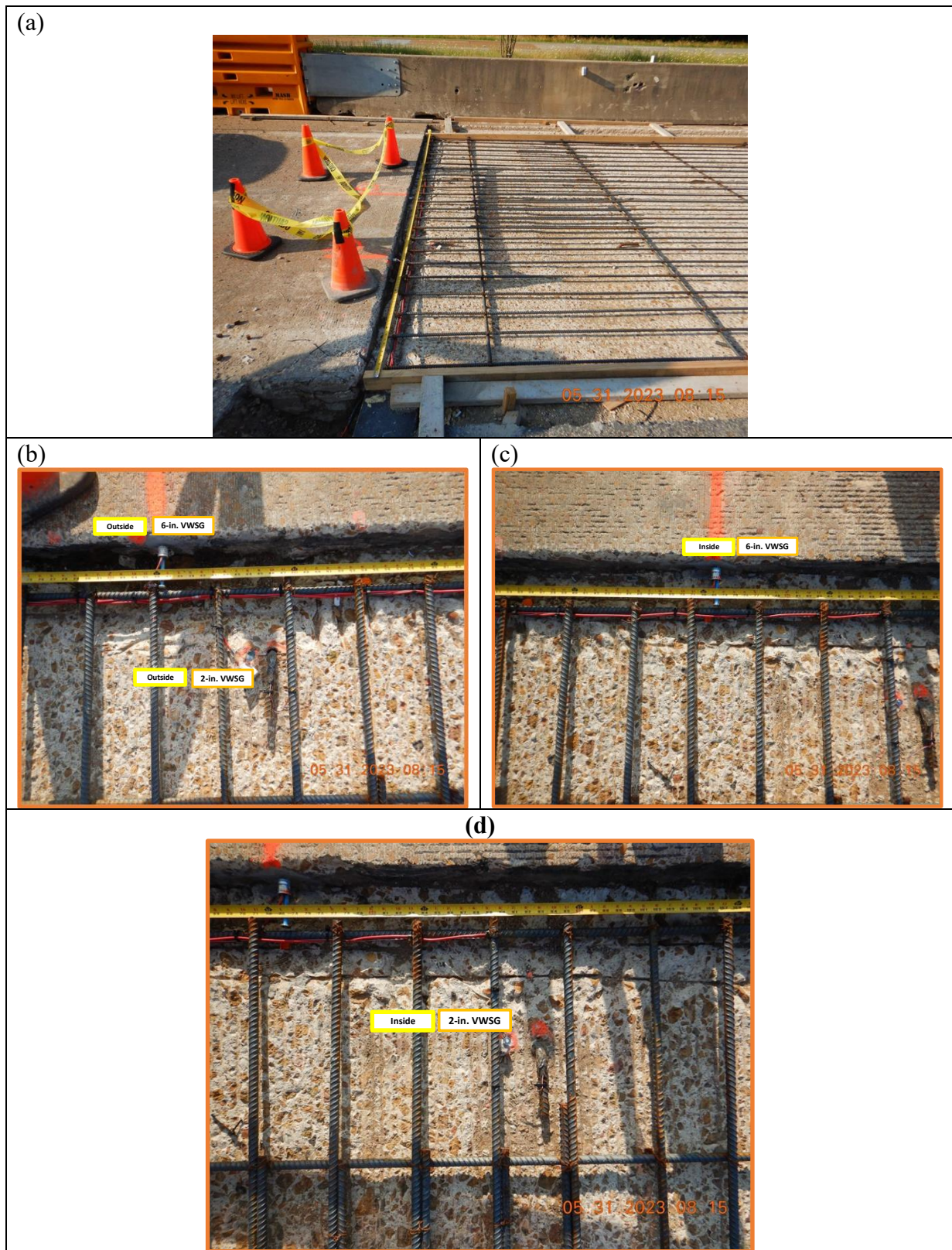
Figure 34 Field gauge installation at section 1
