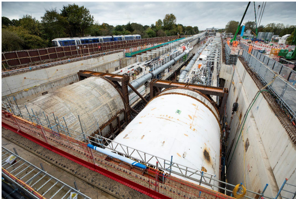
Figure 5-8. Sacrificial temporary rings used to launch TBM can be used for on-site load testing to failure.
