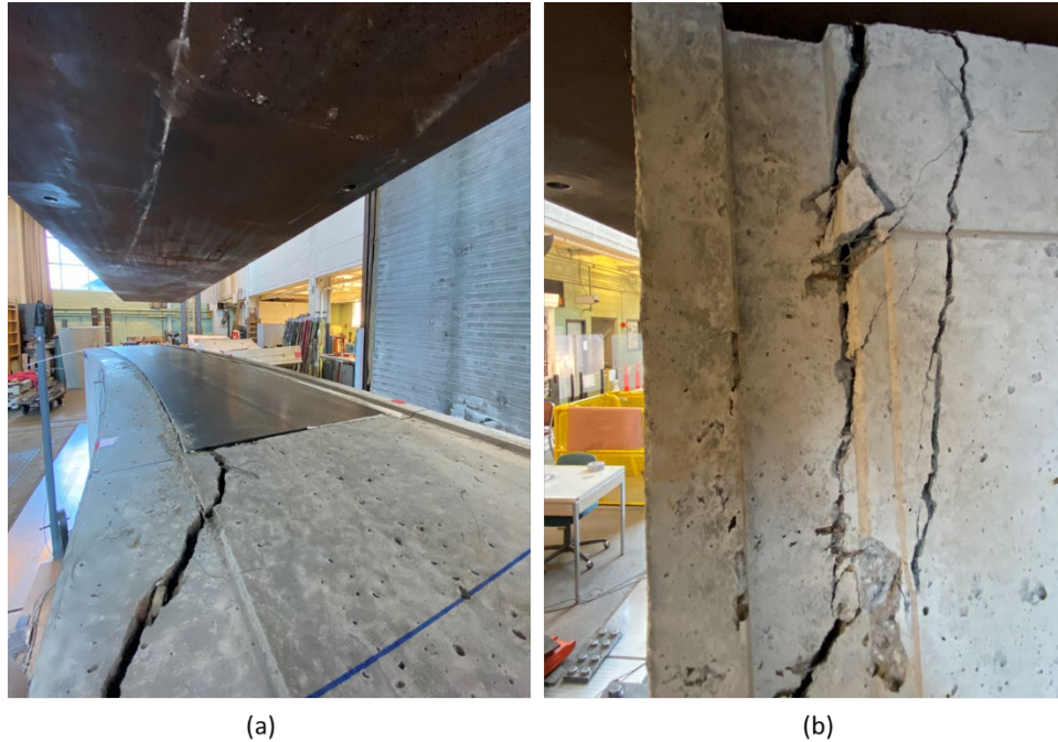
Figure 2-10. View after radial bursting stress failure of SFRC segment: (a) Leading edge where radial bursting stress induced cracking is clear; (b) side of the segment where radial bursting stresses (along thickness direction) exceeded the tensile capacity of the SFRC.
