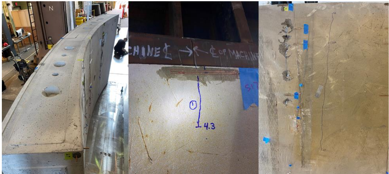
Figure B6-7: Damage of segment after test 6 completion.
