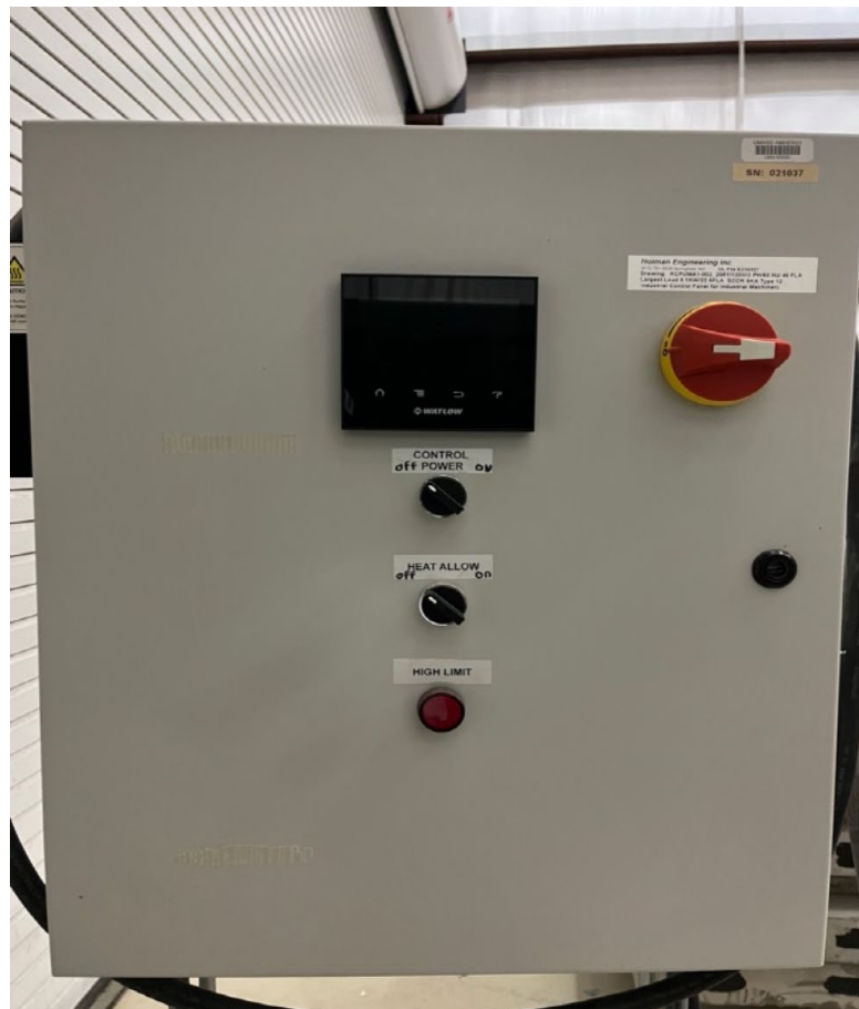
Figure 2-3: F4T terminal attached to the heaters
