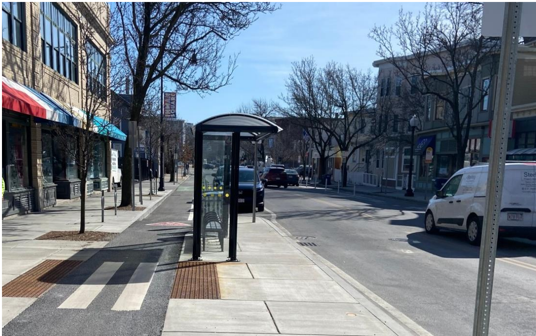
Figure 3.22: Floating bus stop with tactile pavement (Hampshire St. at Cambridge St., Cambridge, MA)
