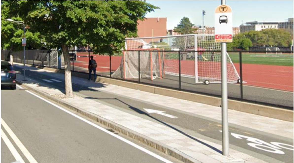
Figure 3.5: Partial-width platform bus stop (Vassar St opp. Pacific St Extension, Cambridge, MA)
