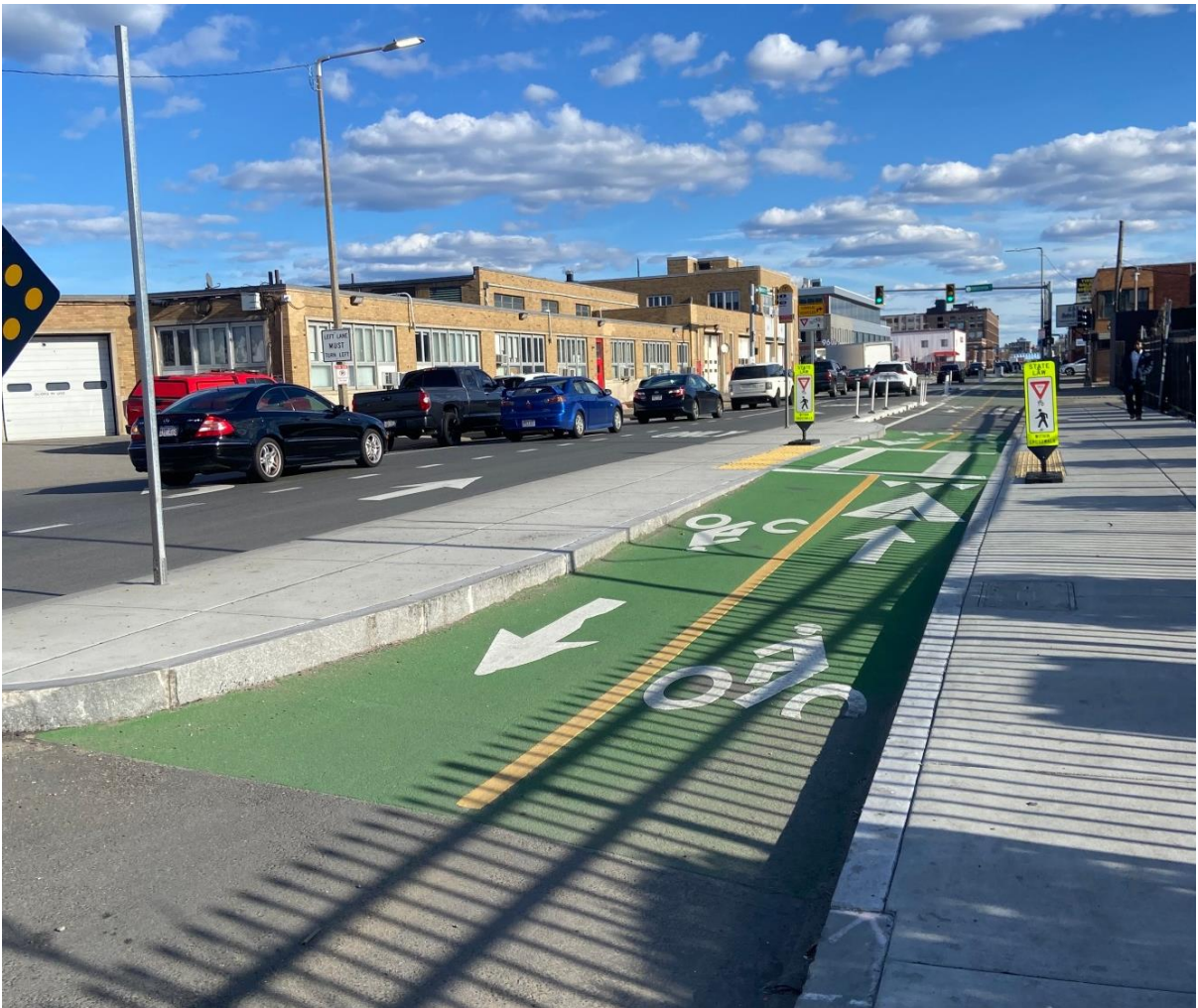
Figure 3.9 Vertical curve along the adjacent bike lane (Massachusetts Ave at Island St, Boston, MA)
