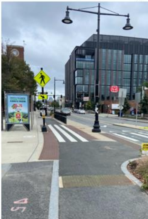
(b) Downstream end view
