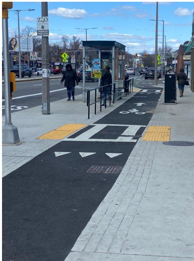
Figure 3.20: Floating bus stop with fencing (Morton St at Blue Hill Ave, Boston, MA)
