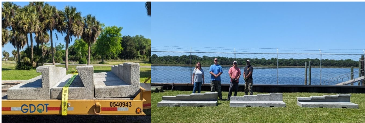
Figure 5. Photo. Curb installation. Left: The three types of reverse curb designs used in the experiment. Right: D5 Maintenance Crew with PI Andrews at the Brunswick test site when the curbs were being delivered.
