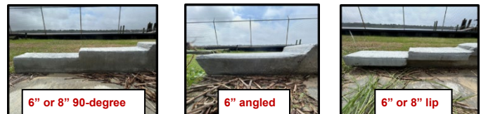
Figure 24. Photo. Recommendations. Recommendations for curb heights and angles relative to the degree of likelihood of trespass and maintenance burden based on the research results.
