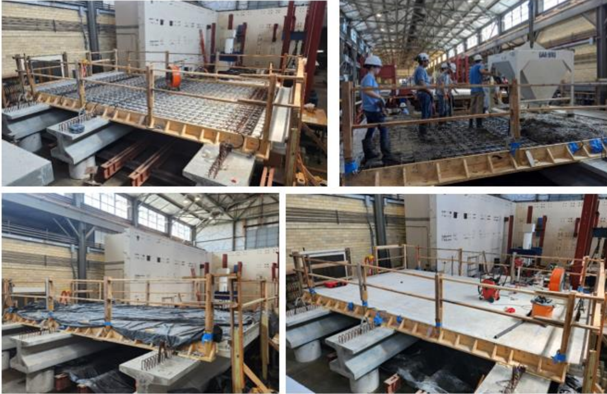
Figure 4-15: Casting and finished WTPD deck specimen
