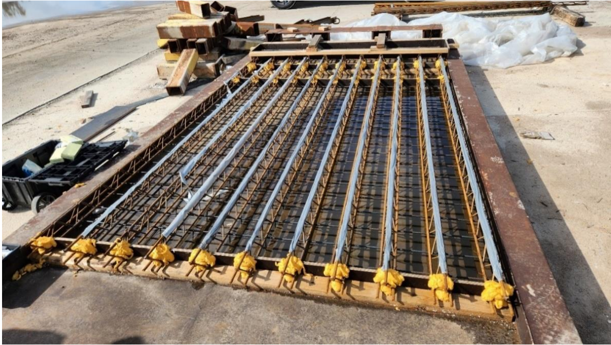
Figure 4-6: Trusses and Lumber Formwork in Standard Precast Bed
