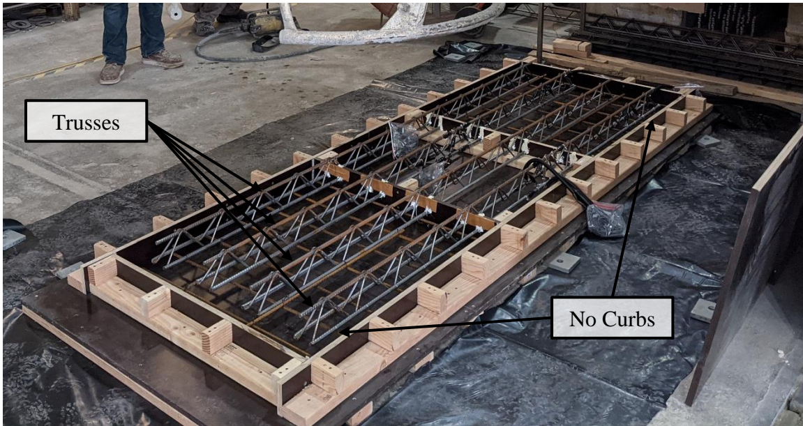
Figure 5-4: Construction of Formwork for Testing Specimen
