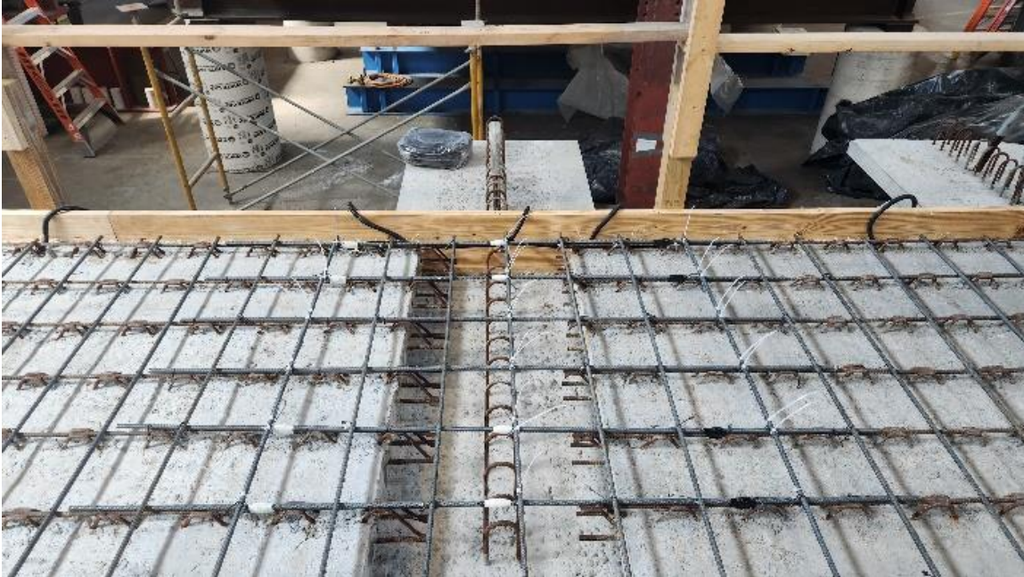
Figure 4-14: Reinforcement and lap-splice
