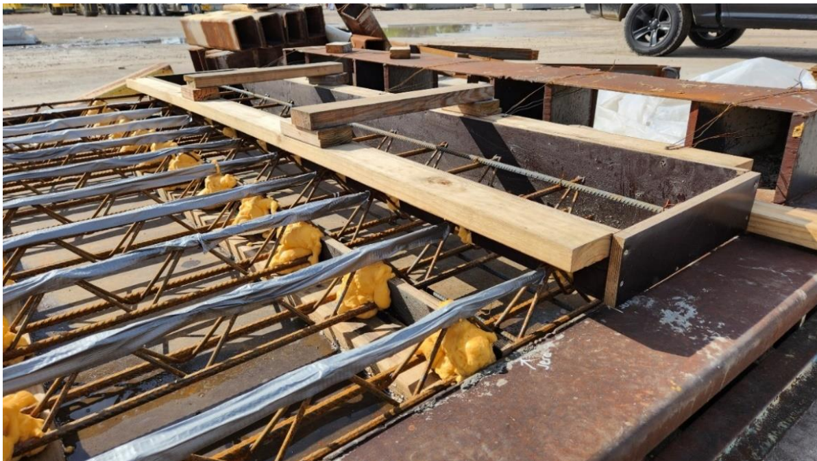
Figure 4-7: Full-Depth Curb Lumber Formwork
