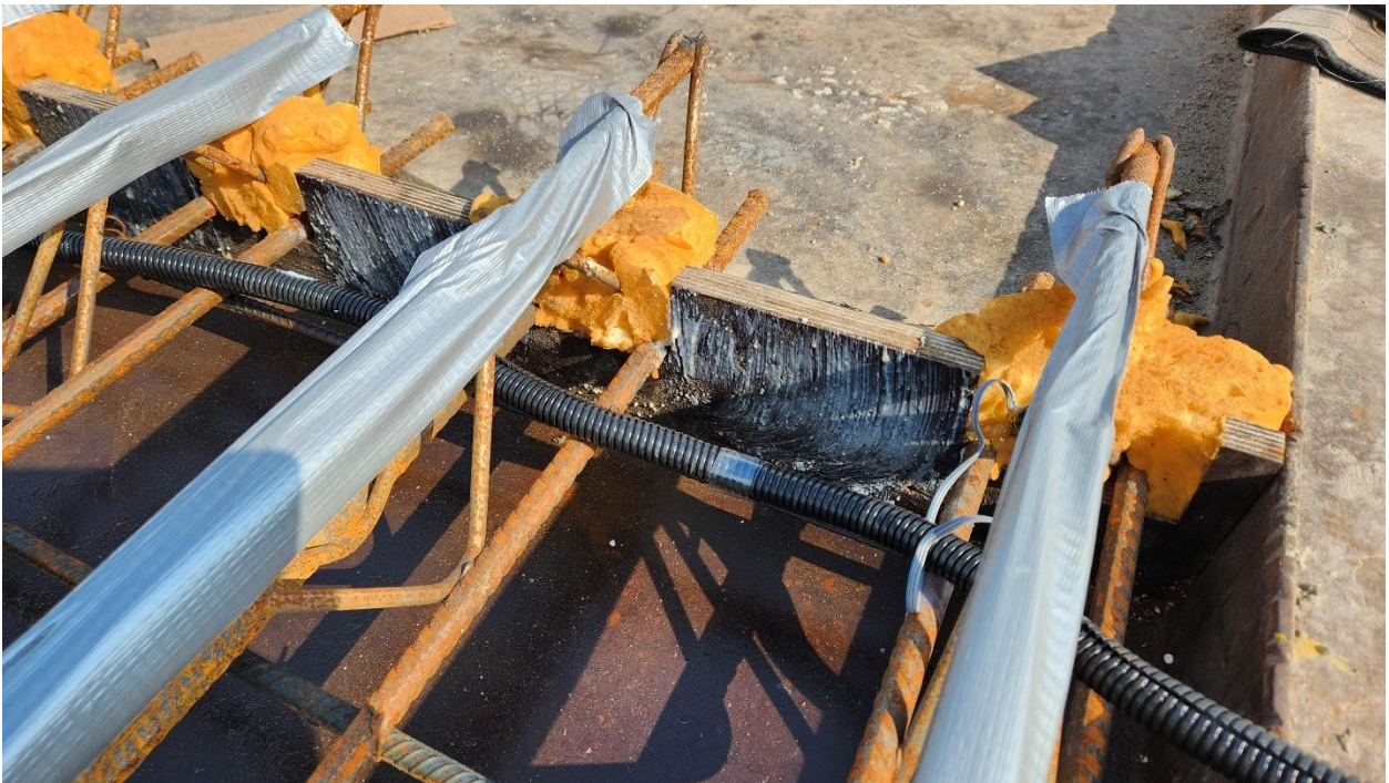
Figure 6-4: Lumber end form and spray foam
