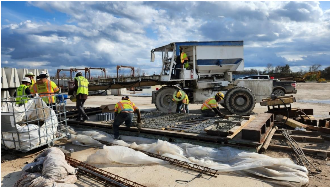
Figure 4-8: Panel pair concrete pouring
