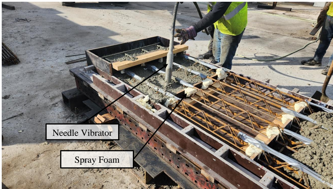
Figure 5-6: Precast Panel Cast
