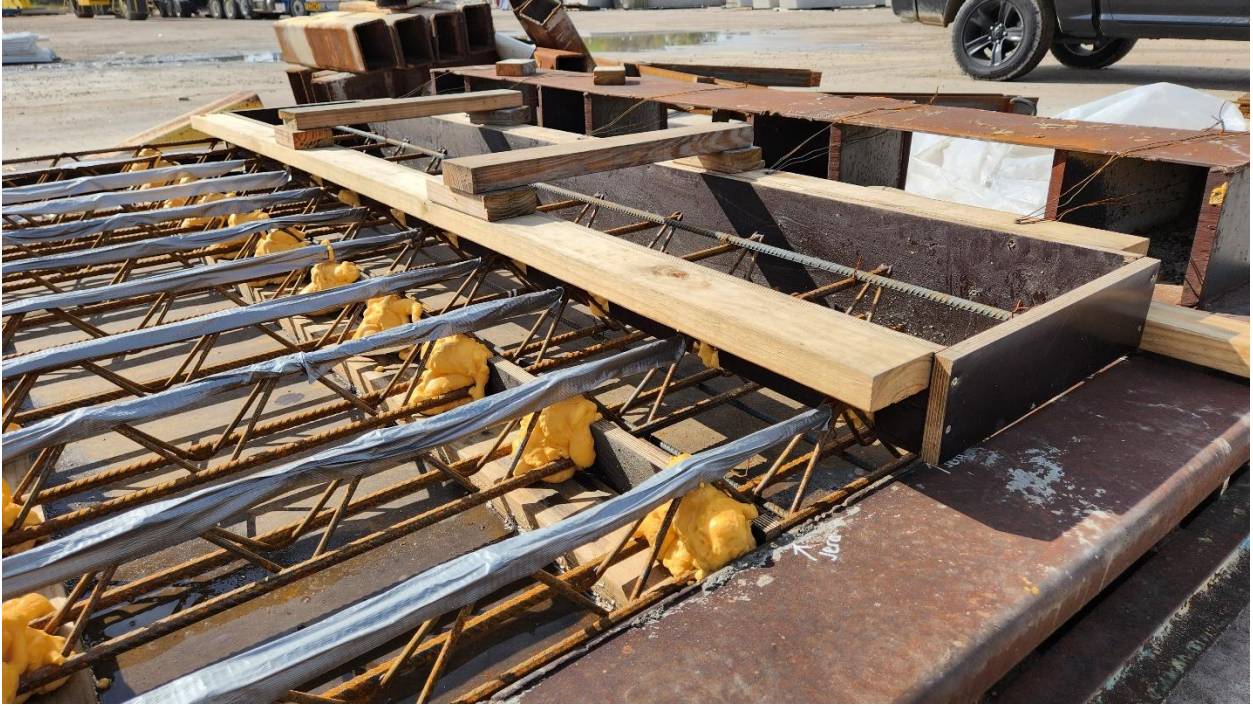
Figure 6-3: Lumber overhang curb formwork
