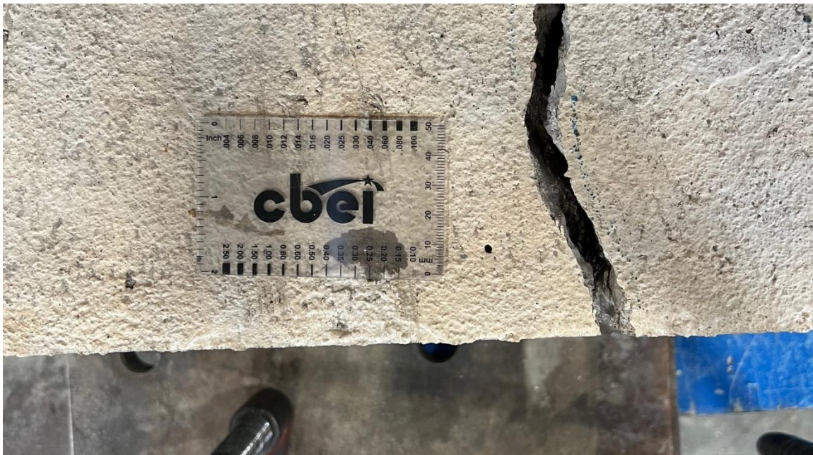
Figure 5-33: Test 5 - Maximum Crack Width at End of Loading
