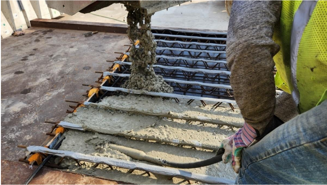
Figure 4-9: Panel pair concrete vibrating
