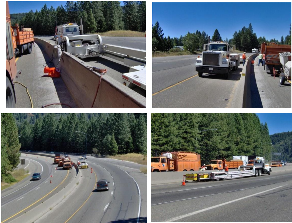
Figure 4.3: Median repair on a curved section of a highway (Courtesy of District 5).
