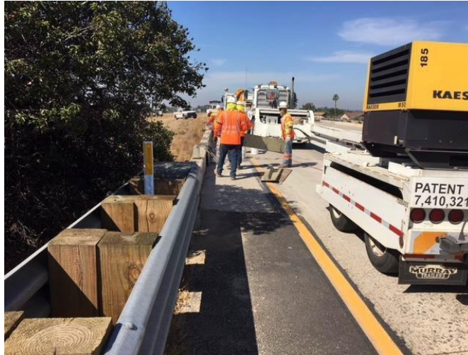
Figure 4.4: Guardrail repair (courtesy of District 11).
