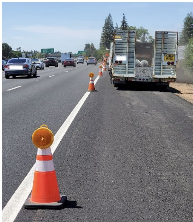
Figure 5.4 Deployment of Intellicone Lamps with Limited Space between Closure and Presence of Work Vehicles
