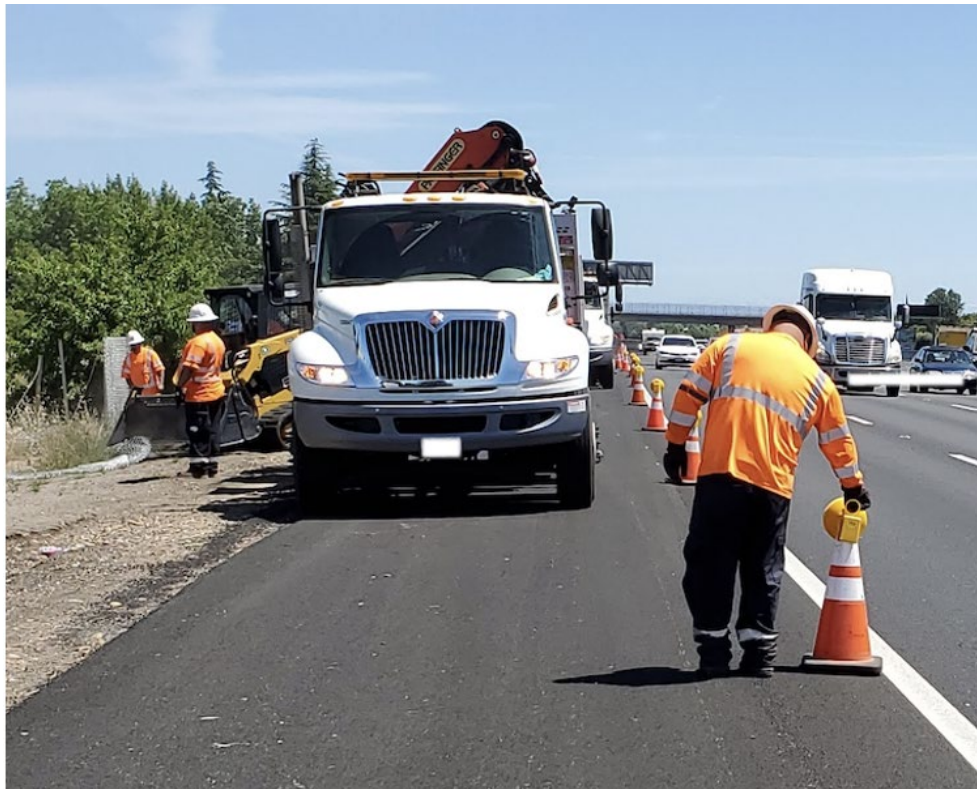
Figure 5.5 Deployment of Intellicone Lamps by Maintenance Worker
