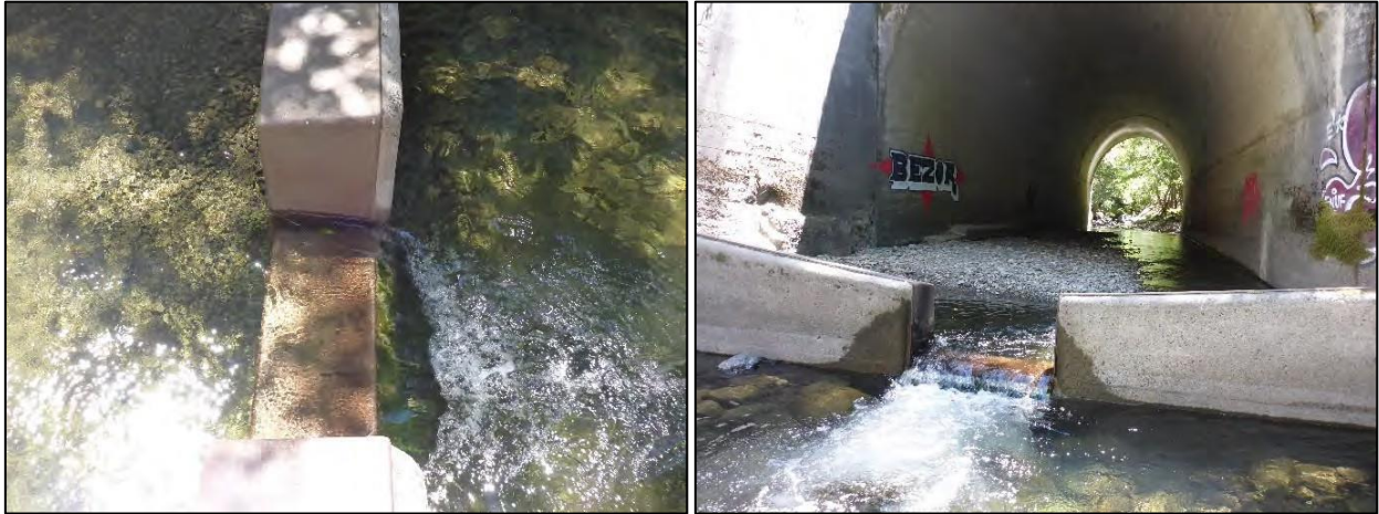
FIGURE 9-3. THE WEIR NOTCHES ON THE OUTLET FISH LADDER ARE BROAD, CREATING LOCALIZED SHALLOW, FAST FLOW. WEIR 1 SHOWN HERE HAD THE SHALLOWEST DEPTHS (0.45 FT ON THE US SIDE, 0.25 FT ON THE DS SIDE). AT SOME FLOWS THE NOTCH CONDITIONS MIGHT EXCEED FISH PASSAGE SWIMMING CRITERIA, ESPECIALLY FOR JUVENILE SALMONIDS. PHOTOS TAKEN JULY 17, 2019.
