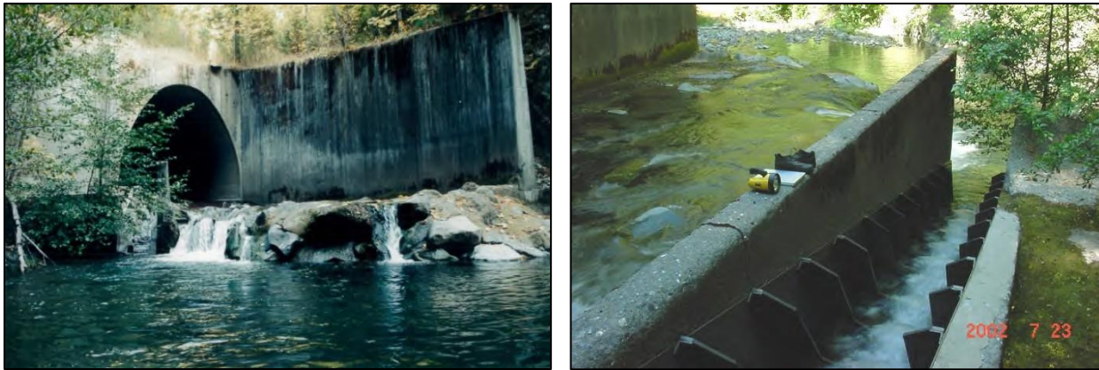
FIGURE 10-1. CEDAR CREEK CROSSING OUTLET AND FISH LADDER BEFORE THE 2017 MODIFICATIONS. PHOTO ON LEFT PROVIDED BY M. MOLINAR CALTRANS, PHOTO ON RIGHT BY M. LANG.
