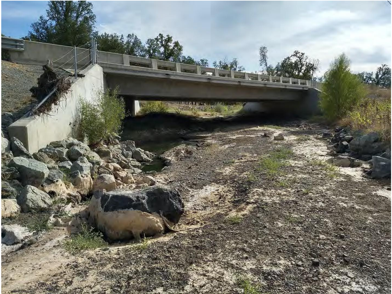
Figure 4. Lemm/Yank Creek Highway 299 bridge looking downstream. The creek channel is aligned with the thalweg along the left wingwall upstream, then crossing through the structure to the right wingwall downstream. High flow debris was captured on the fence above the left wingwall as it poured over the wall creating the scour hole in the foreground. Photo taken October 4, 2019.
