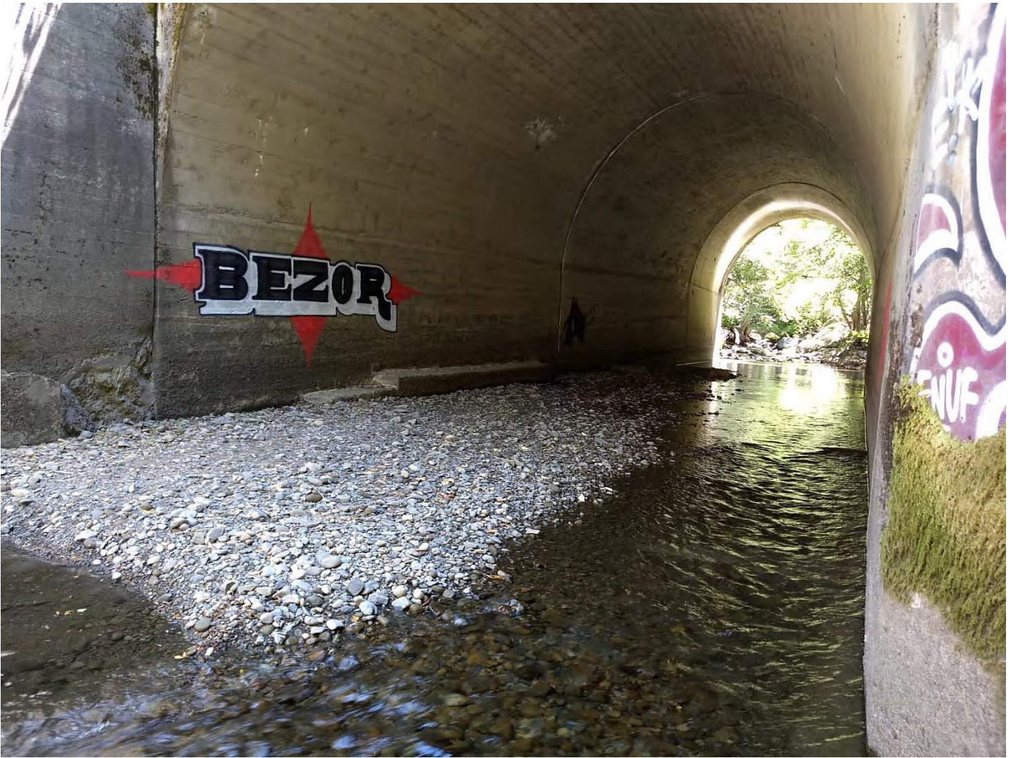
Figure 2. Sediment accumulating to form a natural substrate channel bottom within most of the culvert, view is upstream from the culvert outlet. Photo M. Lang on July 17, 2019.
