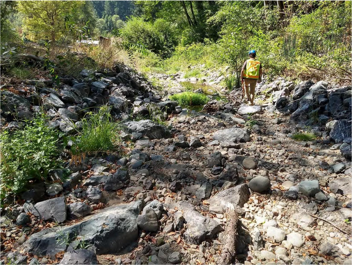
Figure 6. The downstream project channel looking downstream from the culvert outlet. Flow is discontinuous but surfaces behind most of the rock weirs. Photo by Margaret Lang on 9/12/2019.
