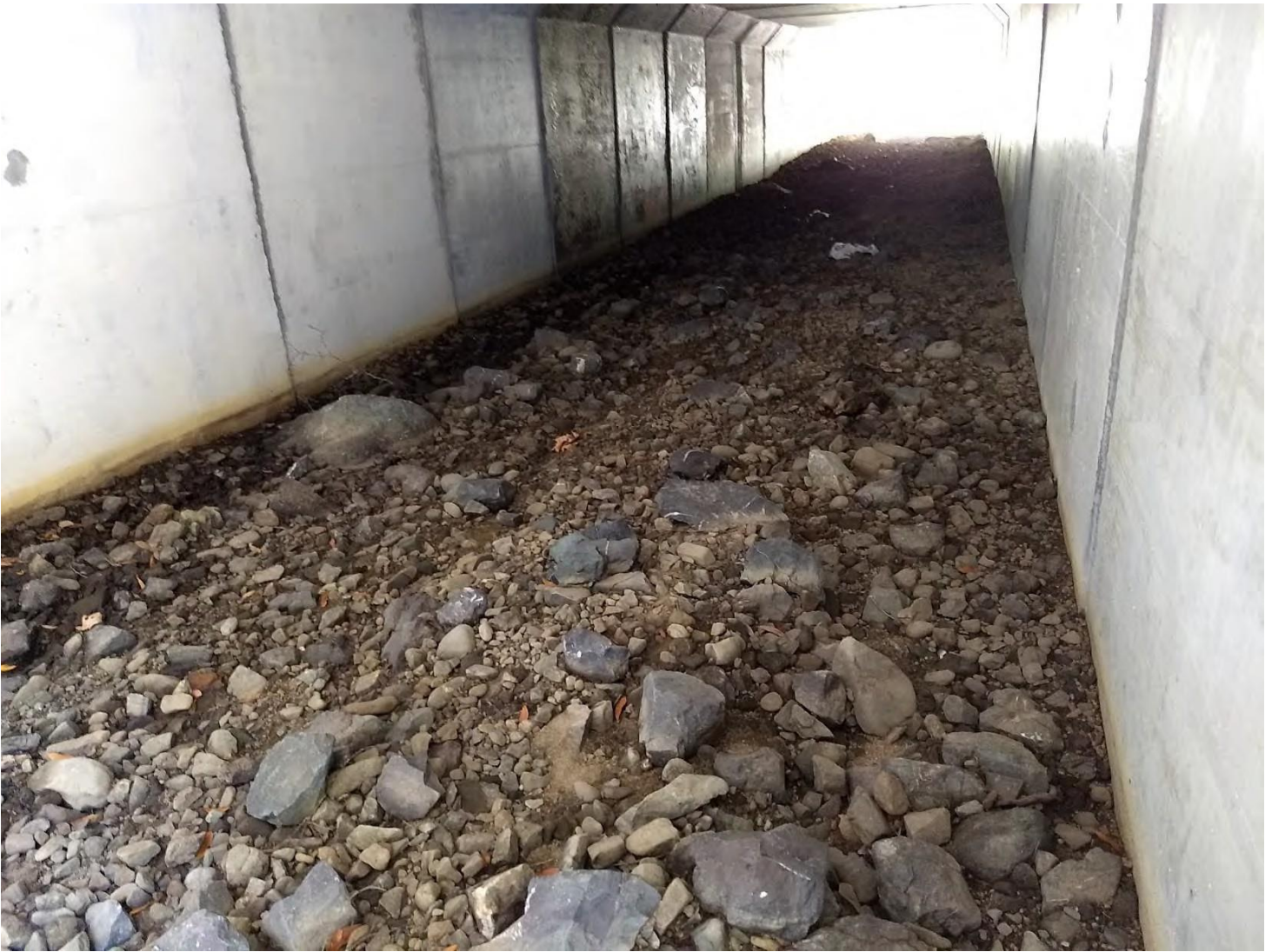
Figure 4. The culvert's invert and natural substrate bottom. The culvert substrate is almost a plain bed with the larger disruptor rocks mostly buried. At this low flow, there was no flow in the culvert, but it was very moist along the left side. Photo by Margaret Lang on 9/12/2019.
