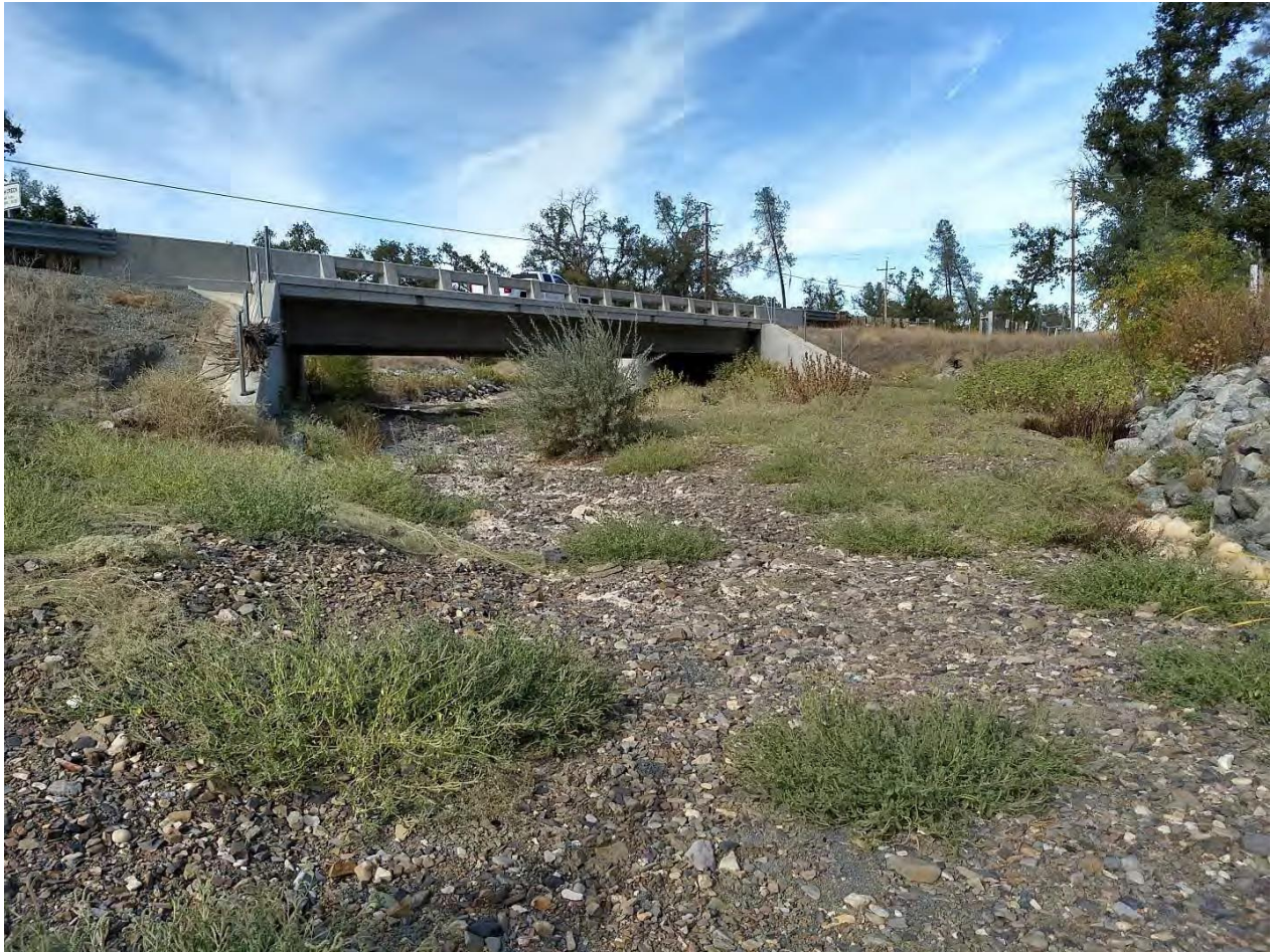
Figure 3. Lemm/Yank Creek Highway 299 bridge looking upstream. The creek channel is aligned with the thalweg along the left wingwall upstream, then crossing through the structure to the right wingwall downstream as shown in this picture. High flow debris was captured on the fence above the right wingwall as shown which matches debris at the same elevation as on the left wingwall fence upstream. Photo taken October 4, 2019.
