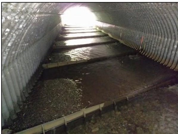
FIGURE 1-1. PEACOCK CREEK AT (A) CHANNEL DOWNSTREAM OF SR197, THE CULVERT OUTLET APRON (B) AT HIGH FLOWS AND (C) WITH WOOD PLUGGING NOTCH, (D) REPLACEMENT BAFFLES IN CULVERT IMMEDIATELY AFTER CONSTRUCTION AND AFTER SEDIMENT ACCUMULATION, AND (F) THE WOOD JAM ACROSS THE CHANNEL IMMEDIATELY UPSTREAM OF THE CULVERT INLET.
