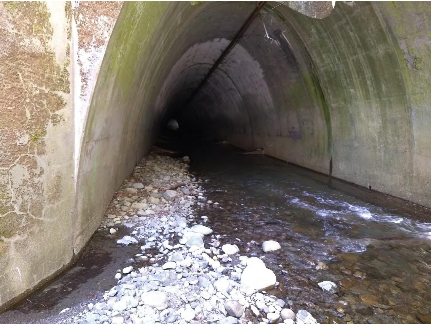
Figure 3. Cedar Creek culvert invert looking downstream from the inlet. The installed weirs are capturing sediment and maintaining a natural streambed near the inlet. Photo taken by M. Lang April 15, 2021.
