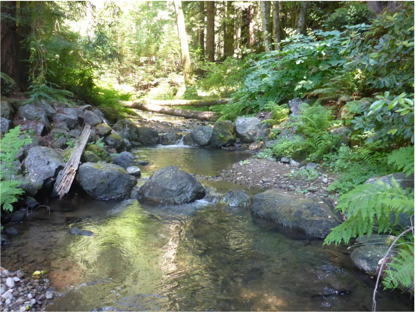
Figure 4. The two most upstream weirs in wider, lower gradient channel region and without the deep plunge pools. Photo by Michael Love on 7/17/2019.
