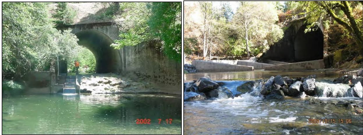
FIGURE 9-1. RATTLESNAKE CREEK CROSSING OUTLET BEFORE AND AFTER MODIFICATION. PHOTOS PROVIDED BY M. MOLNAR, CALTRANS.
