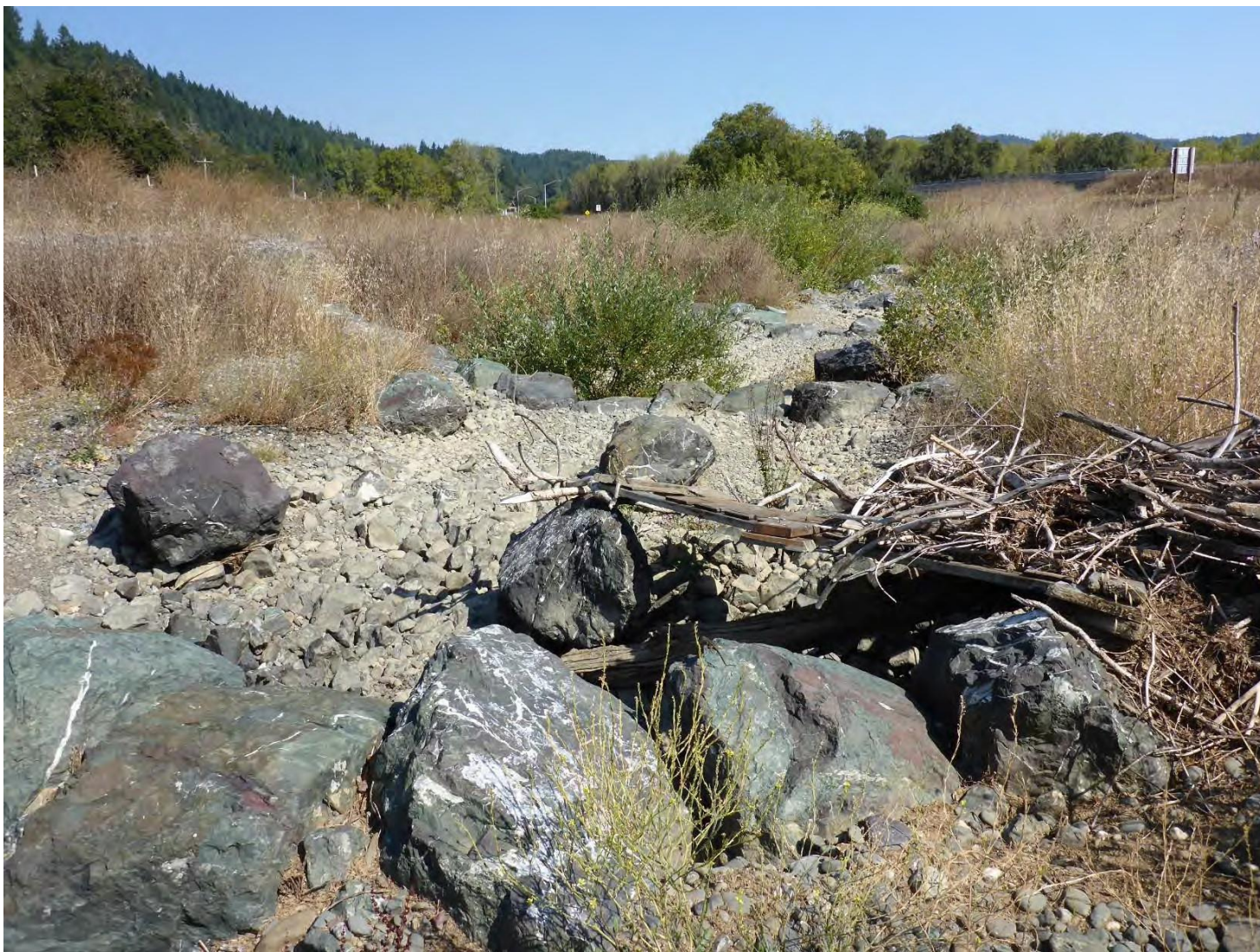
Figure 7. The older channel restoration just downstream of this project site was built at similar channel widths as the new channel under the bridge. This channel is being narrowed by encroaching willows. Photo by Michael Love on 9/12/2019.
