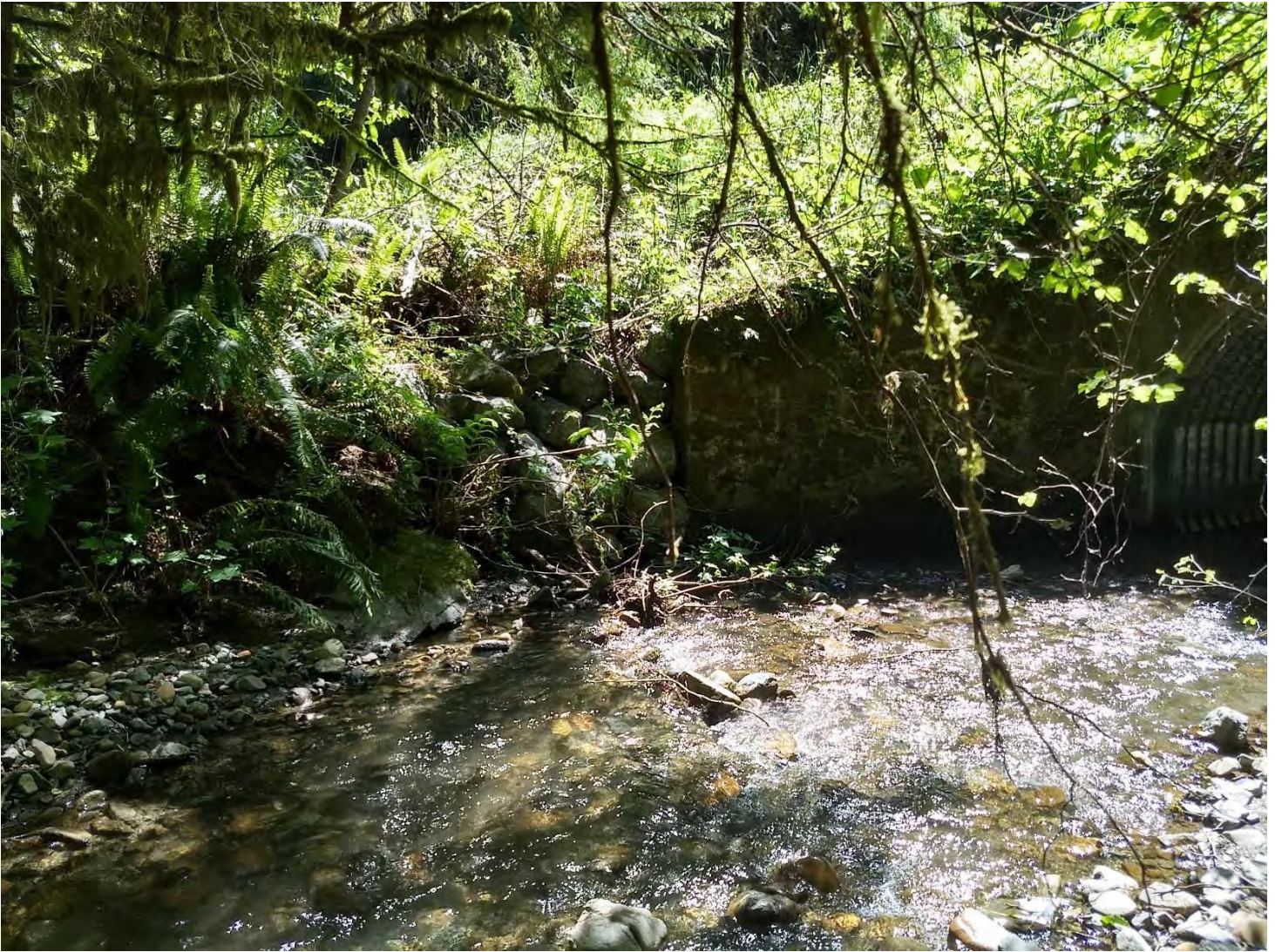
Figure 2. Left inlet wingwall showing some bank erosion from backwatering during high flows.
