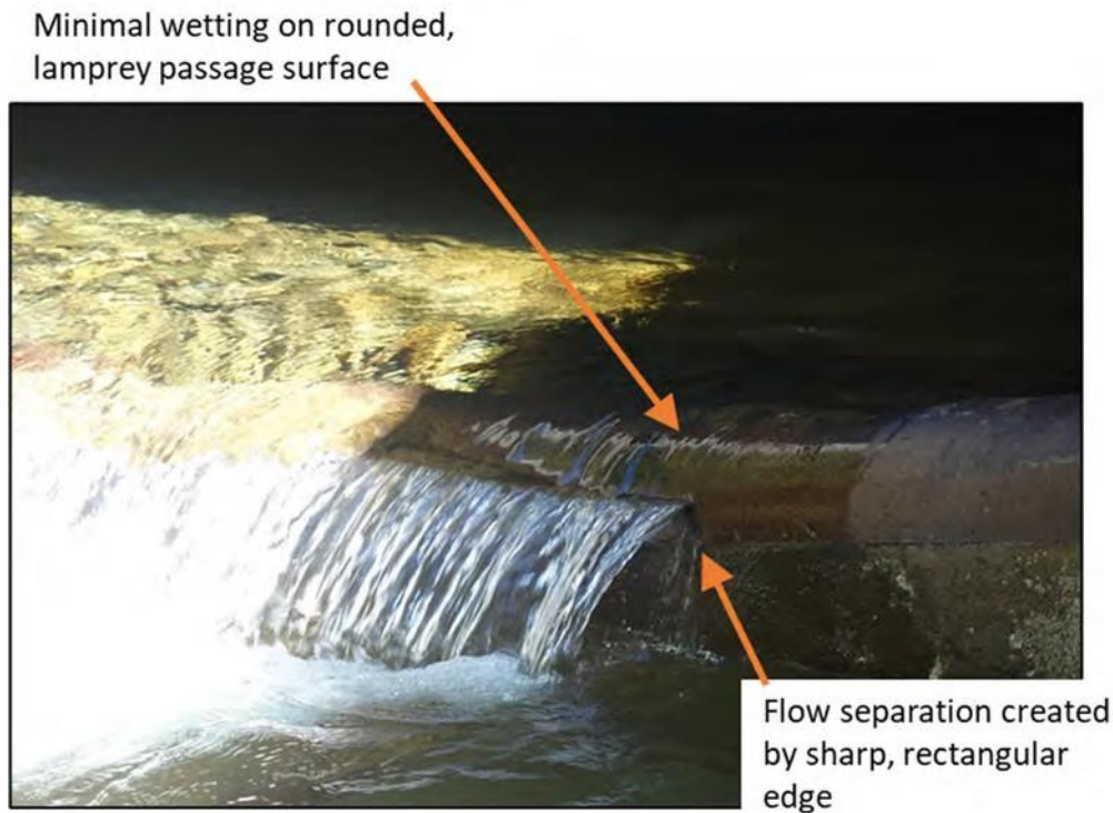
FIGURE 10-5. SOME OF THE OUTLET FISHWAY WEIRS HAVE SHARP EDGES AND PROTRUSIONS THAT MAY NOT BE EFFECTIVELY WETTING THE LAMPREY PASSAGE PORTION OF THE WEIR AND CREATE FLOW SEPARATION THAT COULD HINDER JUVENILE SALMONID PASSAGE. PHOTO TAKEN JUNE 3, 2020 BY M. LANG.
