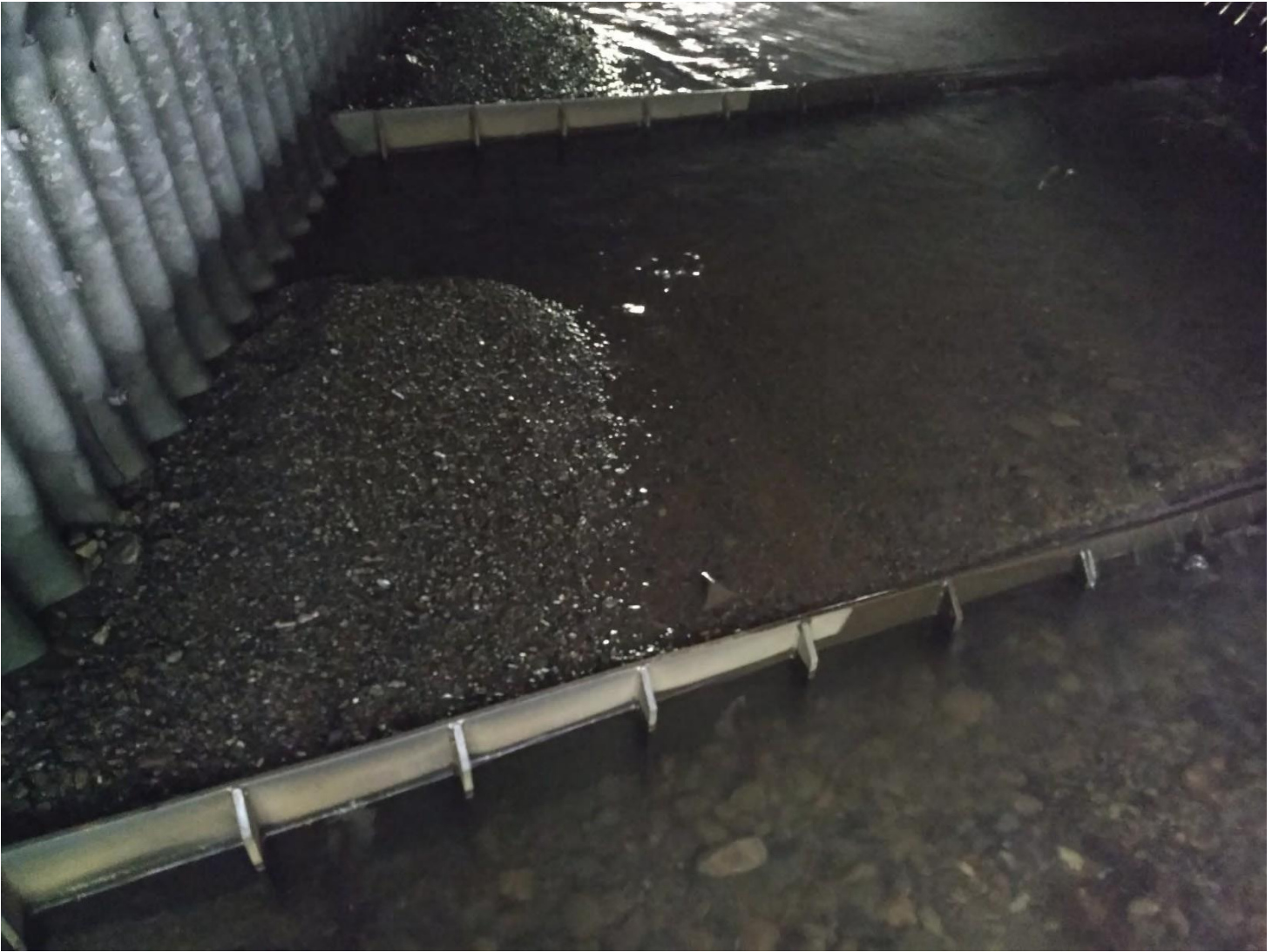
Figure 4. Sediment accumulation behind most baffles.
