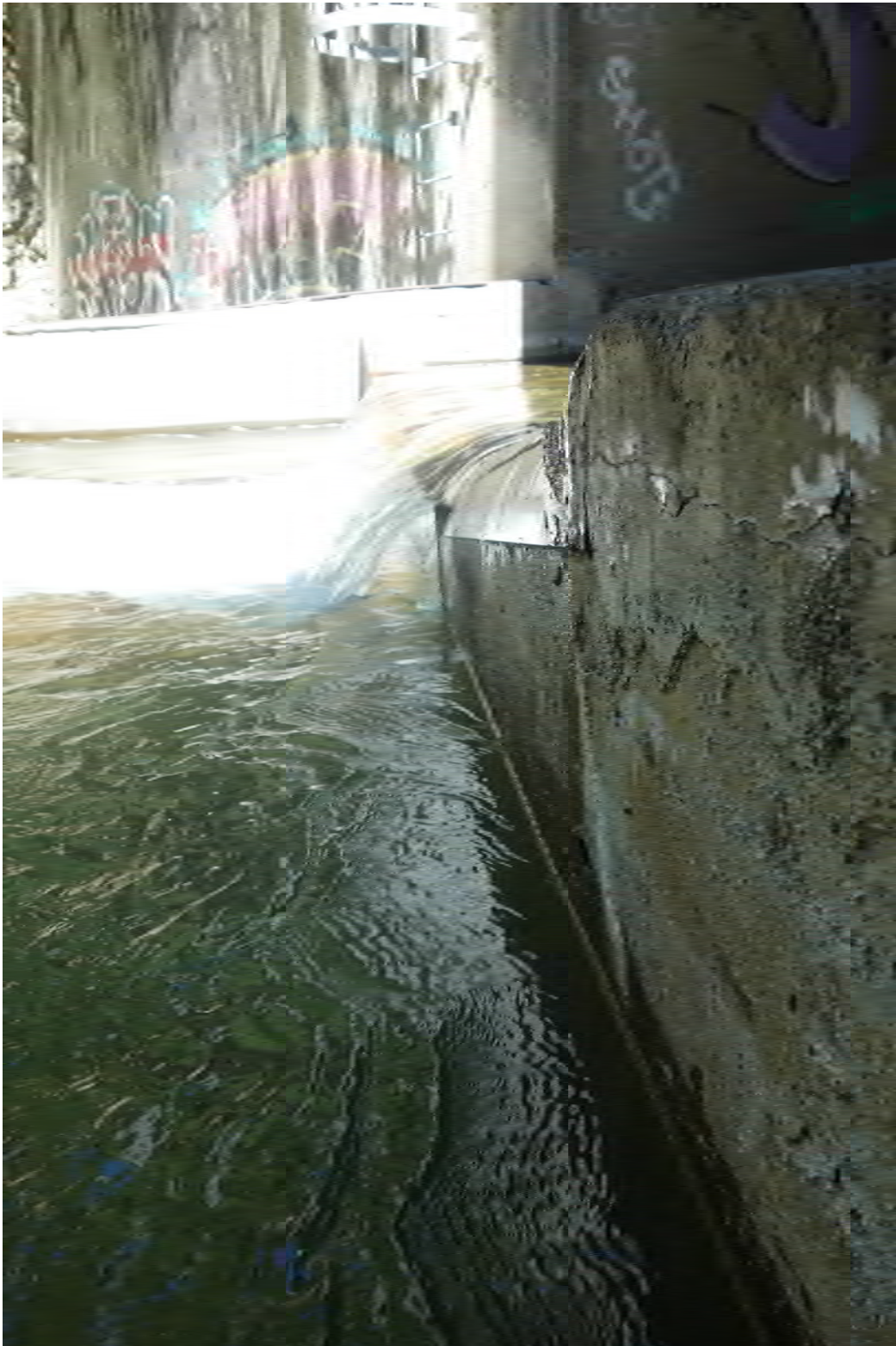
Figure 8. Cedar Creek culvert outlet weir. The concrete at this location has a small edge which was not smoothed out when the steel cover was installed. This edge creates a detached flow that does not wet the rounded section installed to assist lamprey migration. Photo taken June 3, 2021.
