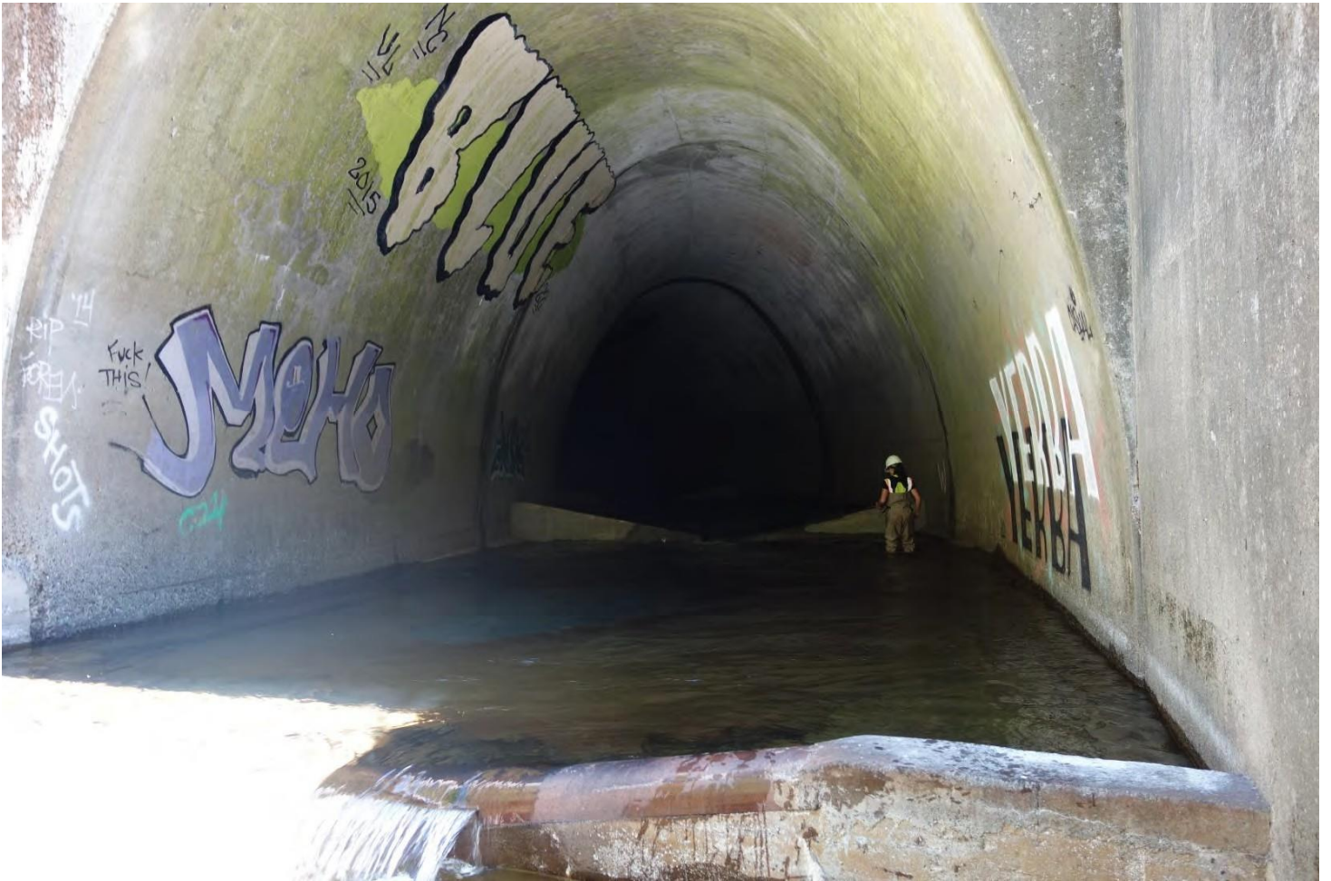
Figure 4. Cedar Creek culvert looking upstream from the outlet. The internal fish weirs are functioning well. Photo taken June 3, 2021.
