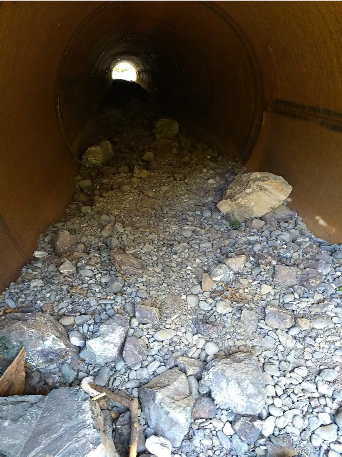
Figure 4. The higher culvert's invert and natural substrate bottom with keystone rocks looking downstream from the culvert inlet. Photo by Margaret Lang on 9/12/2019.
