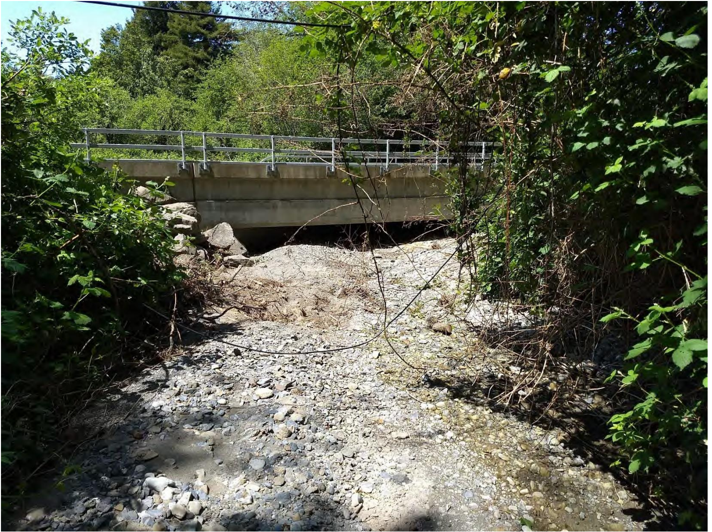
Figure 2. Sediment accumulation under the Sultan Creek bridge on Del Norte 197, postmile 5.00. View is looking downstream from the upstream channel.
