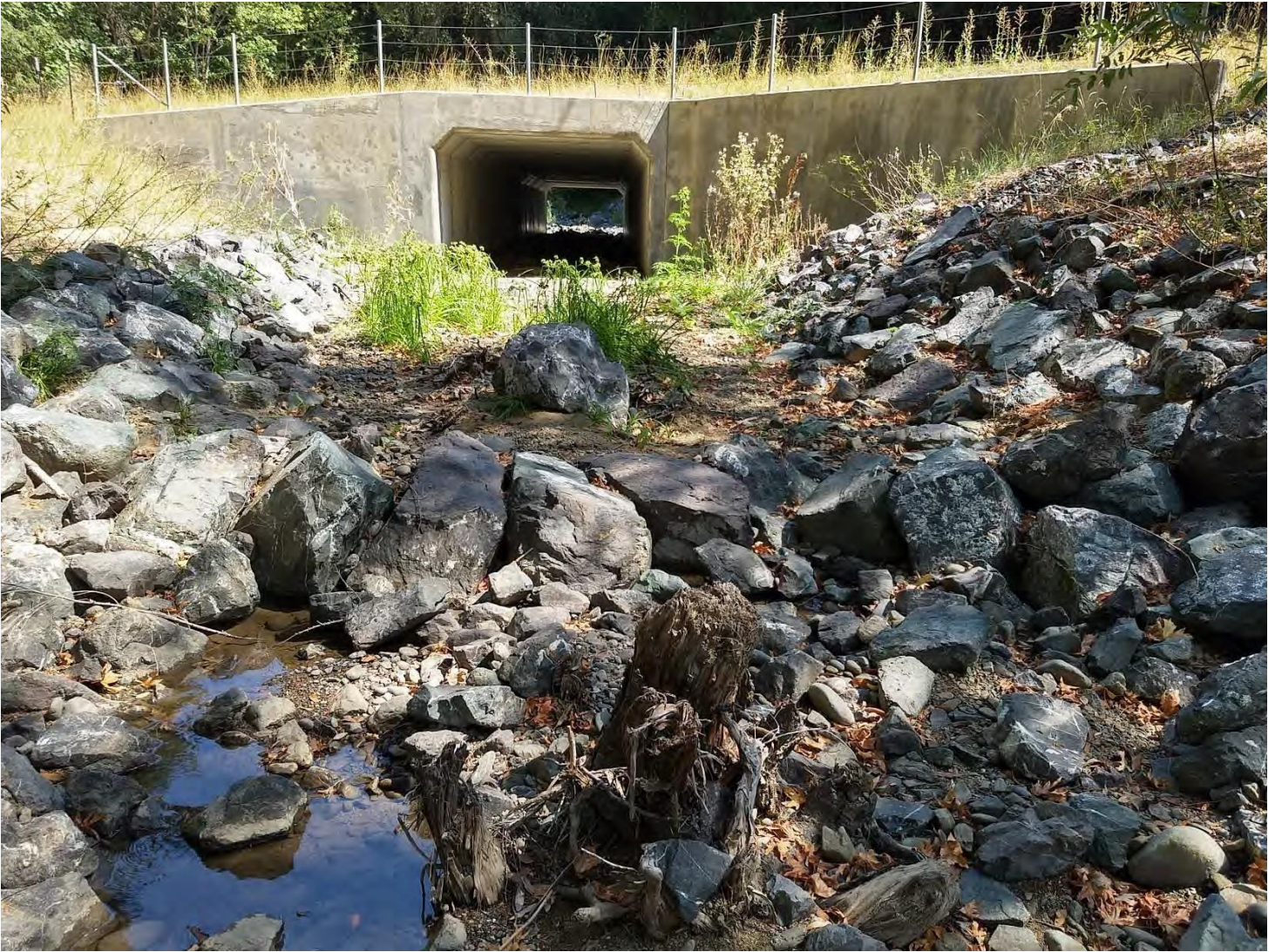
Figure 5. The culvert outlet looking upstream. The flow becomes discontinuous starting at the culvert inlet and remains discontinuous through the culvert and within the downstream project reach. Photo by Margaret Lang on 9/12/2019.
