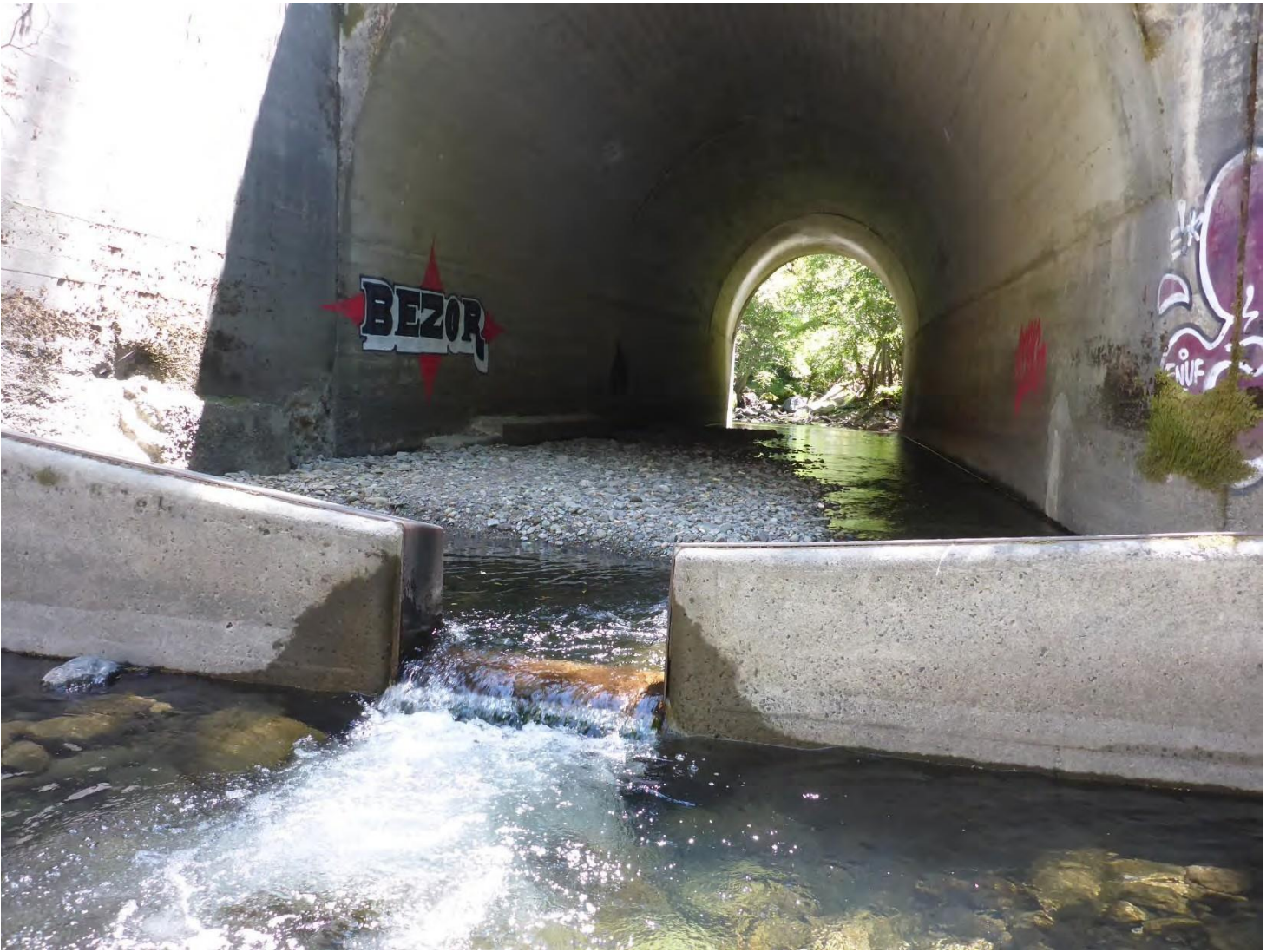
Figure 6. The culvert outlet and most upstream weir notch looking upstream from the from outlet weirs. Photo M. Love on July 17, 2019.
