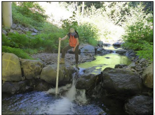
FIGURE 5-1. DUNN CREEK (A) UPSTREAM REFERENCE REACH, (B) TWO UPSTREAM-MOST WEIRS, (C) OVERALL PROJECT SHORTLY AFTER CONSTRUCTION, (D) TYPICAL WEIR UPSTREAM OF BRIDGE, (E) EXCESS POOL SCOUR BELOW U-SHAPED WEIR, AND (F) EXCESSIVE DROP OVER WEIR 2 AFTER DOWNSTREAM-MOST WEIR FAILURE.
