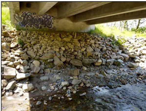
FIGURE 3-2. LITTLE MILL CREEK (A) BRIDGE LOOKING DOWNSTREAM, (B) STEEP CHANNEL SECTION FLOWING INTO SMITH RIVER DOWNSTREAM OF BRIDGE, (C) BRIDGE LOOKING DOWNSTREAM (D) LOOKING UPSTREAM AT CHANNEL AND DEPOSITIONAL BAR UNDER BRIDGE, (E) CLOSE UP OF SCOURED RSP TOE UNDER BRIDGE, AND (F) LOOKING UPSTREAM AT THE REFERENCE REACH.
