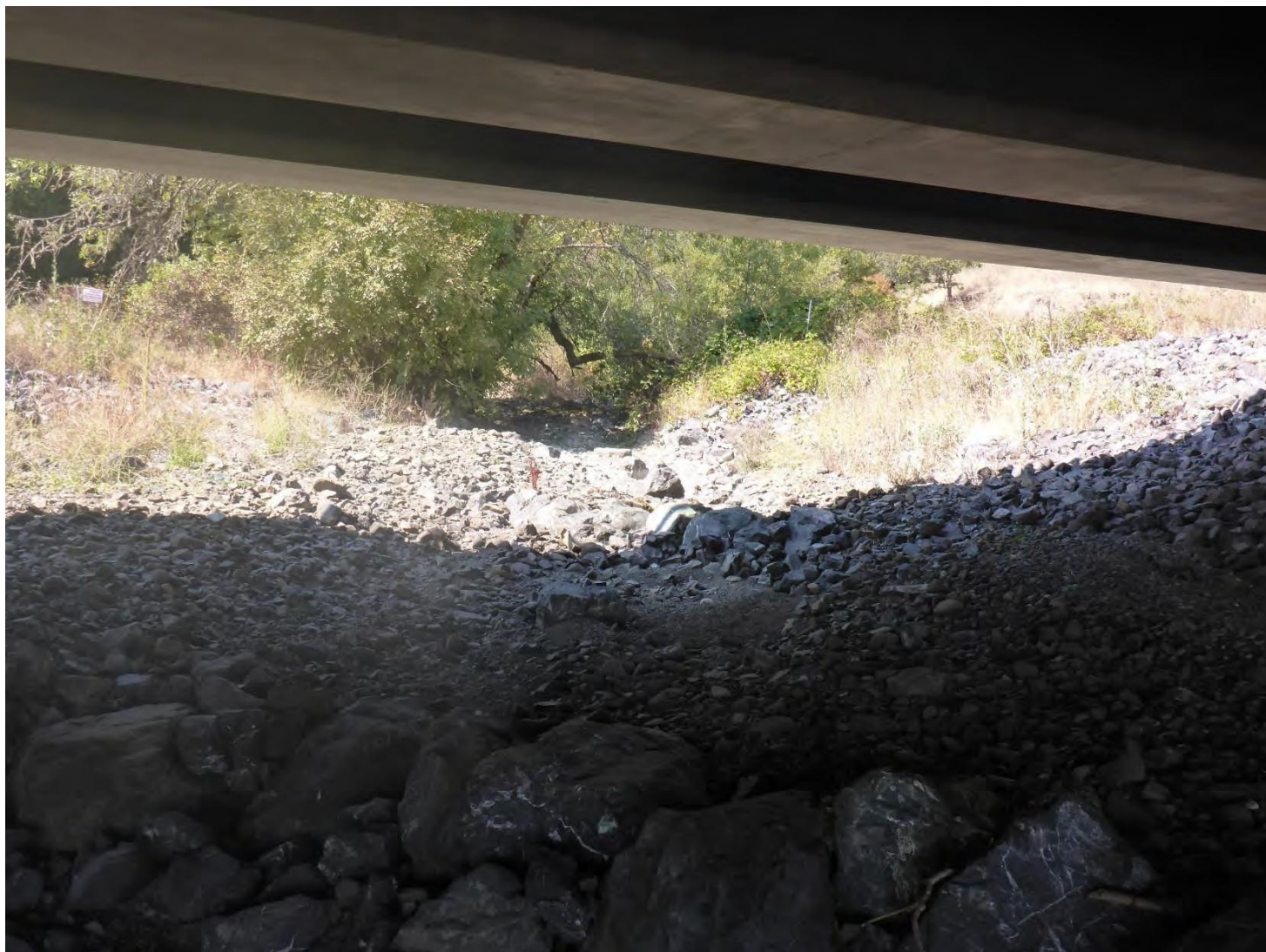
Figure 1. View looking upstream from beneath the new bridge. The most upstream V-shaped rock weir is in the foreground and the straight rock weir upstream of this weir is missing. Photo by Michael Love on 9/12/2019.
