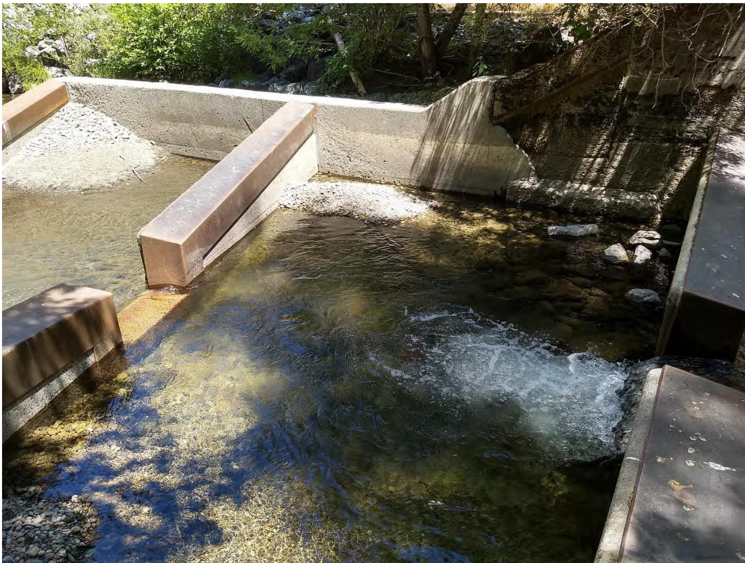
Figure 3. Sediment trapping and pool maintenance in the outlet weirs. Photo M. Lang on July 17, 2019.
