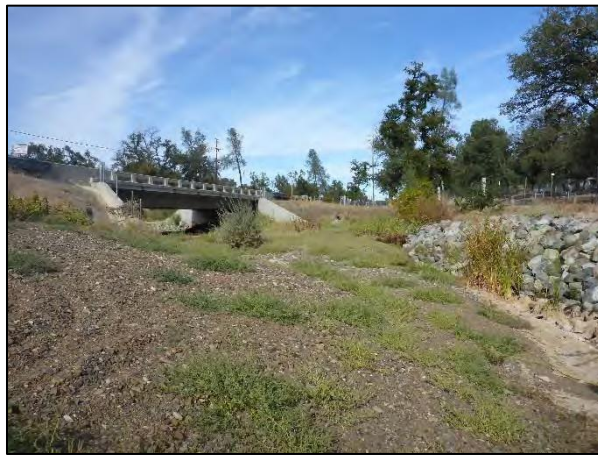
FIGURE 11-2. YANK (LEMM) CREEK (A) UPSTREAM CHANNEL, (B) LOOKING DOWNSTREAM AT THE BRIDGE- NOTE HIGH WATER DEBRIS ON LEFT BANK, (C) CHANNEL UNDER THE BRIDGE SHOWING SKEW FROM LEFT TO RIGHT BANK (D) LOOKING UPSTREAM AT THE BRIDGE — NOTE HIGH WATER DEBRIS ON RIGHT BANK, (E) LOOKING UPSTREAM AT BRIDGE AND 90-DEGREE CHANNEL BEND, AND (F) ARMORED DOWNSTREAM CHANNEL AFTER 90-DEGREE BEND. PHOTOS TAKEN OCT 4, 2019 BY M. LOVE AND M. LANG.
