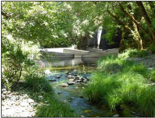
FIGURE 9-2. RATTLESNAKE CREEK (A) UPSTREAM CHANNEL (B) CULVERT BARREL IS RETAINING SUBSTRATE AND FORMING A LOW FLOW CHANNEL (C & D) OUTLET POOL AND WEIR FISHWAY, (E) OUTLET AND FISHWAY LOOKING UPSTREAM FROM THE OUTLET POOL TWC, AND (F) DOWNSTREAM CHANNEL. ALL PHOTOS TAKEN JULY 17, 2019.
