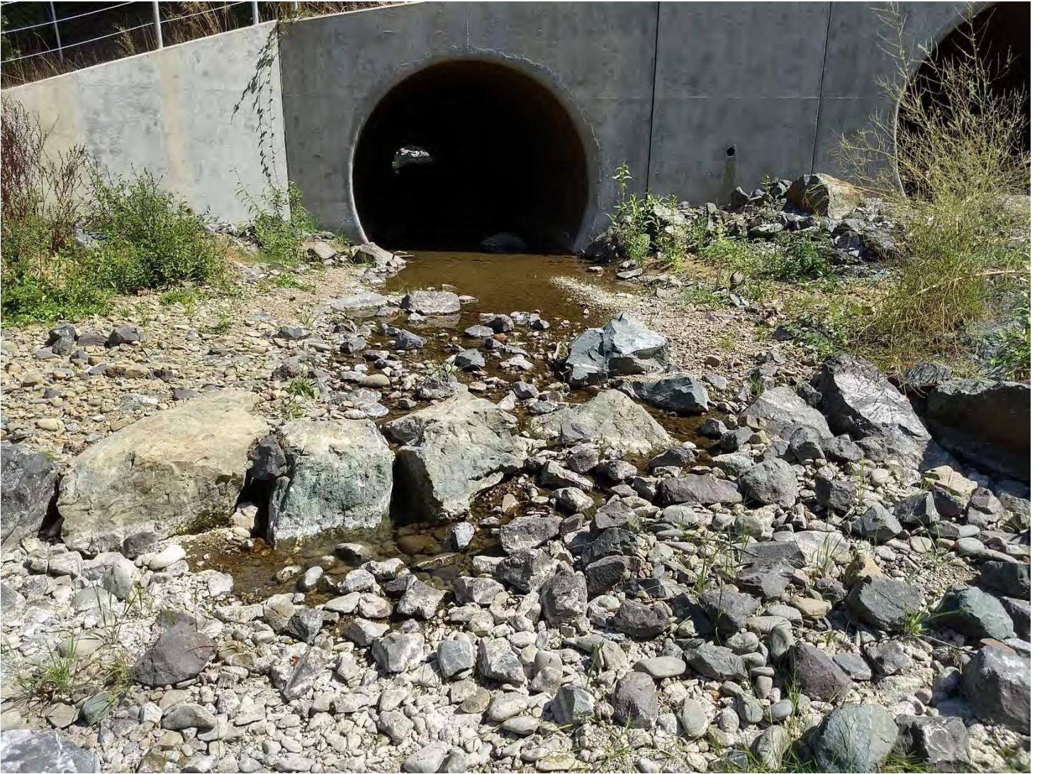
Figure 6. The lower culvert's outlet looking upstream. At low flows, the flow goes subsurface and was discontinuous starting at the first rock weir downstream as seen in the photo's foreground. Photo by Margaret Lang on 9/12/2019.
