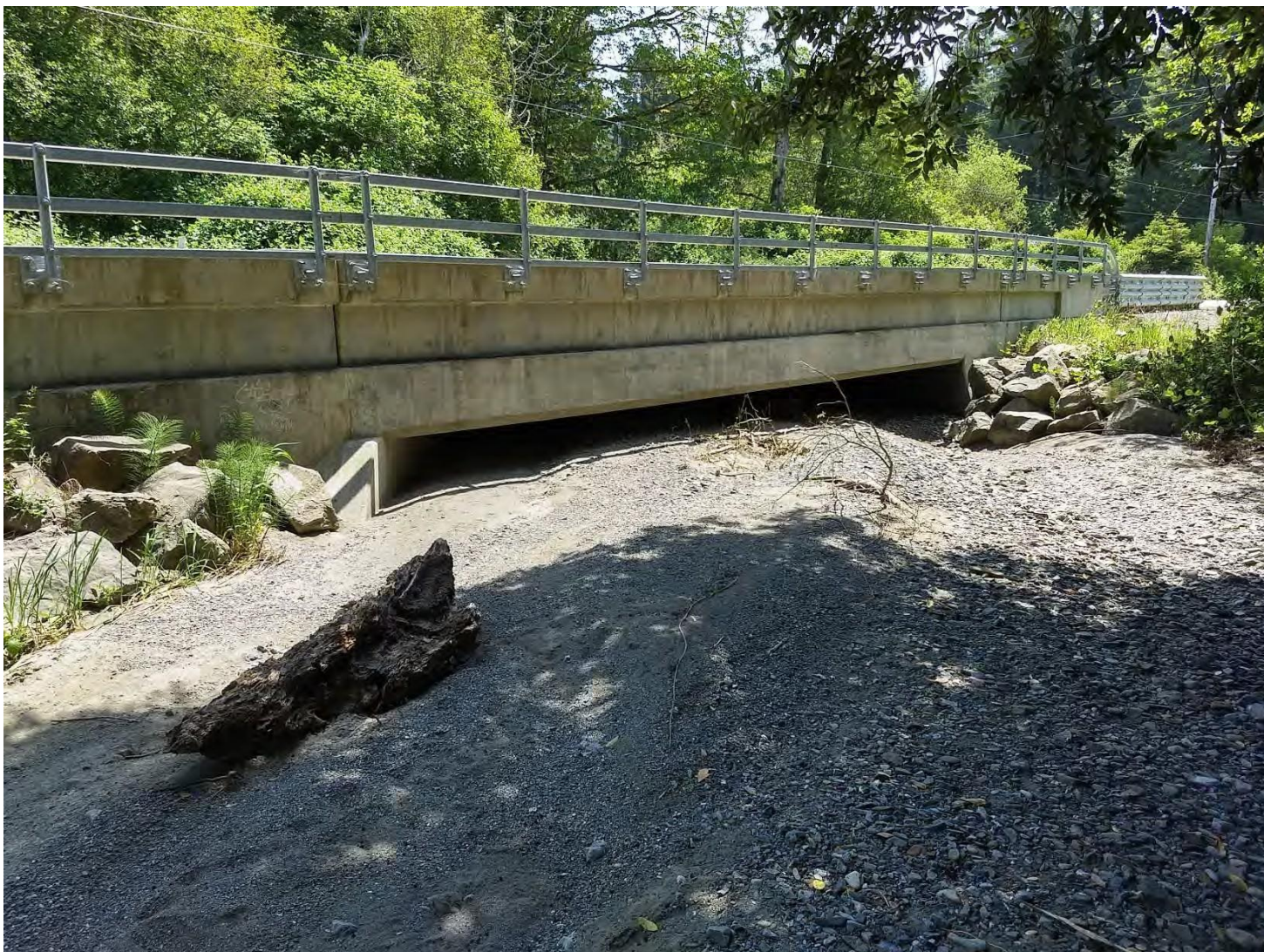
Figure 1. Sediment accumulation under the Sultan Creek bridge on Del Norte 197, postmile 5.00. View is looking upstream from the downstream channel.
