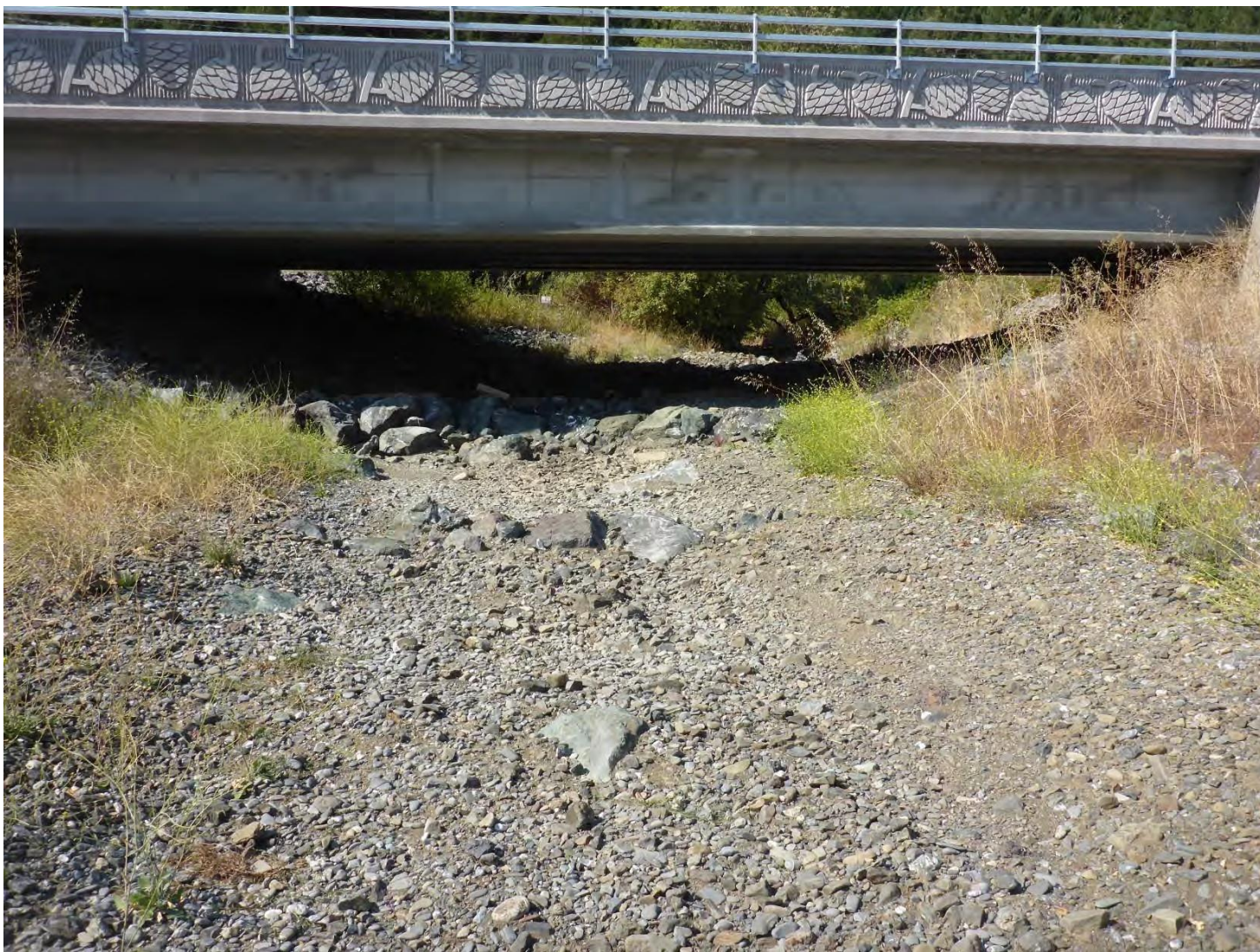
Figure 6. The weir just downstream of the bridge appear to be backwatered and being buried in sediment. Photo by Michael Love on 9/12/2019.
