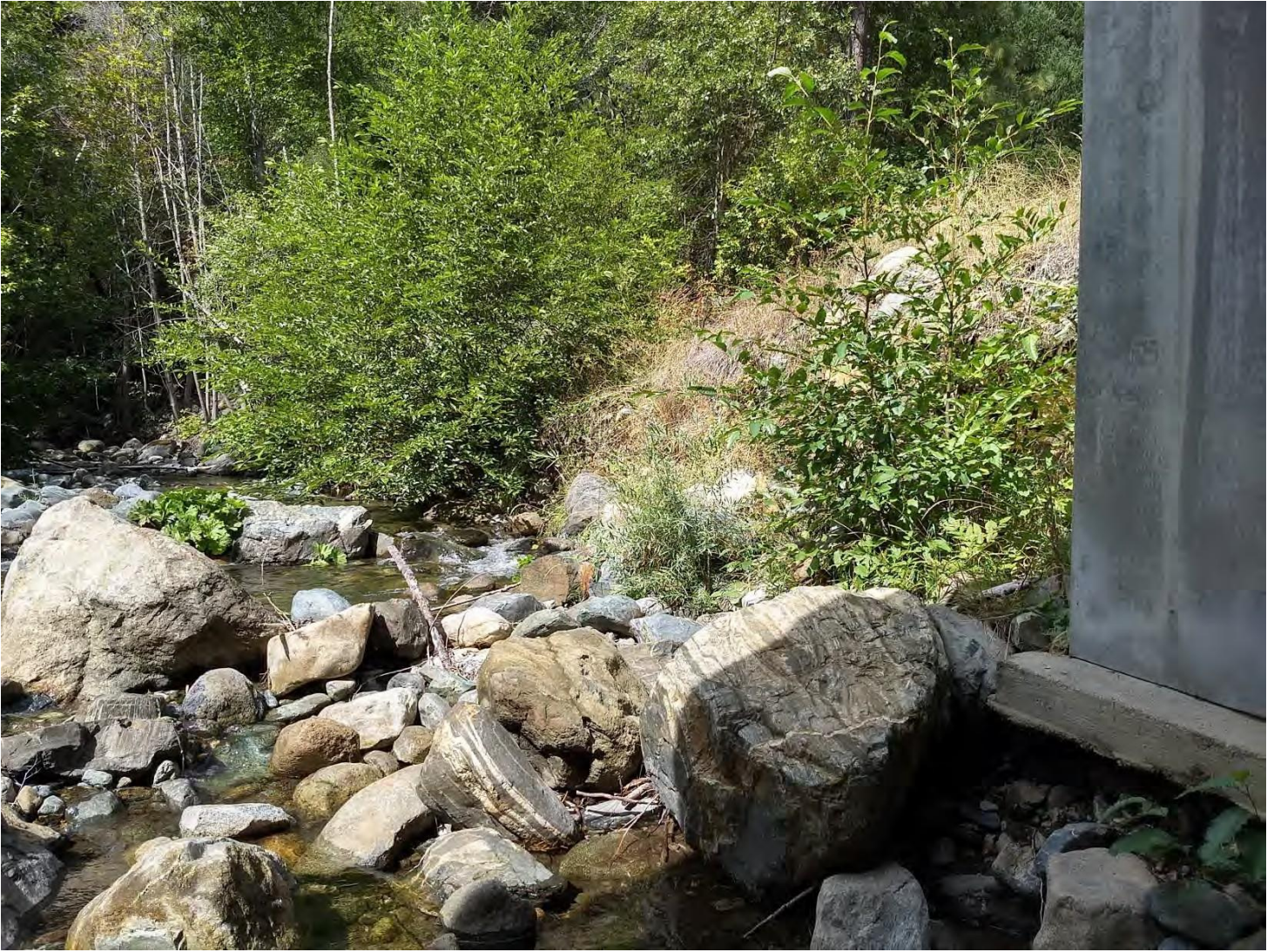
Figure 5. Upstream, left bank and bridge footing showing scoured bank protection and exposed footing. This is an outer channel bend coming into the bridge project site. Photo by M. Lang on 9/19/2019.
