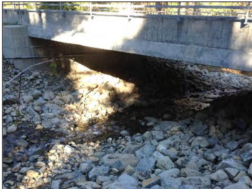
FIGURE 13-2. O'NEIL CREEK BRIDGE AND STREAMBED IN 2013 FOLLOWING STREAMBED REMEDIATION TO INTRODUCE FINE SEDIMENTS AND COMPACT THE BED MATERIAL TO MITIGATE FOR LOW FLOWS GOING SUBSURFACE. PHOTOS PROVIDED BY CALTRANS.
