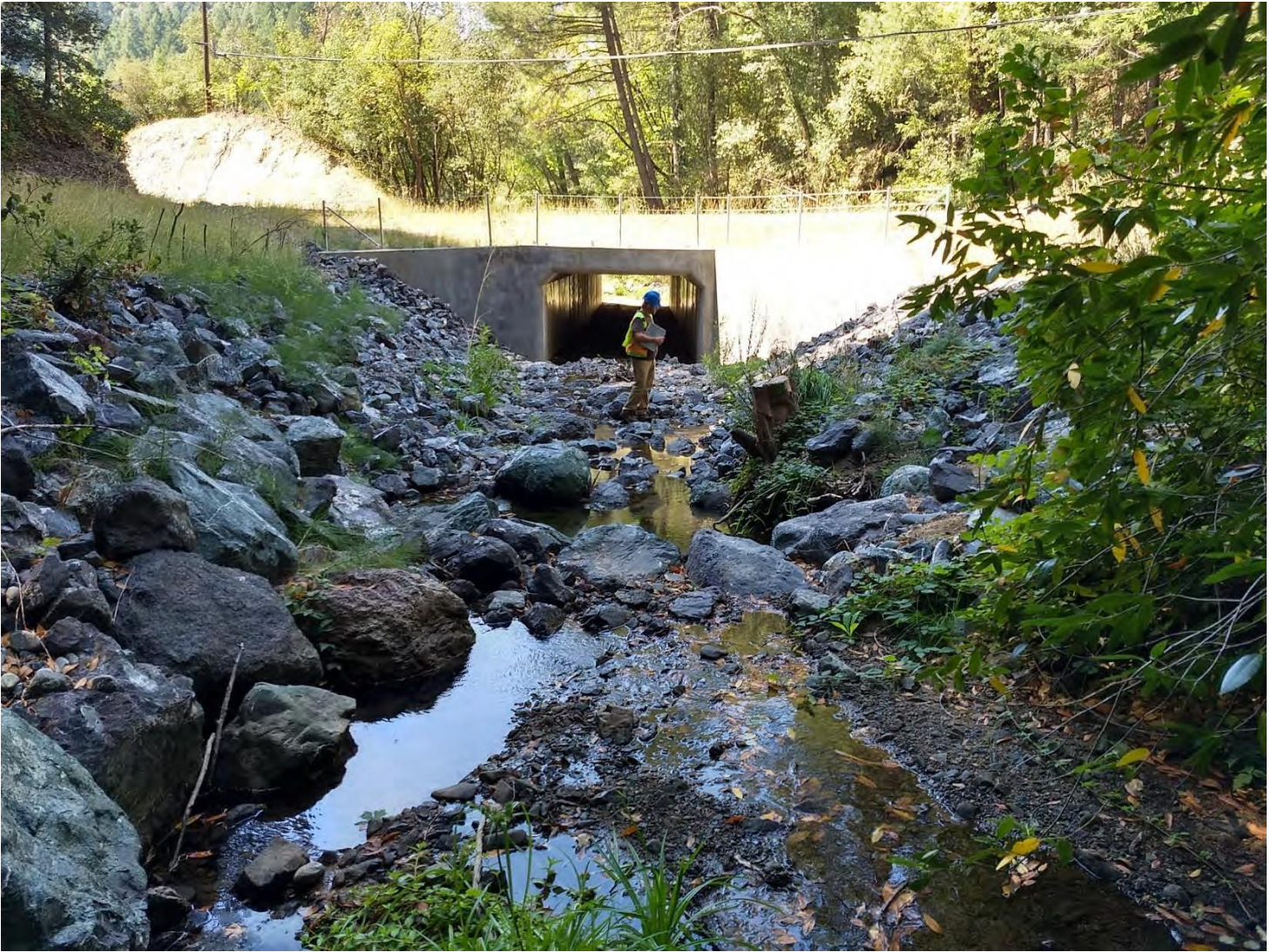
Figure 3. Culvert inlet looking downstream from the upstream project boundary. Stream flow was low but continuous upstream of the culvert during this site visit. Photo by Margaret Lang on 9/12/2019.
