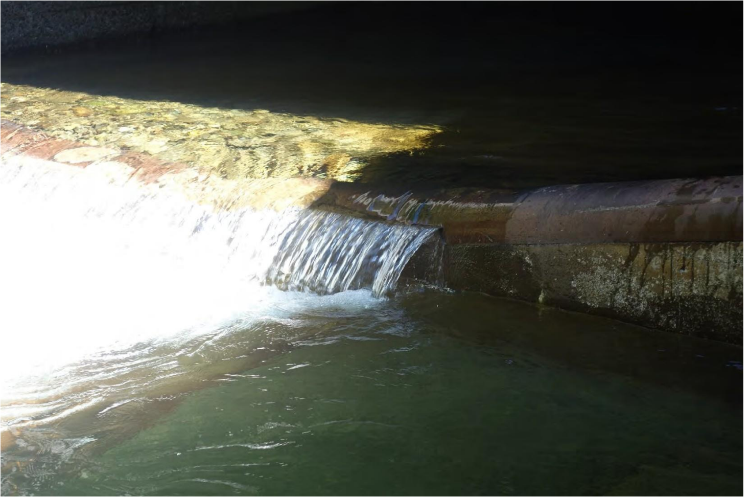
Figure 9. Cedar Creek culvert outlet weir. The concrete at this location has a small edge which was not smoothed out when the steel cover was installed. This edge creates a detached flow that does not wet the rounded section installed to assist lamprey migration. Photo taken June 3, 2021. (alternate view to supplement Figure 8)
