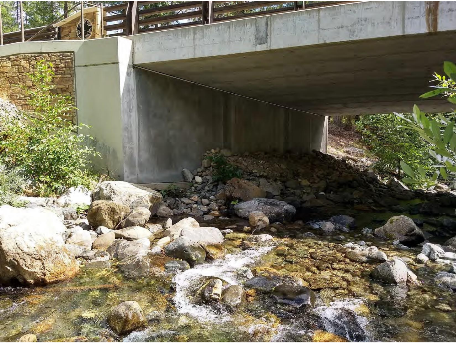
Figure 3. Upstream, left bank of bridge showing scoured bank protection and exposed footing. Photo by M. Lang on 9/19/2019.
