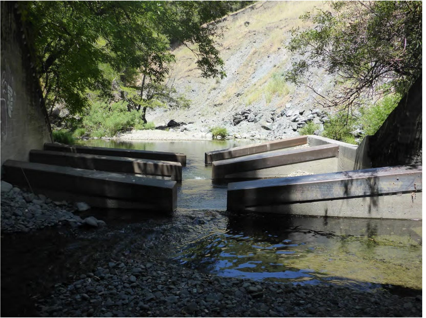
Figure 4. The outlet pool weirs and right channel bank looking downstream from the culvert outlet. The modifications to add the weirs and reorient the outlet flow away from the right bank has reduced the erosion of the right channel bank. Photo M. Love on July 17, 2019.
