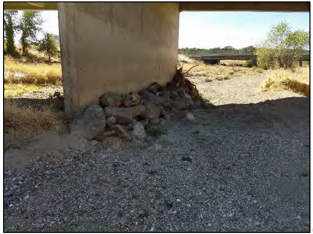
FIGURE 14-1. DIBBLE CREEK (A) UPSTREAM CHANNEL LOOKING DOWNSTREAM AT CROSSING (MAIN CHANNEL ON LEFT OF PICTURE), (B) LOOKING DOWNSTREAM AT THE ROCK RAMP (SHEET PILING GRADE CONTROL IN FOREGROUND), (C) LOOKING UPSTREAM AT ROCK RAMP (D) LOOKING DOWNSTREAM AT ROCK RAMP AND CHANNEL, (E) LOOKING UPSTREAM AT CROSSING, AND (F) EXAMPLE OF ARMORED BRIDGE PIERS IN MAIN CHANNEL. PHOTOS TAKEN OCT 2019 BY M. LOVE AND M. LANG.
