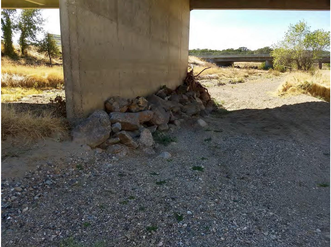
Figure 2. Dibble Creek middle footing of southbound Highway 5 bridge looking upstream at the frontage road bridge. The main channel is on the left of this picture. The left channel has much finer sediment. Photo taken October 4, 2019.
