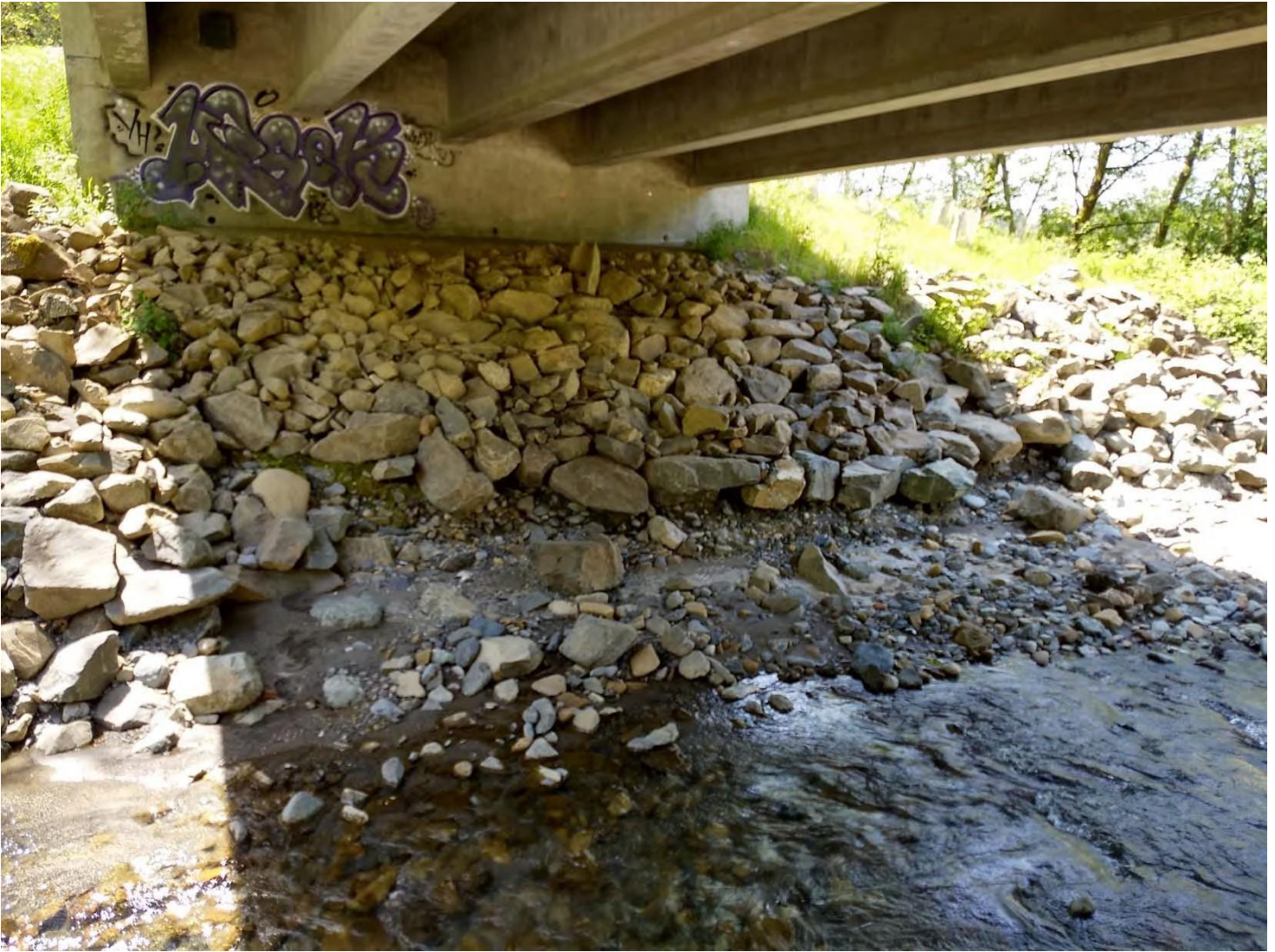
Figure 5. Left bank erosion of rip rap toe. Lowest rock appears to be missing.
