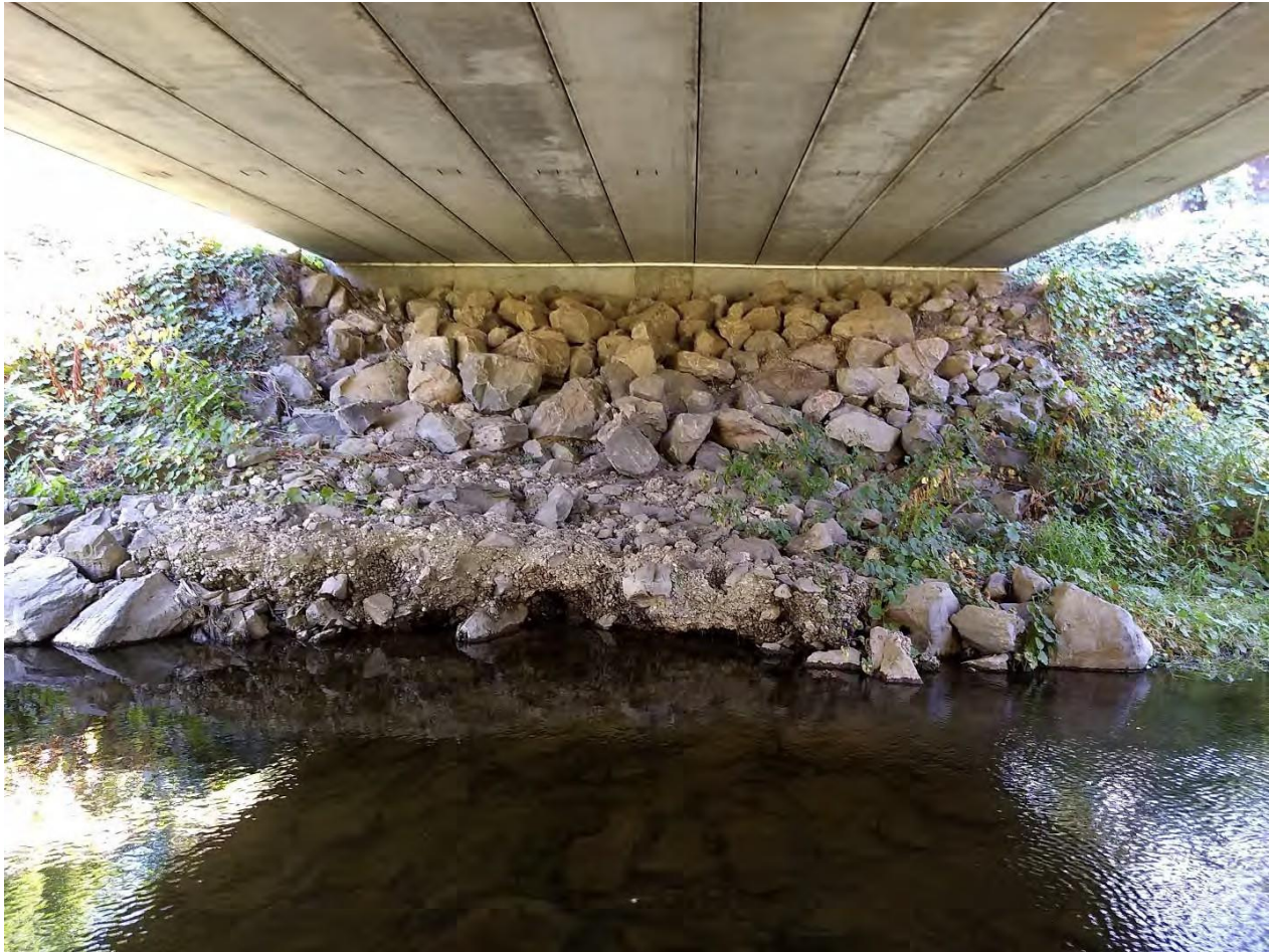
Figure 6. Craig Creek Right bank erosion and loss of bank protection by undercutting at the crossing. Photo taken October 4, 2019.
