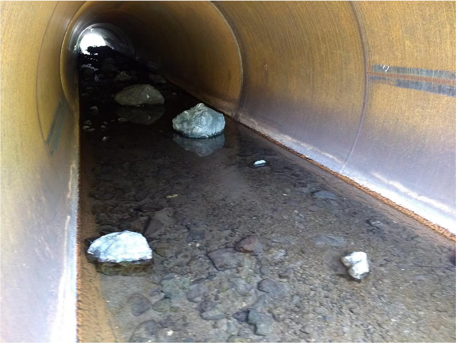
Figure 5. The lower culvert's invert and natural substrate bottom with keystone rocks looking downstream from the culvert inlet. Photo by Margaret Lang on 9/12/2019.
