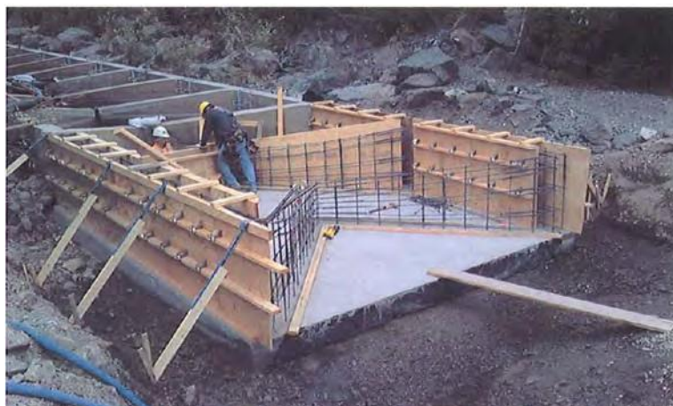
FIGURE 4-2. DOWNSTREAM FISHWAY EXTENSION UNDER CONSTRUCTION IN AUGUST, 2013.
