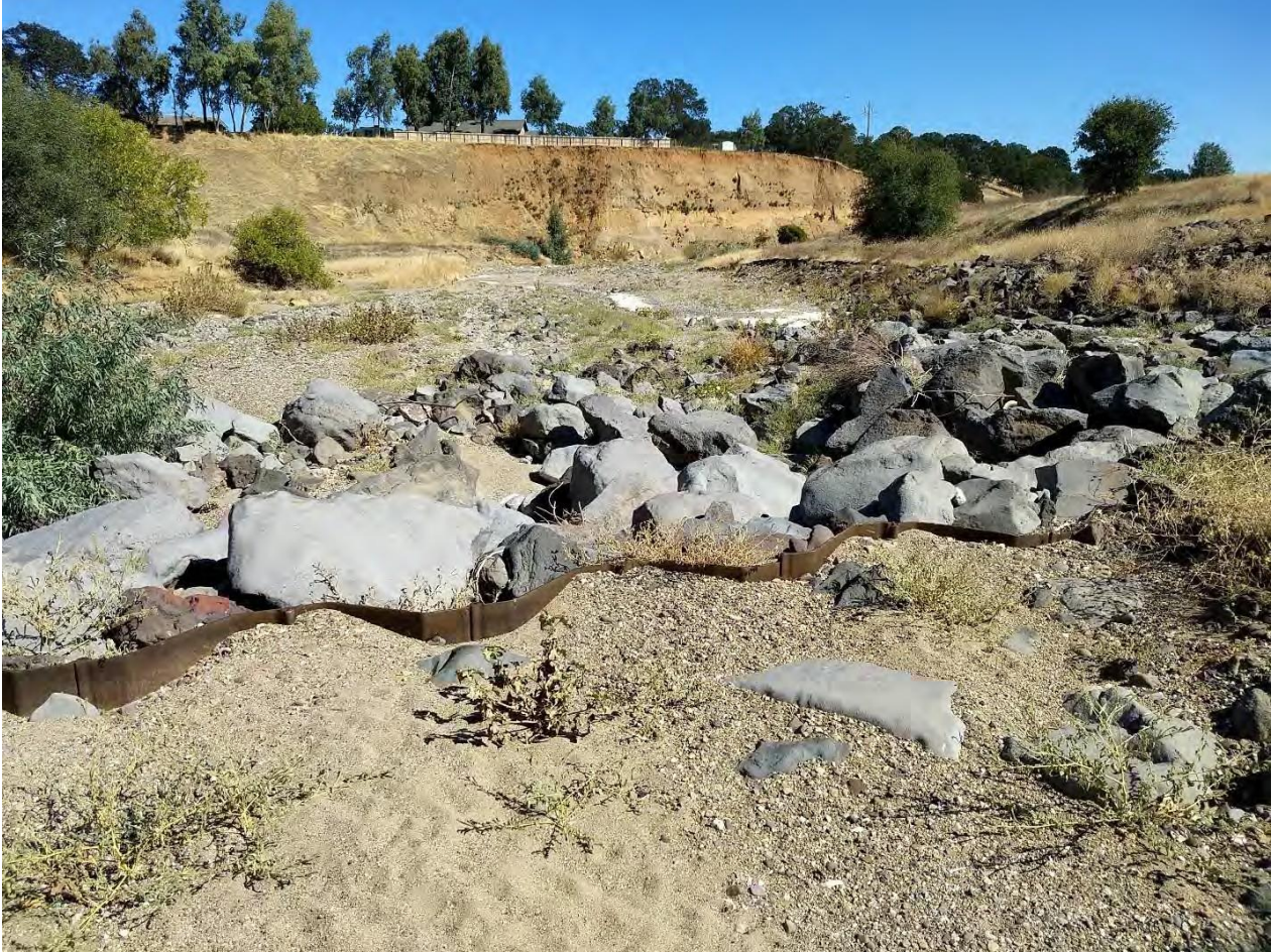
Figure 3. Dibble Creek looking downstream from the bridge left span. The low flow channel is on the right. The high rock weir in the picture forefront controls water elevation in the left channel to guide water to the low flow channel on the right. The sheet piling is just visible upstream of the rocks and is present but at lower creat elevation on both sides of the channel. Photo taken October 4, 2019.
