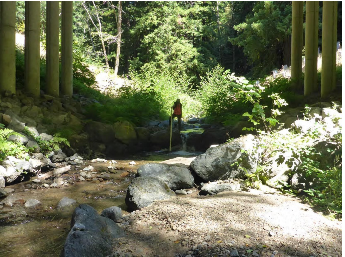
Figure 1. Most downstream rock weir that has failed is in foreground. The next weir is currently in place but now has a 1.8 ft elevation drop at low flow. Photo by Michael Love on 7/17/2019.
