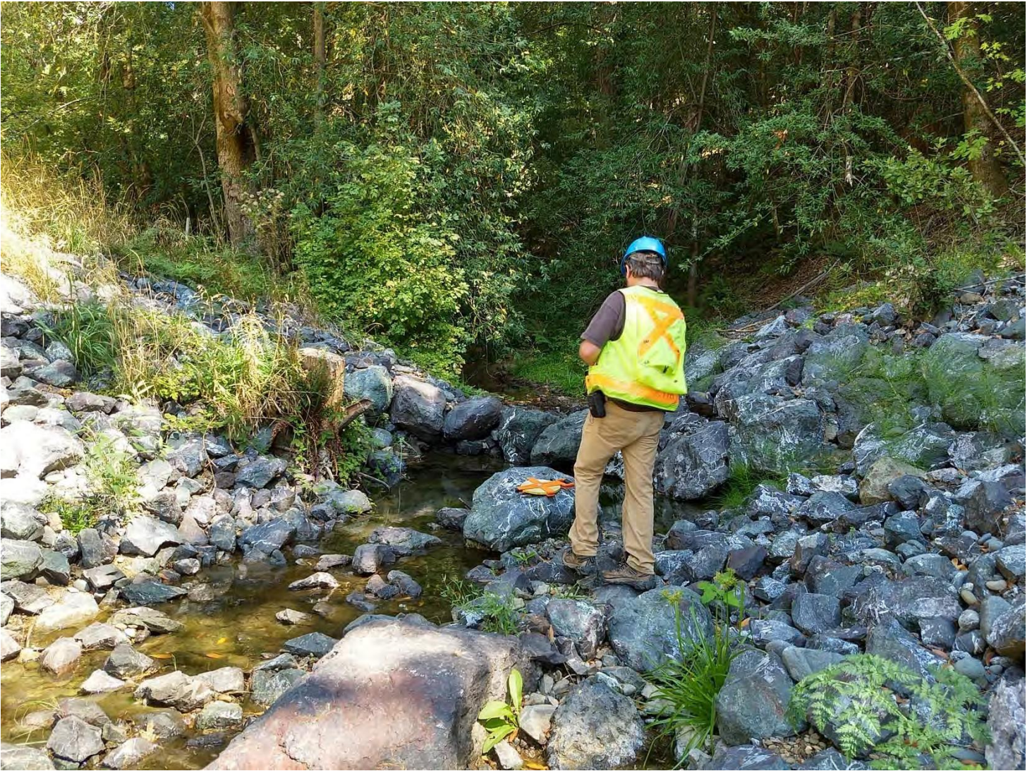
Figure 2. Close-up view of the upstream rock weir. The footing rocks are exposed in the pool increasing the potential for weir failure. Note that the low flow is going through the rocks in the weir rather than over the crest. Photo by Margaret Lang on 9/12/2019.
