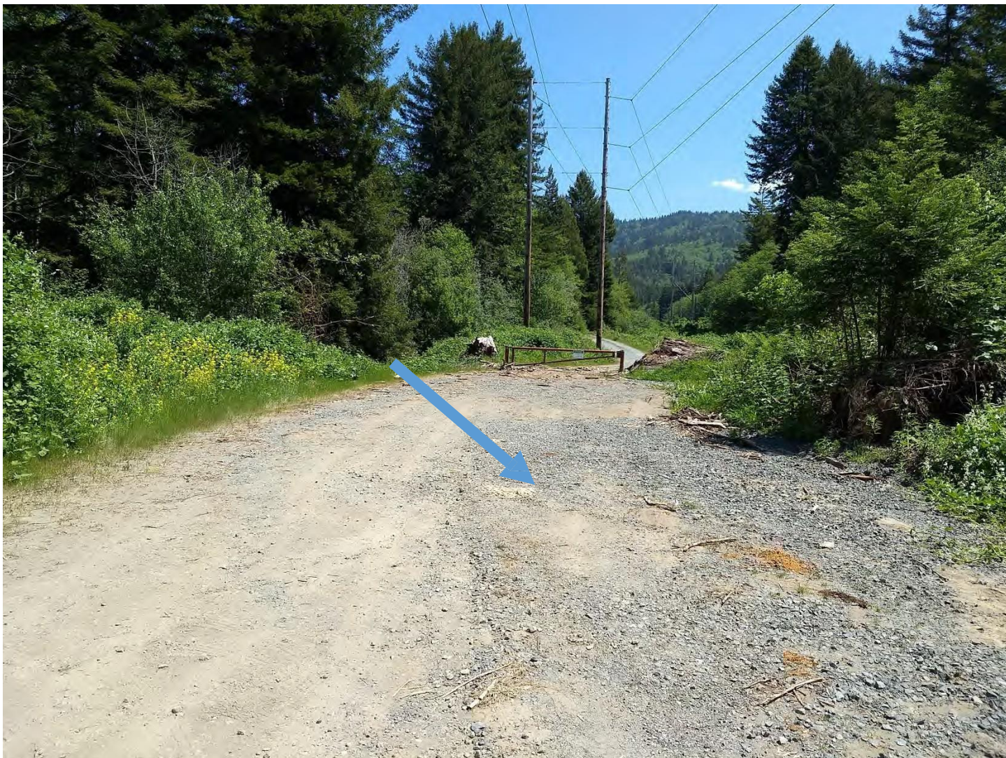
Figure 3. At high flow, water leaves the channel at this location and flows down the Green Diamond access road. There is a debris jam and channel bend at this location in the main channel.
