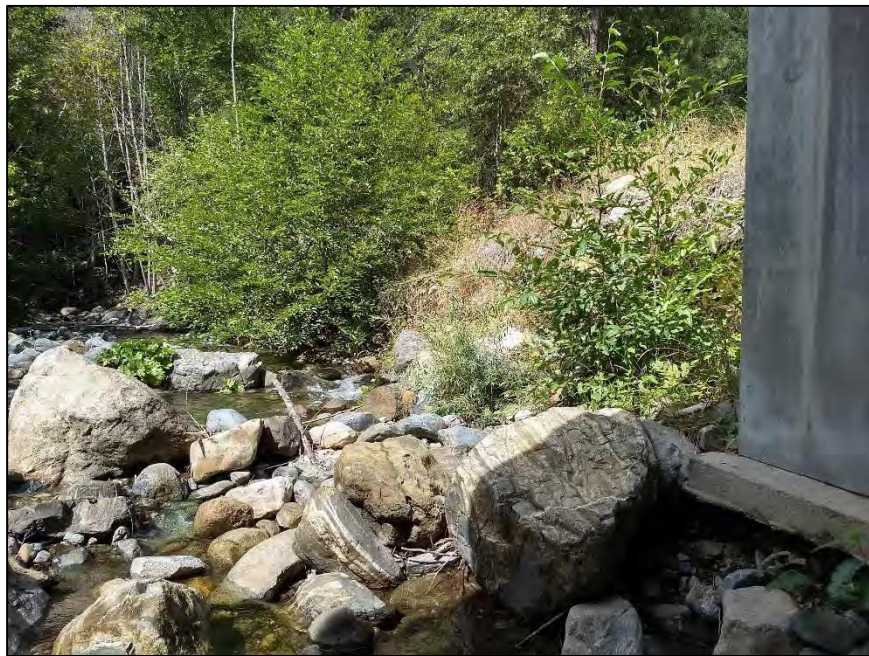
FIGURE 12-4. UPSTREAM LEFT BANK SCOUR (A) LOOKING DOWNSTREAM AT SCoured BANK BENEATH THE BRIDGE AND (B) LOOKING UPSTREAM AT ROCK POSSIBLY ADDED LATER TO PROTECT THE FOOTING. PHOTO TAKEN SEPT 19, 2019 BY M. LANG.
