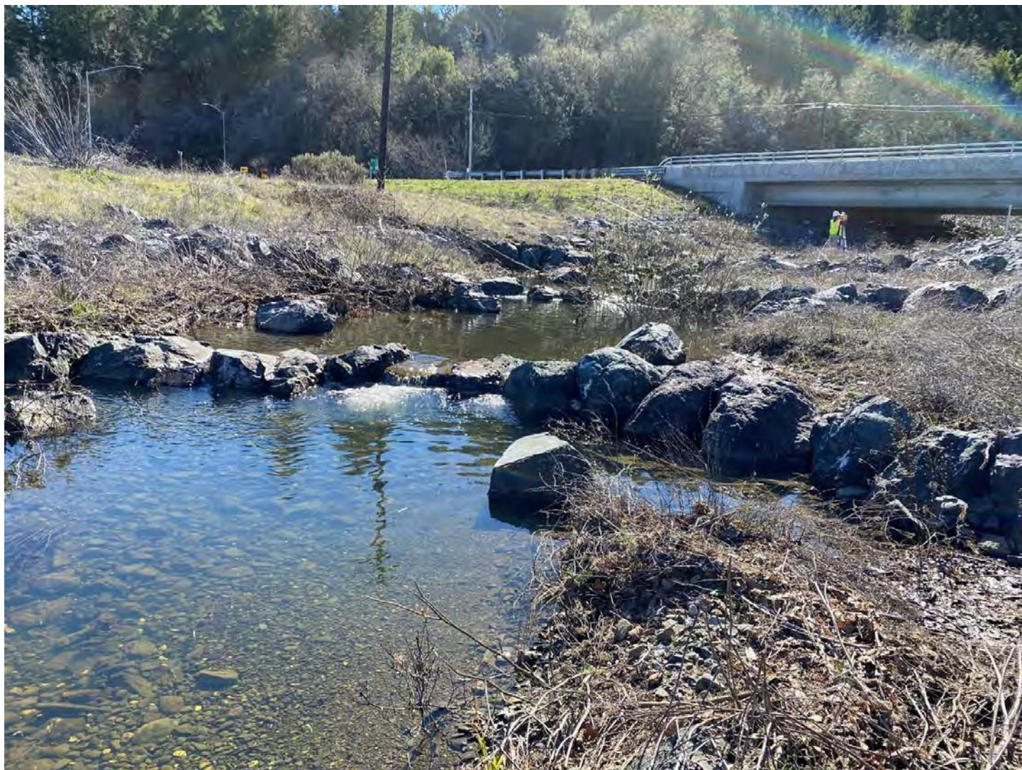
Figure 2. Intact and fully functioning rock weirs viewed from downstream looking upstream at new bridge. Photo by Michael Love on 2/24/2021.
