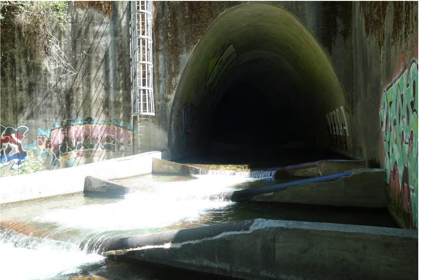
Figure 10. Cedar Creek culvert outlet weirs showing some of the crumbling concrete weir edges, especially around the installed steel plate coverings. Photo taken June 3, 2021.
