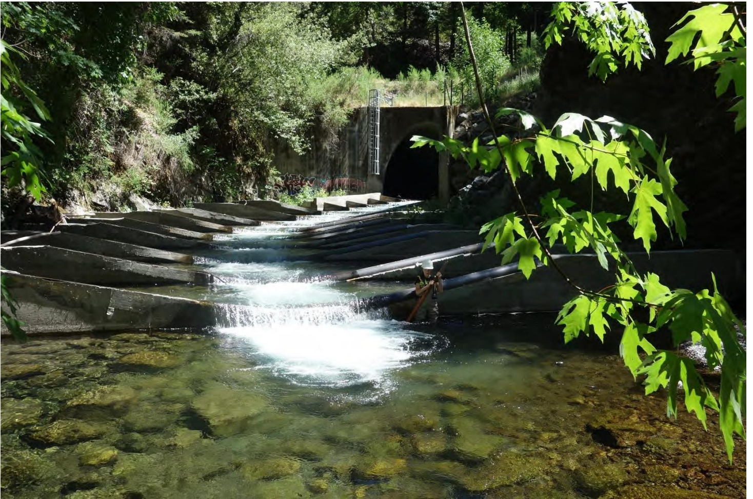
Figure 5. Cedar Creek outlet fishway looking upstream. The drop heights over the weirs under these conditions ranged from 1.25 ft (drop height at most downstream weir) to 0.4 ft; all but two drop heights were less than 0.75 ft. Photo taken June 3, 2021.
