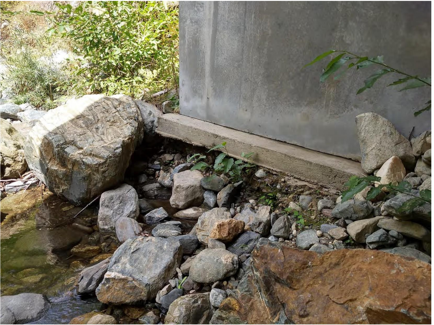
Figure 4. Close-up of upstream, left bank of bridge showing scoured bank protection and exposed footing. Photo by M. Lang on 9/19/2019.
