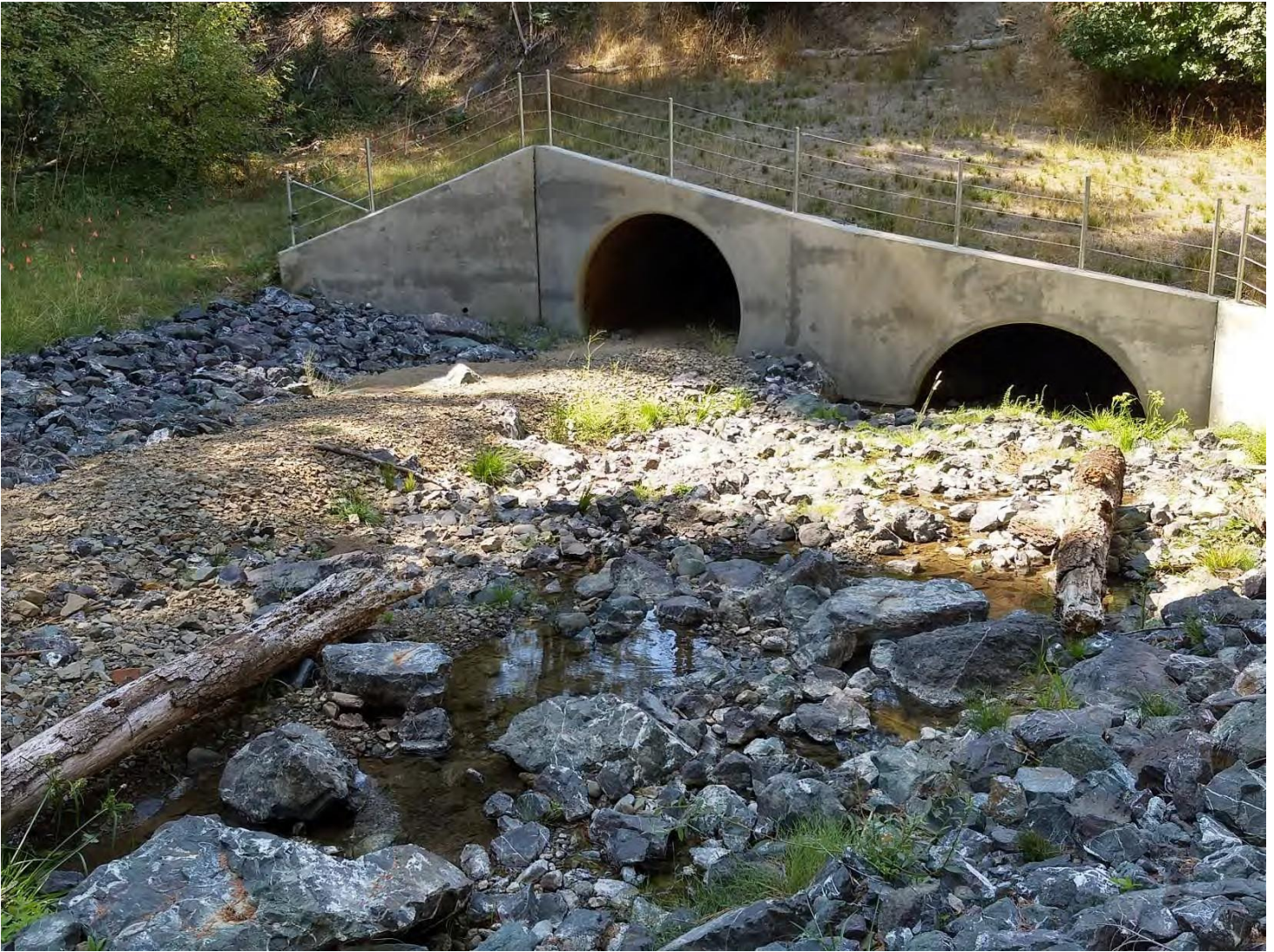
Figure 3. Close-up of the embedded inlets of the double-barrel South Fork Ryan Creek crossing. Photo by Margaret Lang on 9/12/2019.
