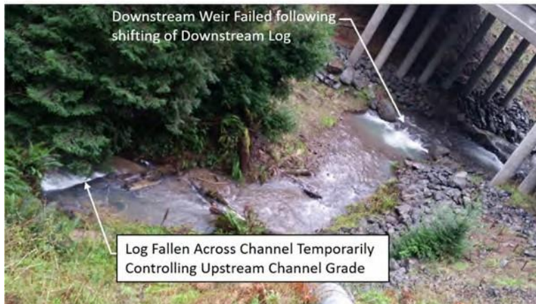
FIGURE 5-2. THE DESIGN ELEVATION AND DROP OVER THE DOWNSTREAM WEIR WAS BASED ON THE DOWNSTREAM CHANNEL BED ELEVATION CONTROLLED BY RECENTLY FALLEN LOG WITHIN THE CHANNEL BED, WHICH SUBSEQUENTLY SHIFTED, CAUSING THE BED TO DROP AND THE BOULDER WEIR TO FAIL.
