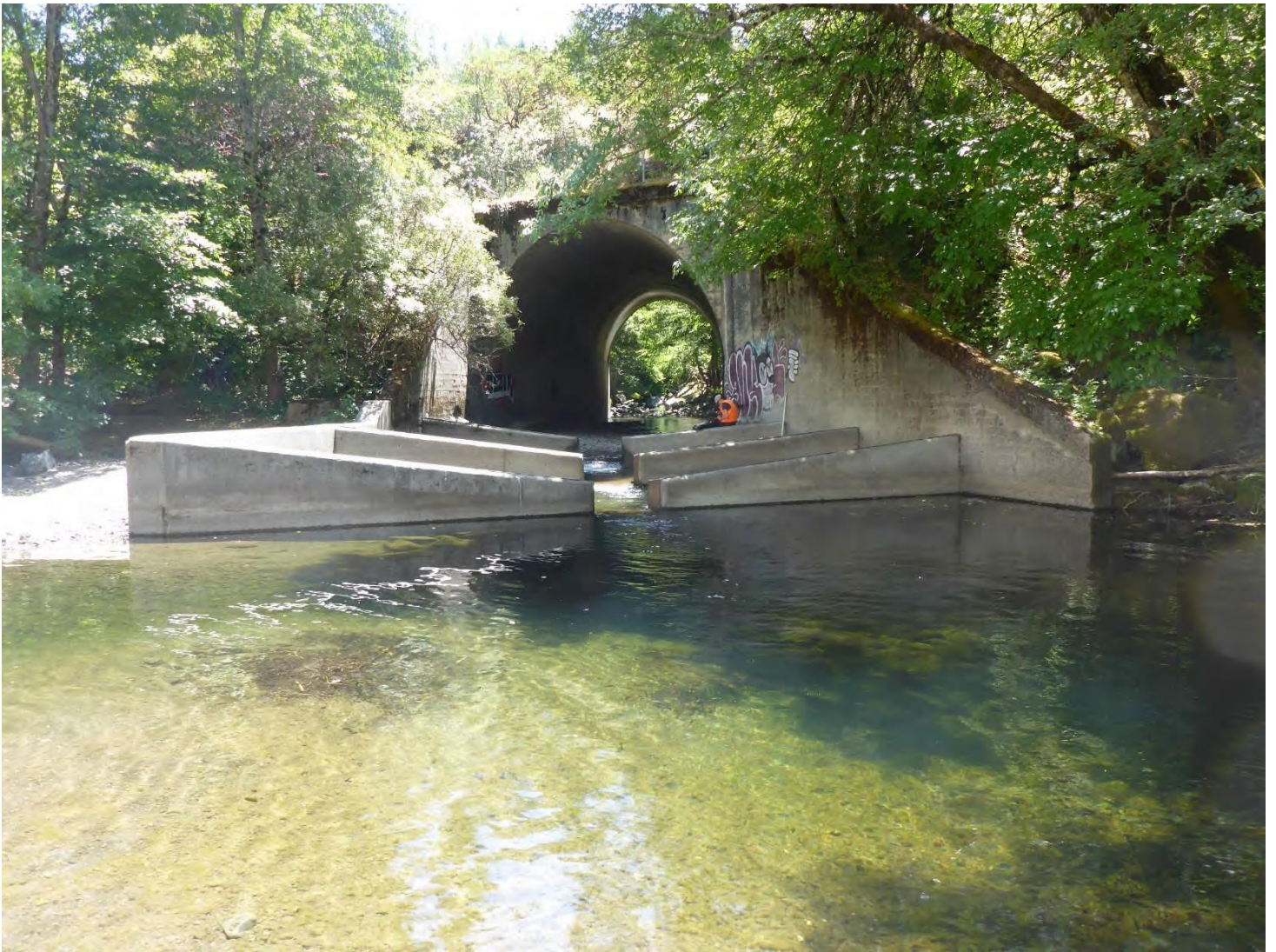
Figure 5. The outlet pool weirs looking upstream from the outlet pool tailwater control. Photo M. Love on July 17, 2019.
