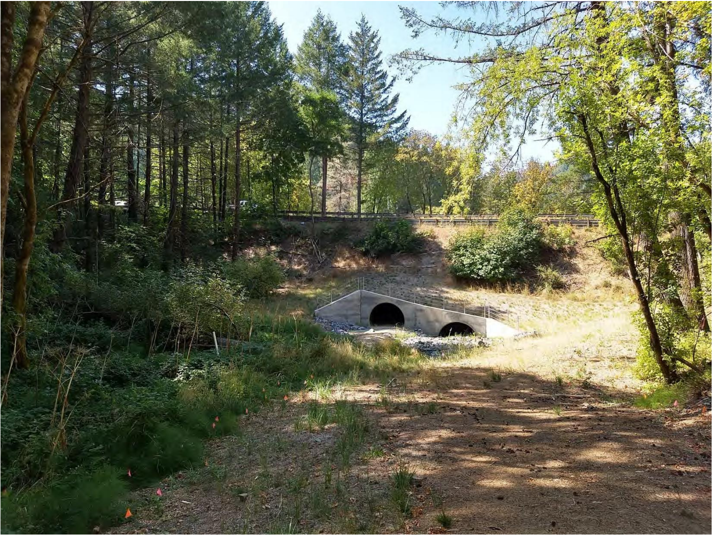
Figure 2. Embedded inlets of the double-barrel South Fork Ryan Creek crossing. Photo by Margaret Lang on 9/12/2019.
