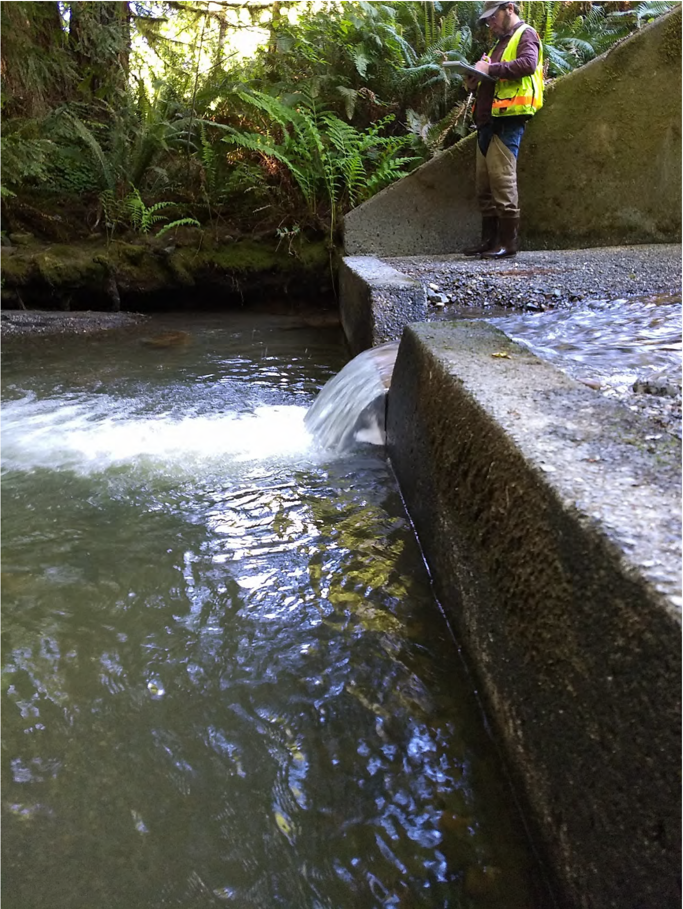
Figure 5. Concrete square-notched weir at outlet. Drop elevation is ~1 foot at low flow.
