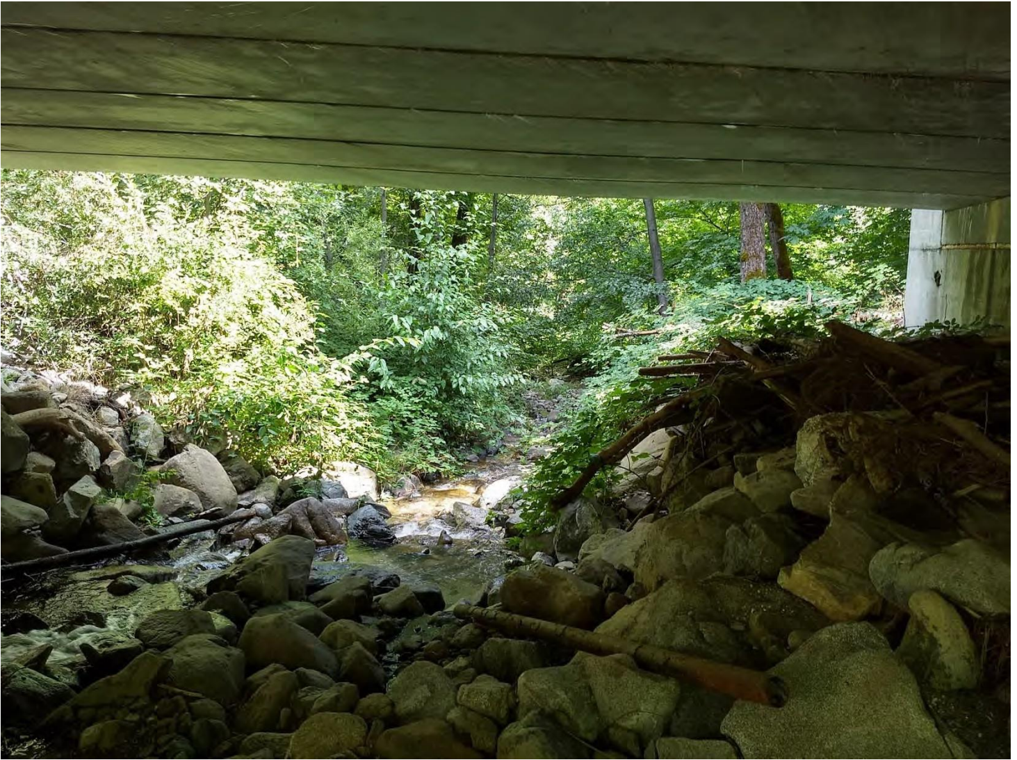
Figure 6. Channel under the bridge showing wood deposited at high flows onto the top of the constructed bank protection. Photo by M. Lang on 9/19/2019.
