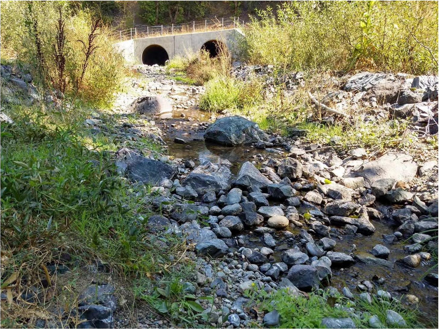
Figure 7. The culverts' outlets looking upstream from the downstream channel. The low flows resurface and become continuous again with the lower sections of the project and were continuous in the downstream channel. Photo by Margaret Lang on 9/12/2019.
