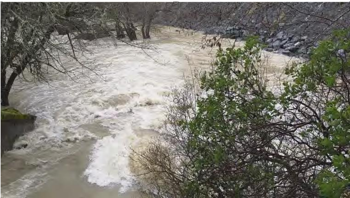
FIGURE 9-4. RATTLESNAKE CREEK OUTLET DURING HIGH FLOW. THE PRIMARY FLOW EXITING THE FISHWAY FOLLOWS THE NEW FISHWAY ORIENTATION AWAY FROM THE RIGHT BANK. AN EDDY FORMS ON THE RIGHT CREATING SOME SCOUR ALONG THE SIDE OF THE FISHWAY. PHOTO TAKEN FEBRUARY 27, 2019 BY M. LANG.
