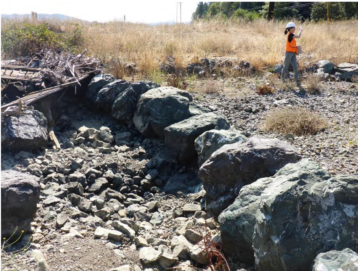
Figure 5. Scour maintained pool downstream of rock weirs. This is the same rock weir shown in Figure 2. Photo by Michael Love on 9/12/2019.
