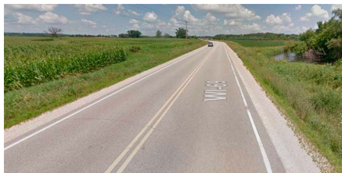
WIS 69 prior to reconstruction
