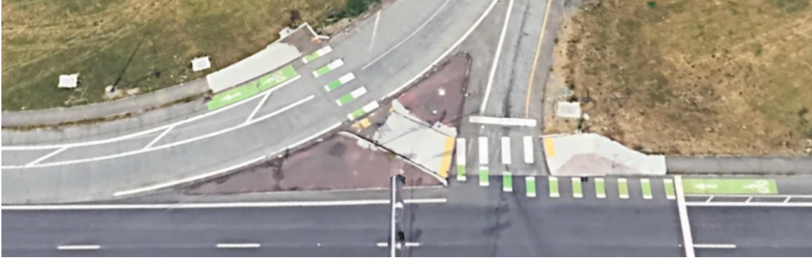
Figure 28. I-5 Exit Ramp at Mill Plain Boulevard in Vancouver, Washington [3].
