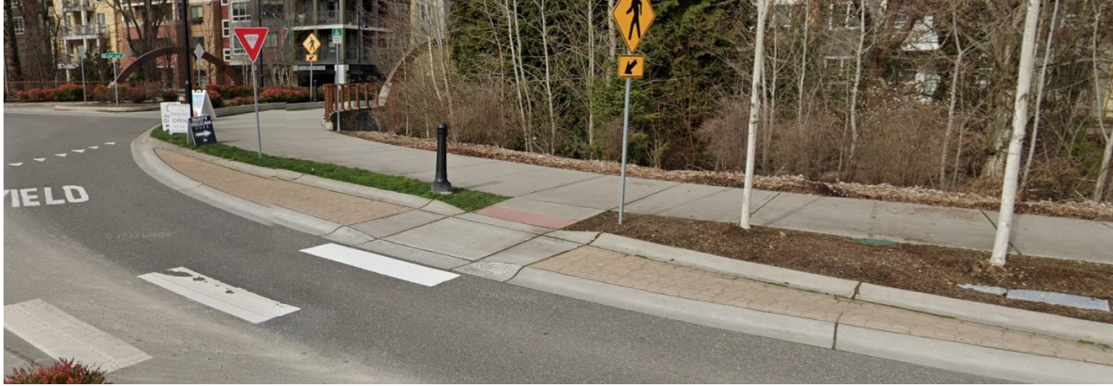
Figure 37. NE 171st Street and 135th Avenue in Woodinville, Washington [3].
