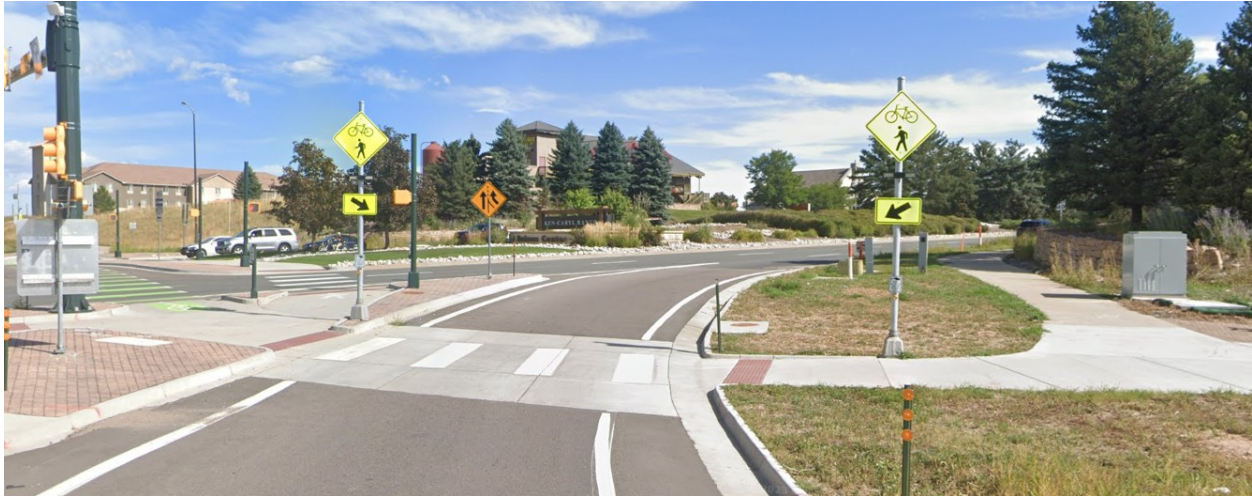
Figure 22. CO-470 Exit Ramp to W Ken Caryl Avenue in Littleton, Colorado [3].
