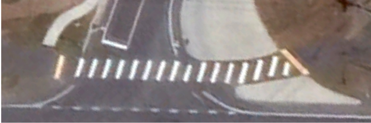
Figure 35. Peace Portal Drive and Hughes Avenue in Blaine, Washington [3].
