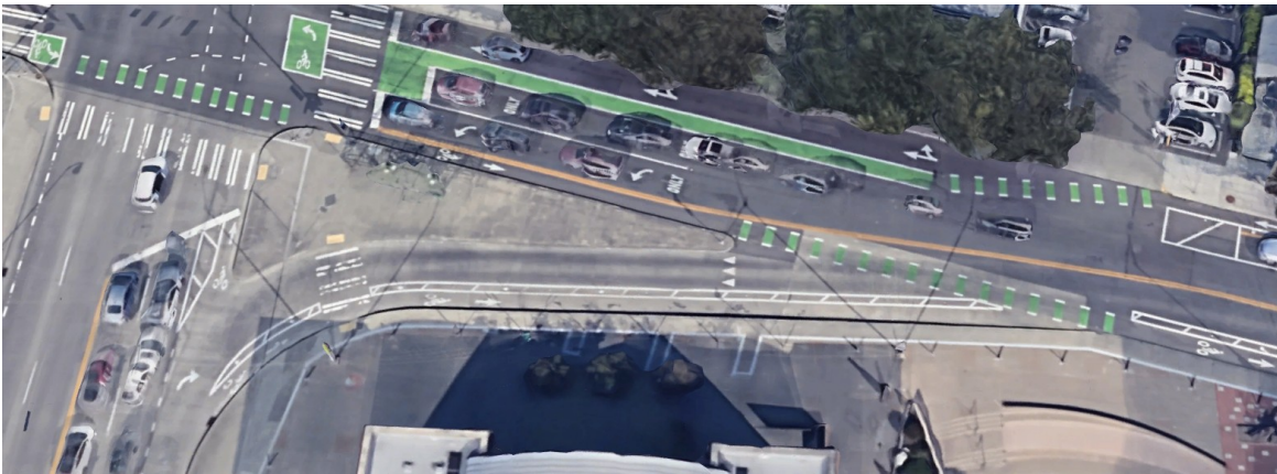
Figure 29. Fremont Avenue at 34th Street in Seattle, Washington [3].
