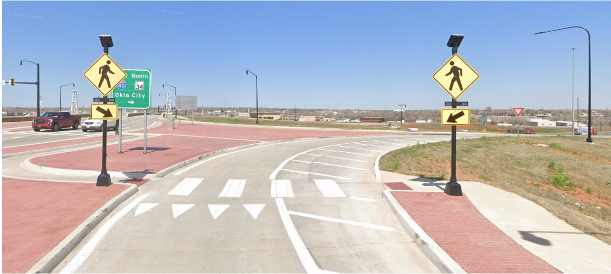
Figure 24. I-20 Exit Ramp at Main Street in Elk City, Oklahoma [3].
