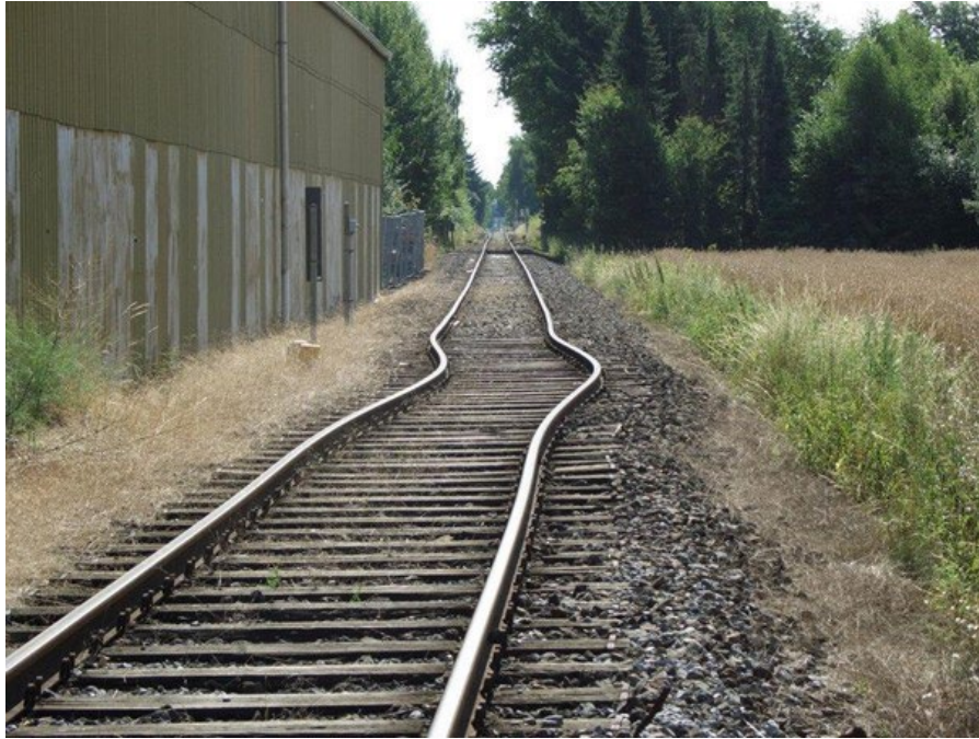
Figure 1: Photograph showing thermally induced buckling of a railway (reprinted with permission from ABproTWE, CC BY-SA 3.0, via Wikimedia Commons)
