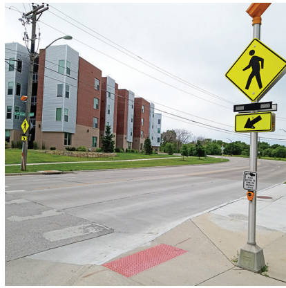
Rectangular rapid flashing beacon under a pedestrian warning sign
